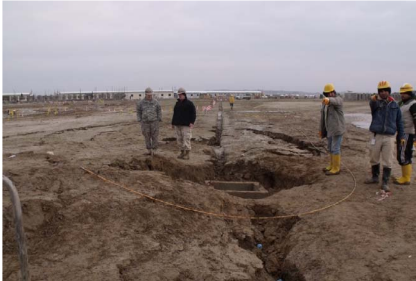
Photo 6: Roadbed Showing Settling at Kunduz ANA Garrison
