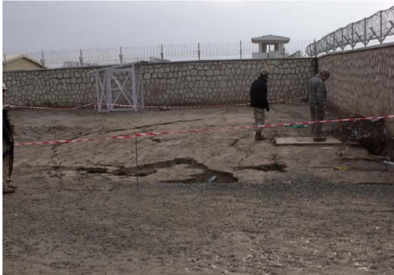
Photo 5: Settling along the Embedded Training Team Compound Wall at Kunduz ANA Garrison
