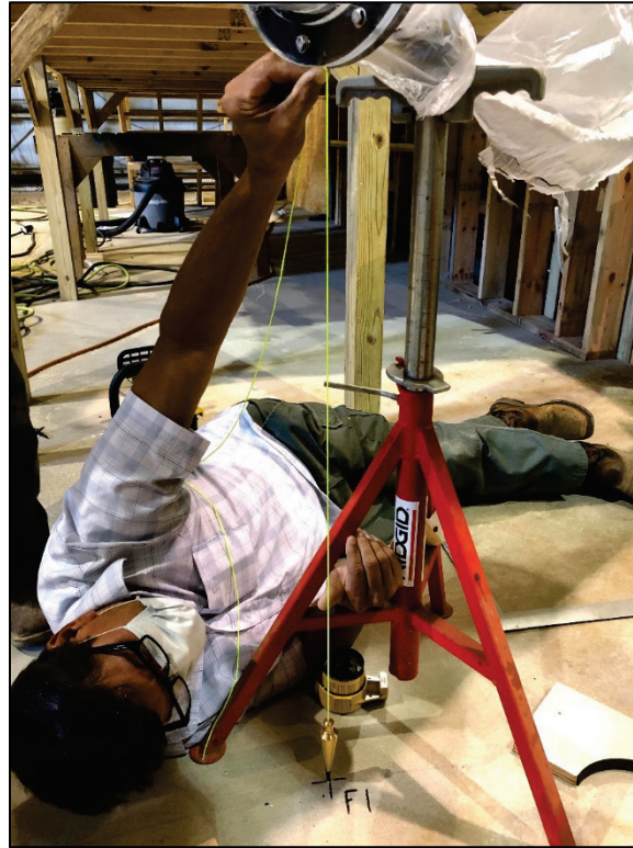
Figure 8. Alignment of conduit with control points.
