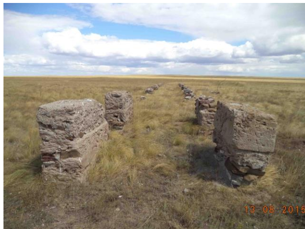
Figure 76. Concrete piers at the control site for the Meridian-1 PNE.
