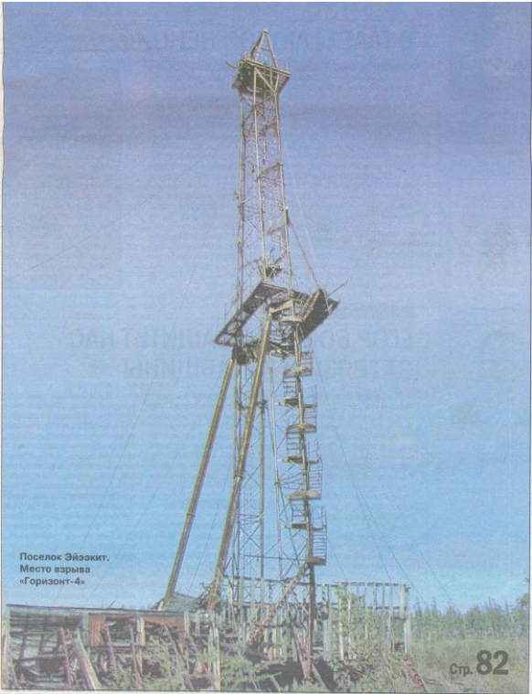
Figure 95. The emplacement tower for the Horizon-4 PNE.
