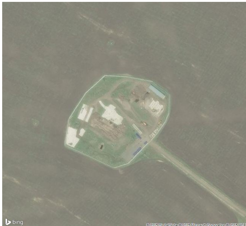
Figure 21. Bing Maps image of the Magistral' location. This is a more recent image and it shows that the site is under development. Note an installed perimeter fence, concrete pads, possible building foundations, material storage, and a line of utility poles just south of the access road. The utility poles trace back to the oil field development to the east.
