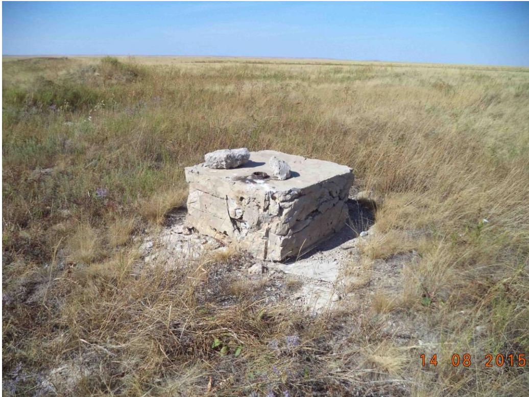
Figure 65. The capped borehole of Region-5
