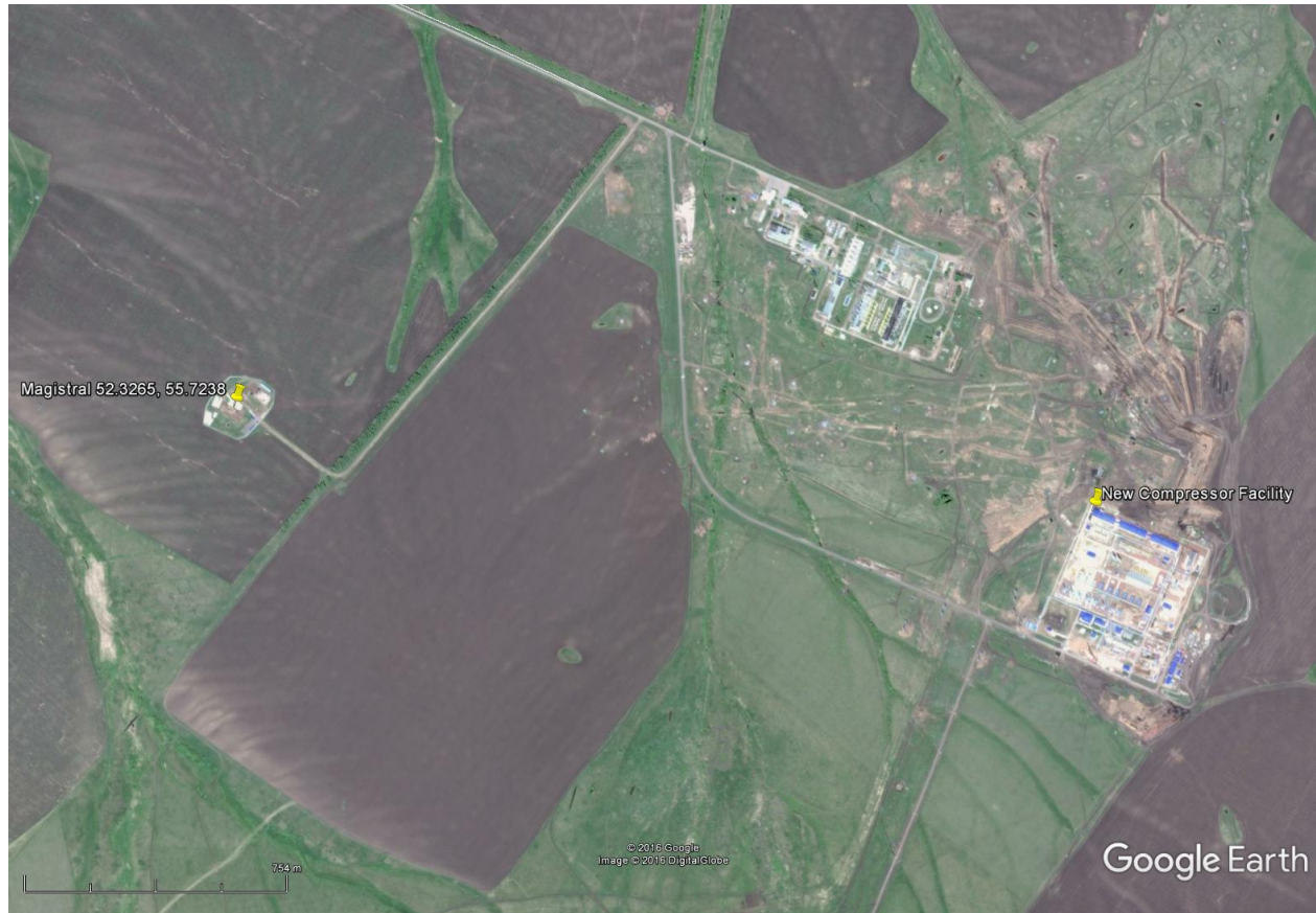
Figure 24. Overview of the Magistral’ site showing the PNE location at left, and the new gas compressor station at right. The older original “gazopromysel Sovkhoznyi” facility. Google Earth Image © 2016 Digital Globe.
