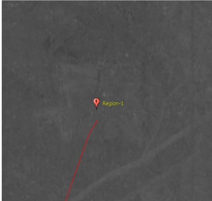
Figure 57. Geoportal Roskozmos image of the Region-1 site showing an overgrown square structure at the site. The square is approximately 150 m per side. A small white spot near the center would be consistent with the concrete plugged borehole. The red line indicates the future location of the connecting pipeline.
