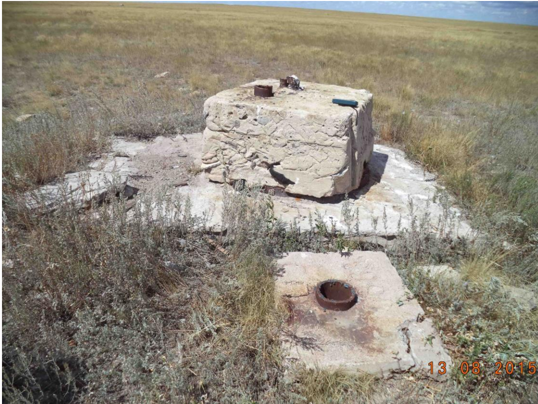
Figure 72. Capped borehole for the Meridian-1 PNE. The steel casing of the borehole is visible at the base of the concrete block. The smaller concrete pad and small borehole casing is highlighted in the next figure below.
