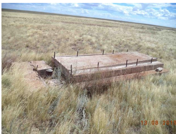
Figure 74. A. One of two concrete mounting pads in line with the main borehole and presumably used for a support tower. B. Instrument borehole casing. C. Concrete mounting pad of unknown use with an apparent borehole at one end.
