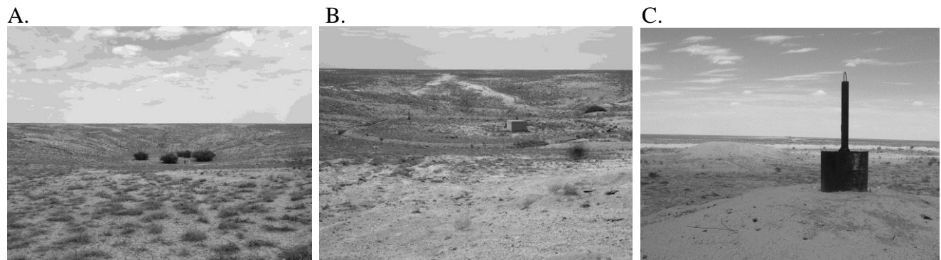
Figure 19. A. Collapse crater from Man-1. B. Collapse crater and infrastructure at the Man-2 site. C. Borehole locations for Man-3.
