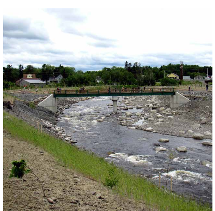
Top: Pools, riffles, bars, and boulders designed for stability during major flood events. (Photo by Inter-Fluve)
