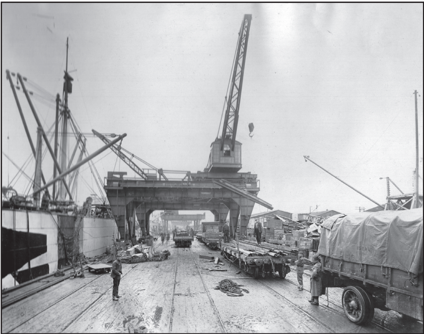
Figure 3.2 Once installed, the gantry cranes at the American-constructed port in Bassens significantly increased the efficiency of the cargo operations. Photo courtesy of the US Army Quartermaster Museum.
