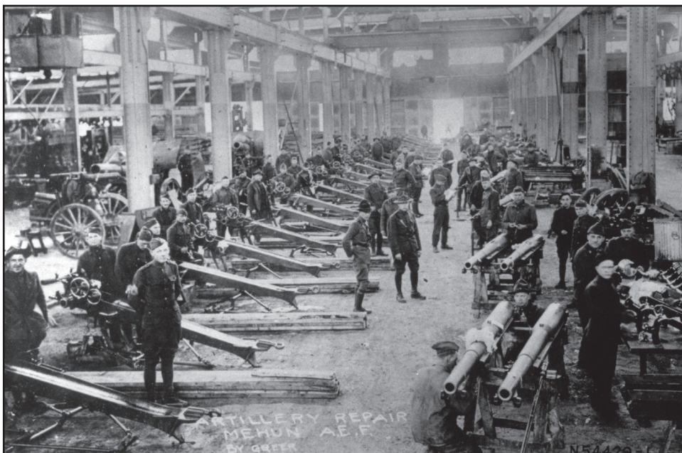
Figure 5.3 Artillery repair shop as part of the massive ordnance facility at Mehun. Photo courtesy of the US Army Ordnance School Historian.
