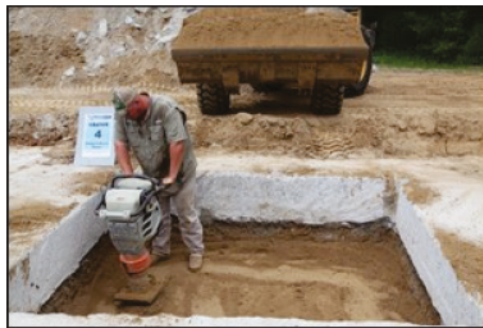
(c) Compacting CL-ML lift with jumping jack.
