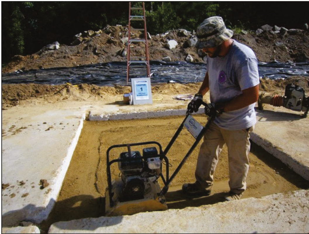
Figure 3.14. Final surface preparation with plate compactor.
