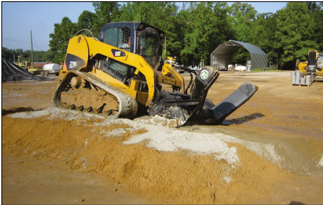
Figure 3.10. CTL tiller attachment (Caterpillar LT13B) used to blend soil with additive.
