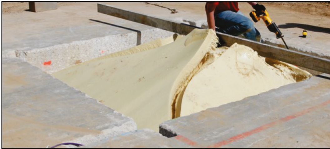
Figure 3.26. Final foam backfill surface of Repair 8 (after cutting).
