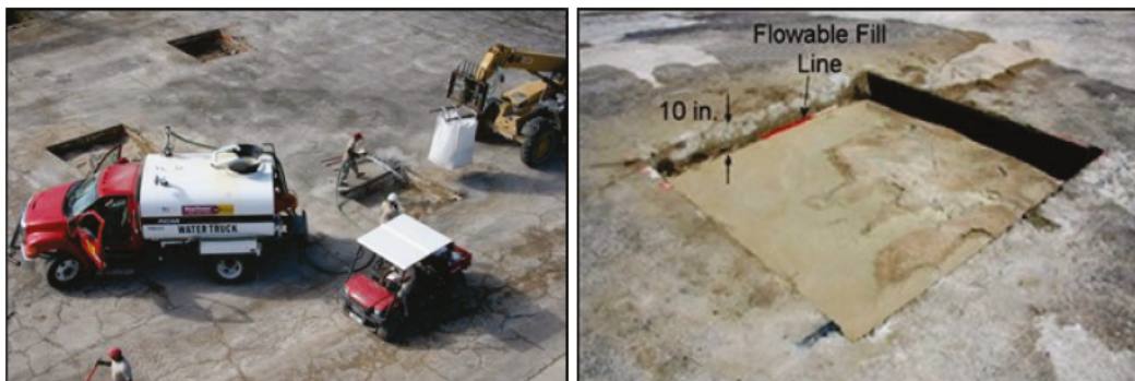
Figure 1.1. RADR backfill method of flowable fill capped with rapid-setting concrete.
