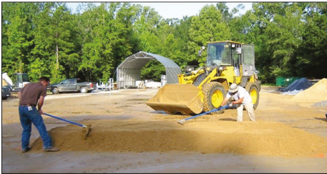
Figure 3.9. Addition of PLC.
