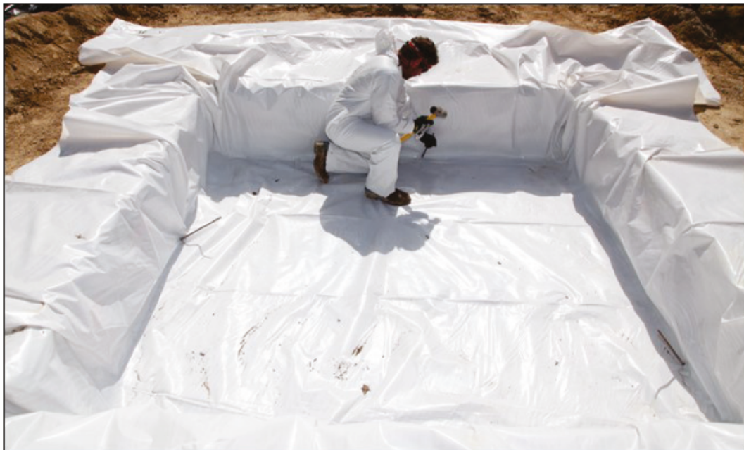
Figure 3.21. Polyethylene liner applied to Repair 4.
