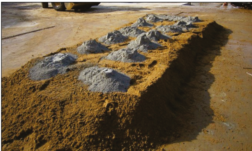
Figure 3.9. Addition of PLC.
