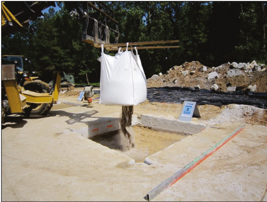
Figure 3.16. Adding water to rapid-setting flowable fill during dry placement method.
