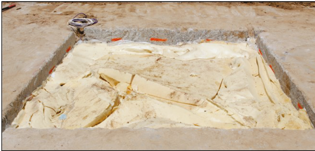
Figure 3.24. Final foam backfill surface of Repair 4.
