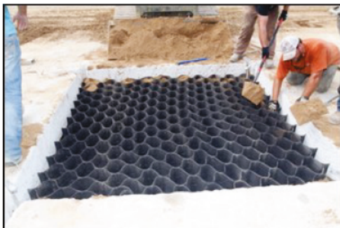
(c) Placing SM along edges (Repair 7).
