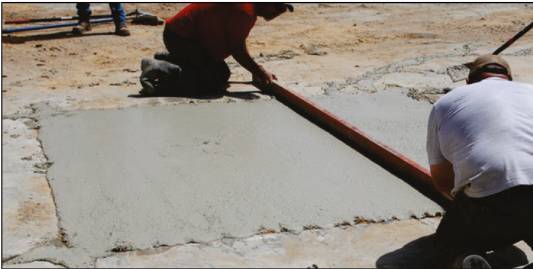
Figure 3.31. Finished rapid-setting concrete cap on Repair 1.
