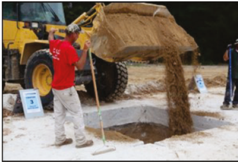
(a) Placing CL-ML lift into crater.
