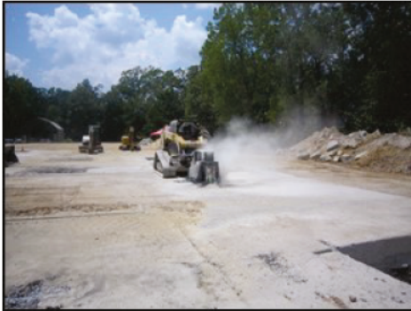
(a) Cutting PCC with wheel saw.
