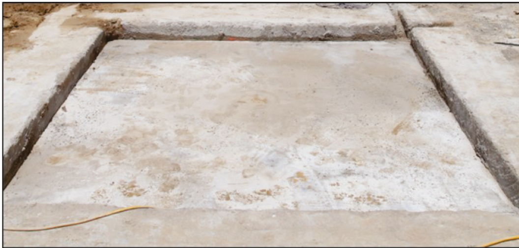
Figure 3.17. Finished rapid-setting flowable fill surface.
