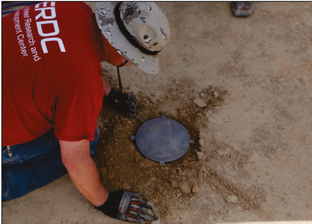
Figure 3.7. EPC being installed at the center of a repair over the constructed subgrade.
