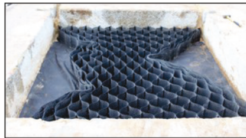
(b) Geocell section placed in crater
