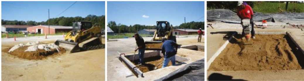
Figure 1.4. Chemically stabilized soil backfill method.
