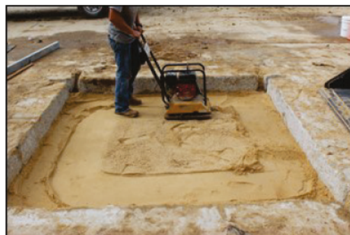
(f) Compacting SP with plate compactor (Repair 3).
