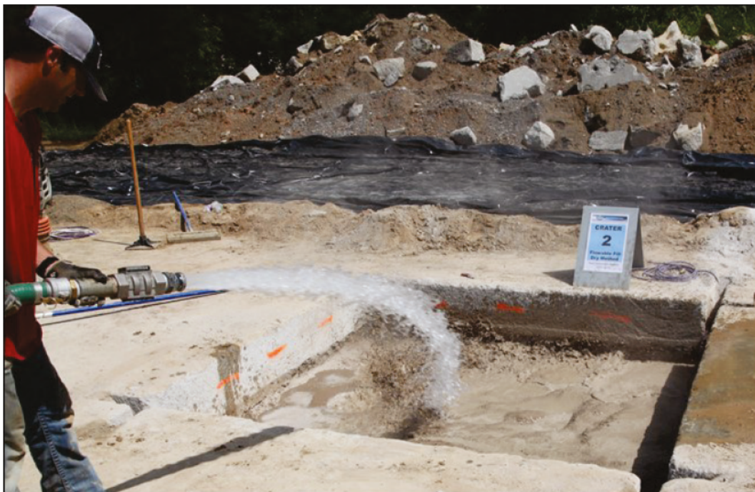
Figure 3.16. Adding water to rapid-setting flowable fill during dry placement method.
