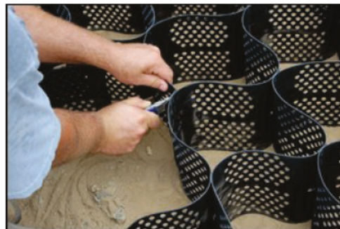
(b) Cutting geocell section with utility knife.
