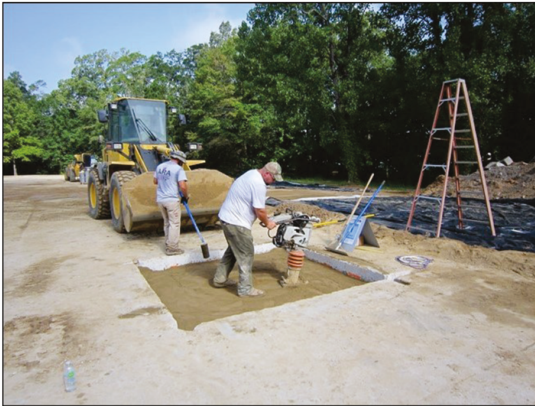
Figure 3.13. Compacting soil.
