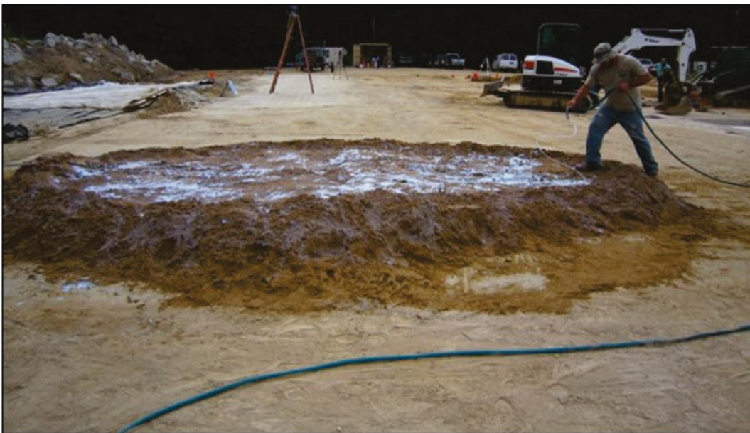
Figure 3.12. Spraying polymer emulsion on loose soil.
