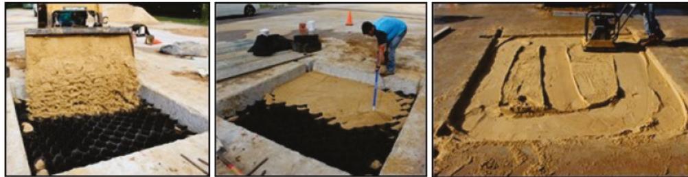
Figure 1.3. Geocell mechanical stabilization method.
