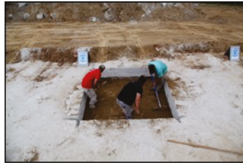
(b) Leveling CL-ML lift.
