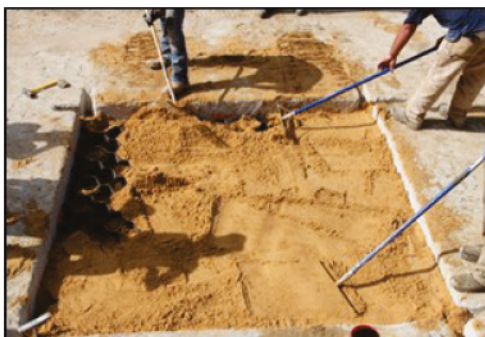
(e) Spreading SP evenly with rakes (Repair 3).
