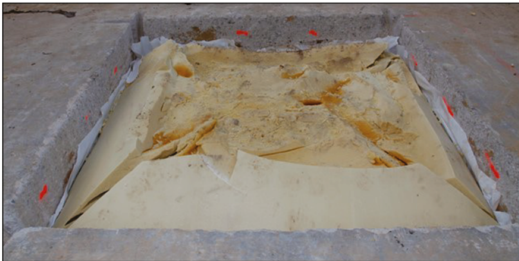
Figure 3.26. Final foam backfill surface of Repair 8 (after cutting).
