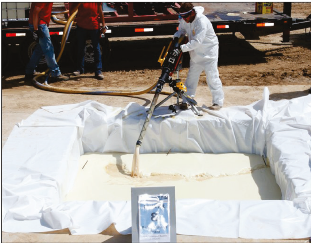
Figure 3.23. Placing additional foam in Repair 4 to achieve the desired backfill thickness.
