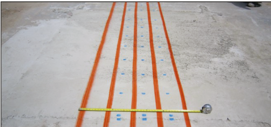
Figure 3.38. Finished rapid-setting concrete cap on Repair 8.
