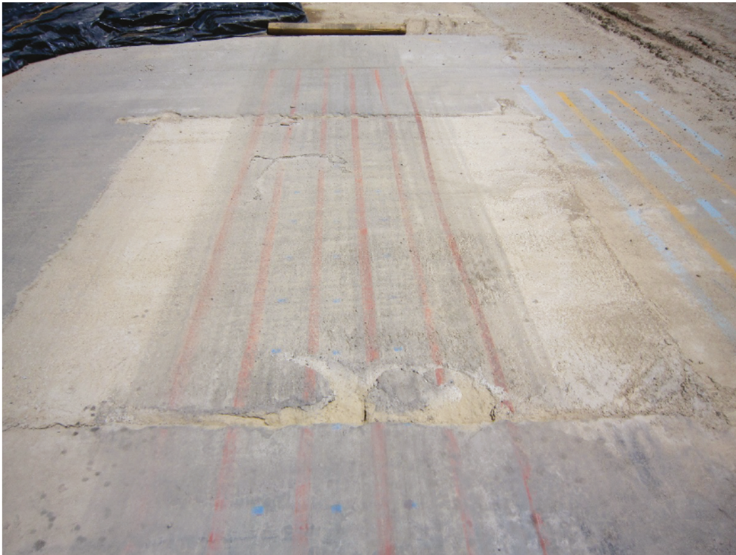
Figure 4.11. Shrinkage cracks on Repair 4.
