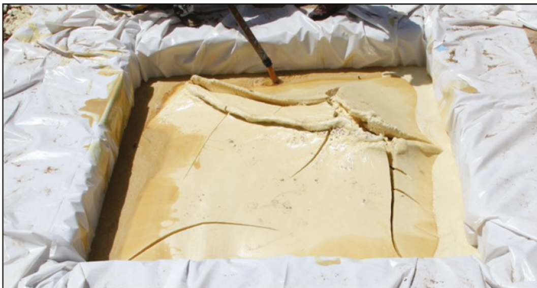
Figure 3.23. Placing additional foam in Repair 4 to achieve the desired backfill thickness.
