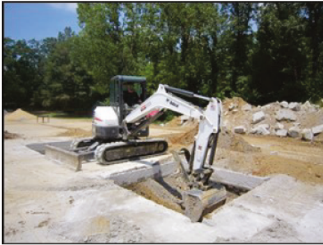
(c) Excavating to proper depth.
