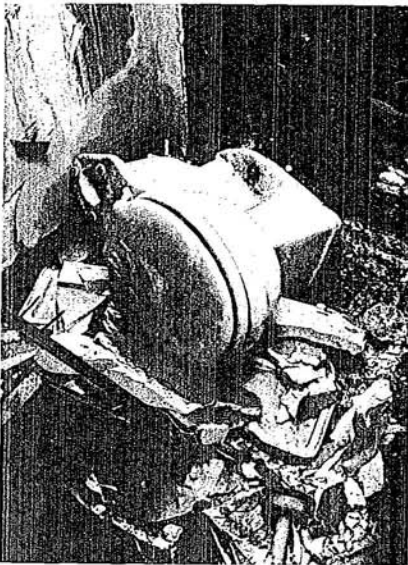
Vandalized bathroom severely damaged and stripped of fixtures.
