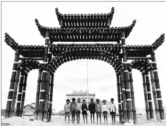
Photo by Maj Barry Broman, USMCR (Ret) The gate to a Buddhist temple in An Hoa constructed out of used Marine Corps artillery containers, showing local children happy to pose and some of the civic action work done by Marines at An Hoa in 1969.
