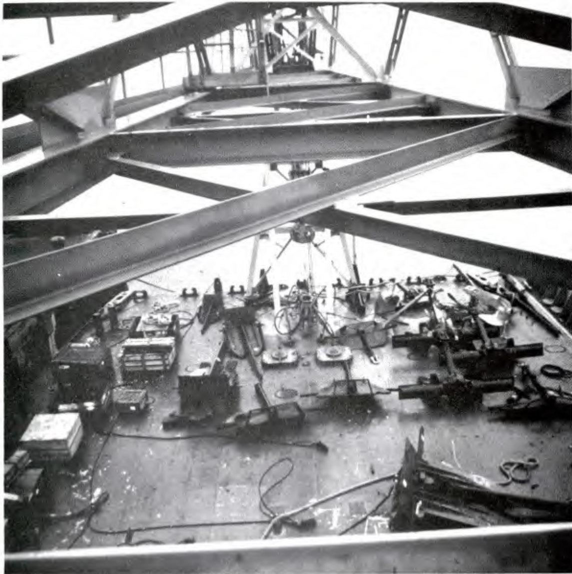
Figure 8. Barge crane with all test anchors.
