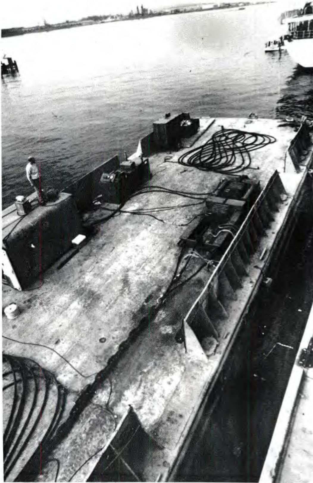
Figure 25. Test deck layout showing cable pulling system and prerigged test wire.
