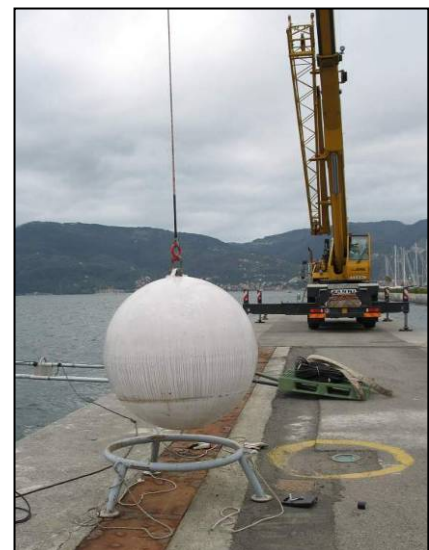
A crane was used to precisely position a target to study the signatures recorded by an underwater intruder detection sonar.
