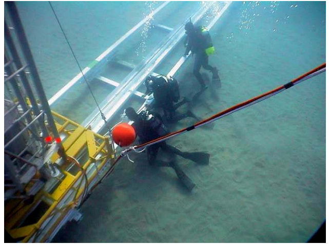
Divers working on the assembly of the rail and tower during EVA '06.
