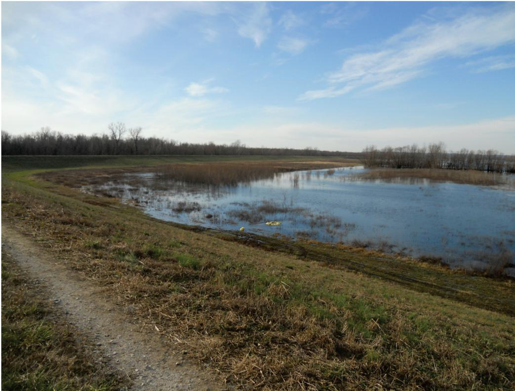
Figure 79. Two moderate-sized bagged sand boils (number 163 and 164) visible in the seepage lake (swale filled with seepage). View is in vicinity of study area 2 corresponding to location of sand boil 1 in Figure 18, which is visible in center of image.
