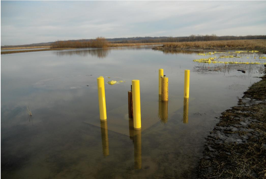
Figure 77. Extent of sand boil range near edge of the seepage berm constructed following 1993 Flood (right edge of photo).
