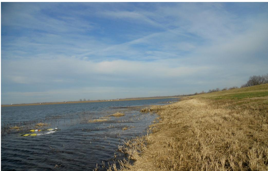
Figure 80. Shallow slide (location 168) developing on the landside slope. Slide incorporates the crown and toe of the levee at the northeast corner of the island. Note the seepage that has collected and the wet area at the toe. Probable levee through seepage occurring at this location. Several slides are present in this reach with very plastic soils used to build this section of the ring levee contributing to slide conditions.
