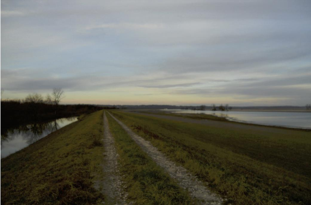
Figure 71. View looking due west from base of berm in vicinity of boil No. 151. Several sacked sand boils visible in background. Note the dry brown foam crust present on the surface of the sand boil.
