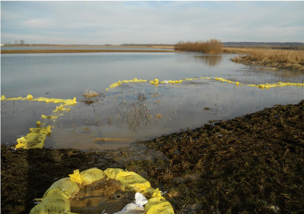
Figure 78. Small bagged boil (number 160) near turn in levee.
