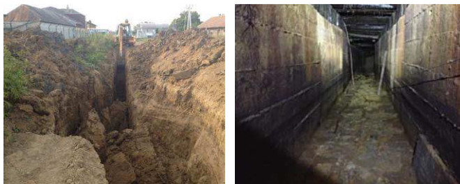
Figure 2: Photographs of soil (left) and concrete lined tunnel (right).
