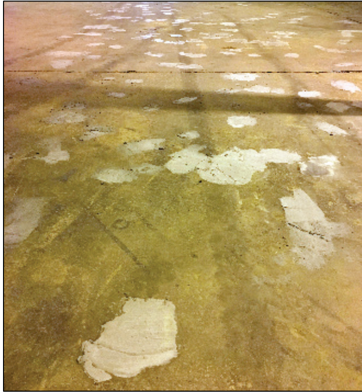
Figure 5. Divots filled with concrete and mounds removed.
