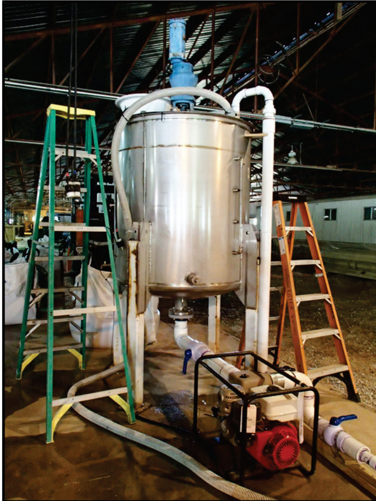
Figure 3. Sediment mixing tank.
