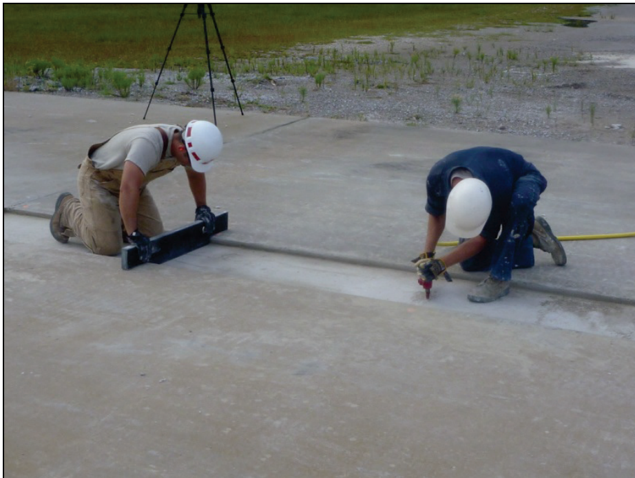
Figure C-23. Final leveling of the panel slot.
