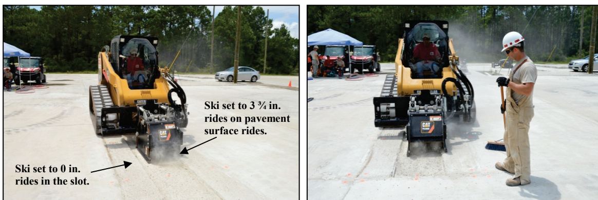
Figure E-12. Milling the panel slot.
