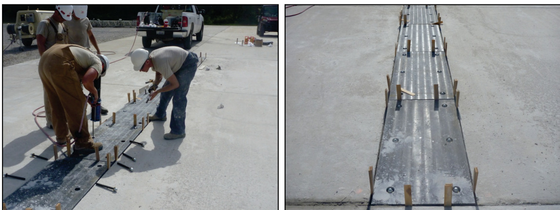
Figure E-24. Anchor installation.
