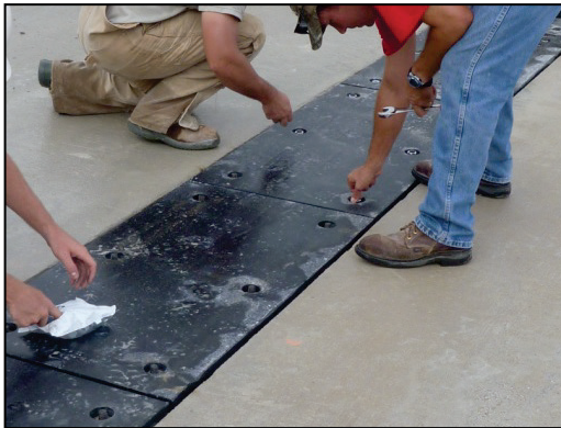
Removing temporary setting.
