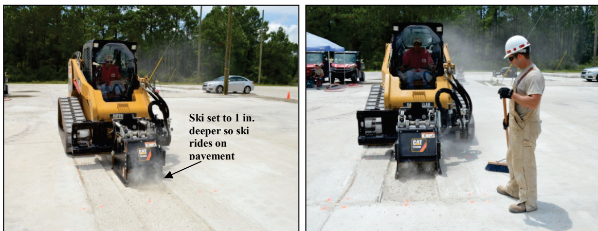
Figure B-27. Milling the panel slot.
