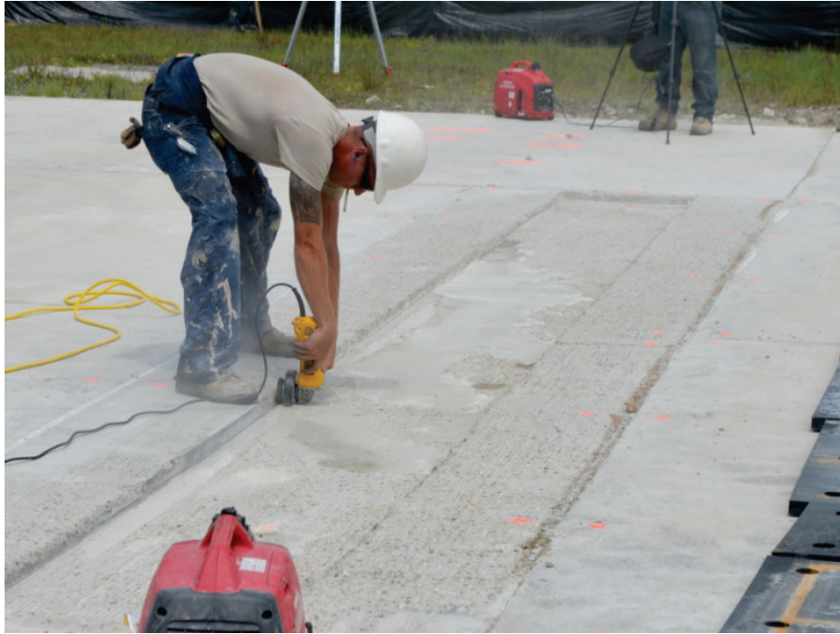
Figure C-22. Cleaning slot perimeter.
