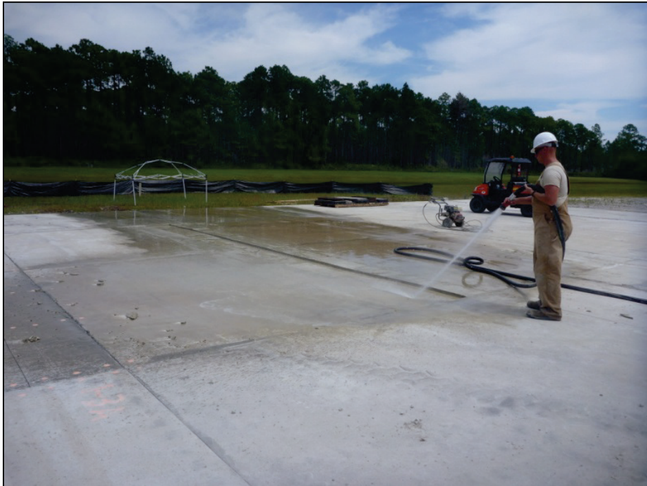
Figure A-4. Lightly rinsing the surface while sawing.
