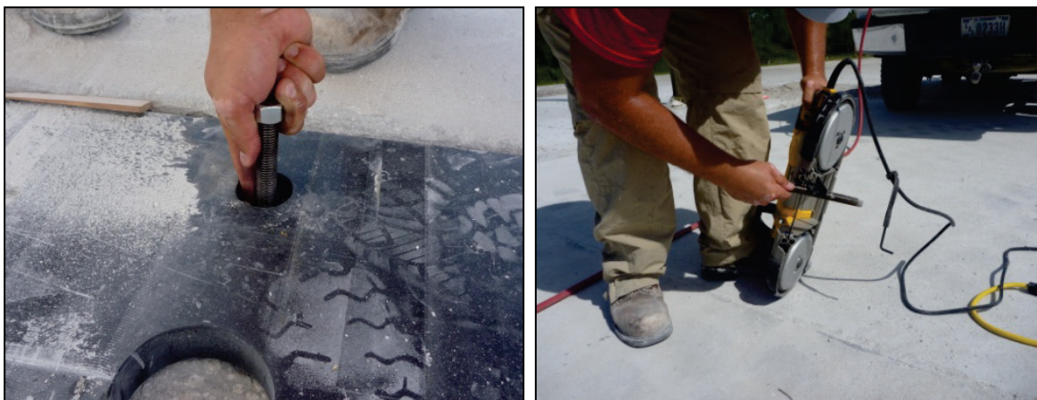
Figure E-40. Trimming a panel anchor.
