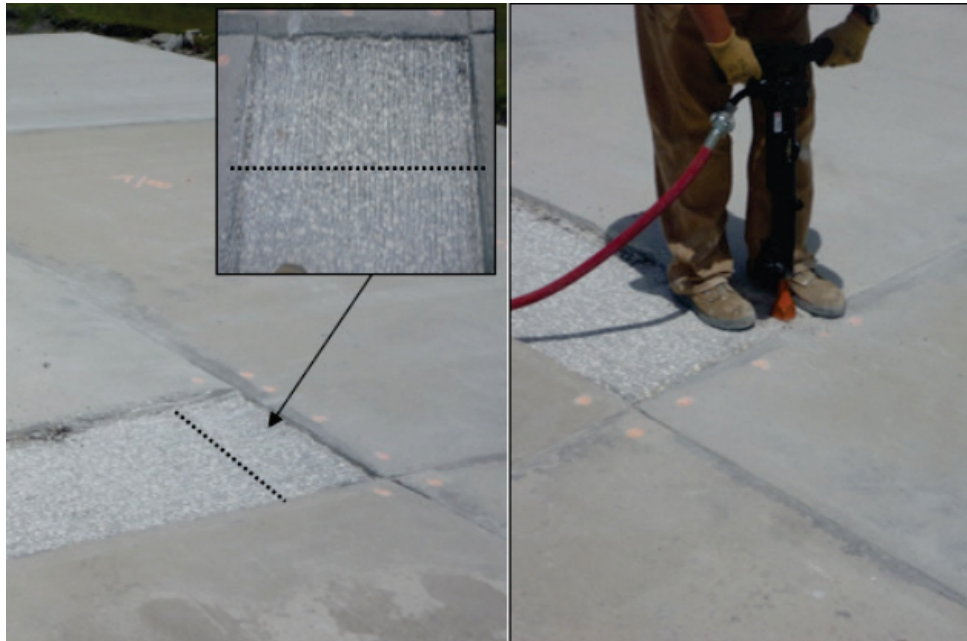
Figure 28. Un-millable portion of panel slot.
