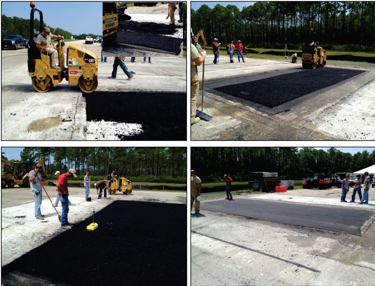
Figure D-17. Compacting asphalt patch.
