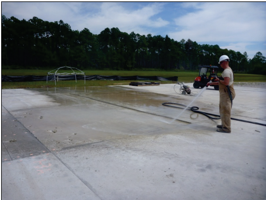
Figure C-3. Lightly rinsing the surface while sawing.
