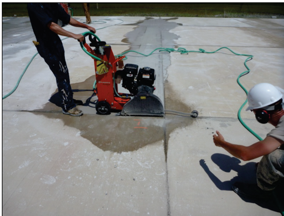
Figure E-9. Performing longitudinal cuts.
