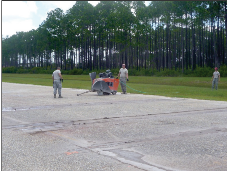
Figure B-3. Making transverse cuts.
