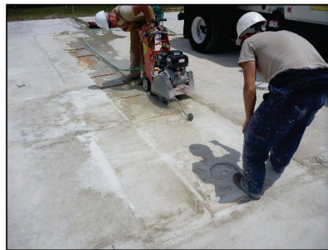
Saw needed to free formwork
