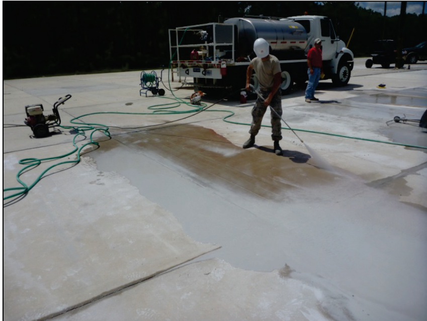
Figure A-5. Waterblasting saw slurry.
