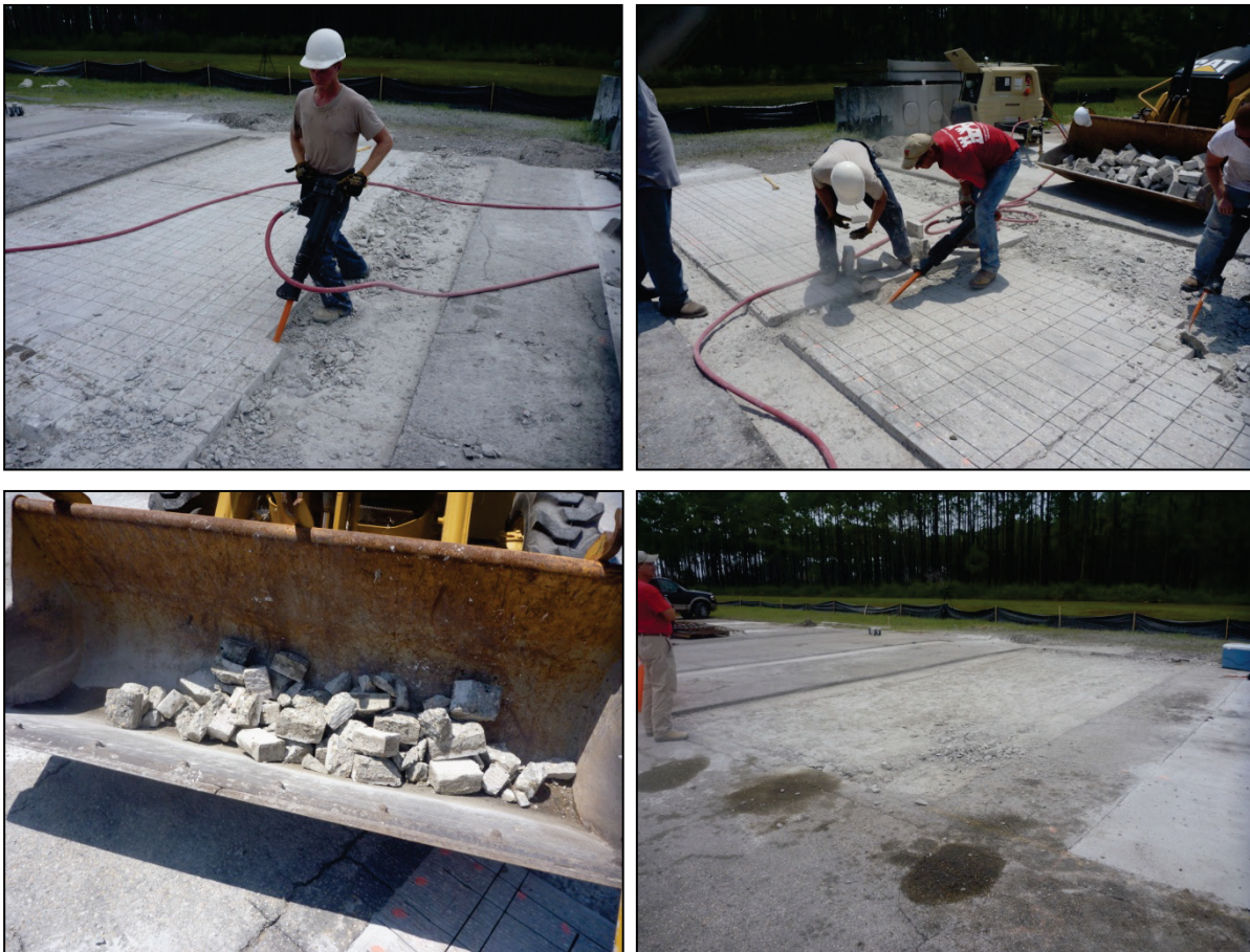
Figure C-9. Concrete foundation surface removal.
