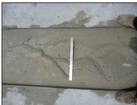
Air pockets present after removal
