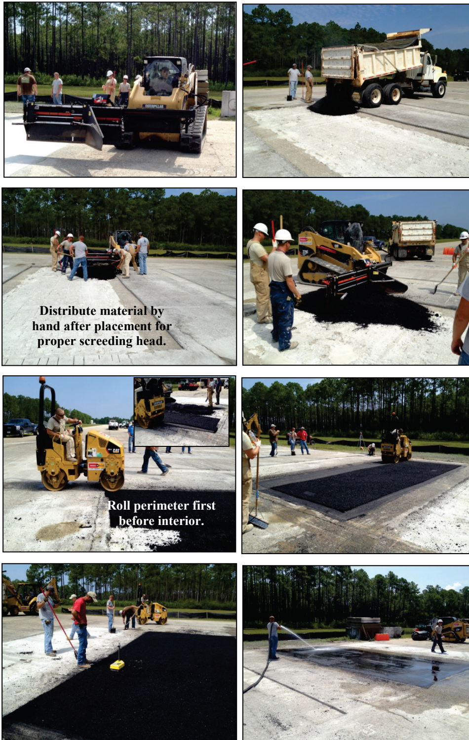
Figure B-28. Asphalt placement.
