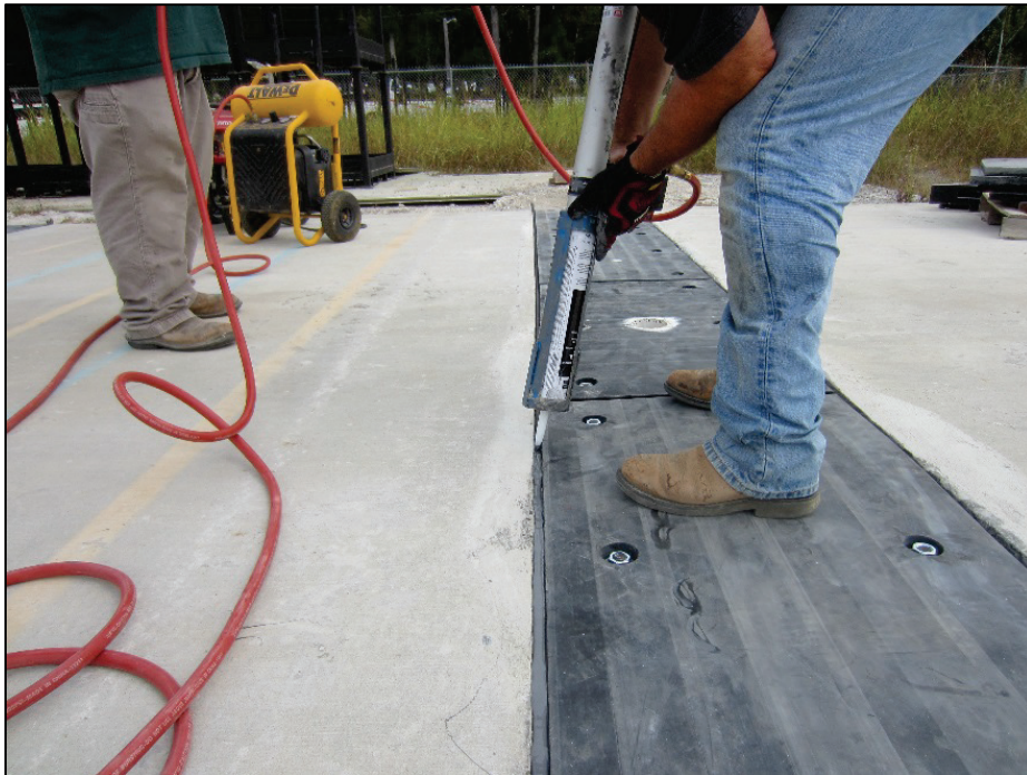
Figure C-32. Joint sealant installation.
