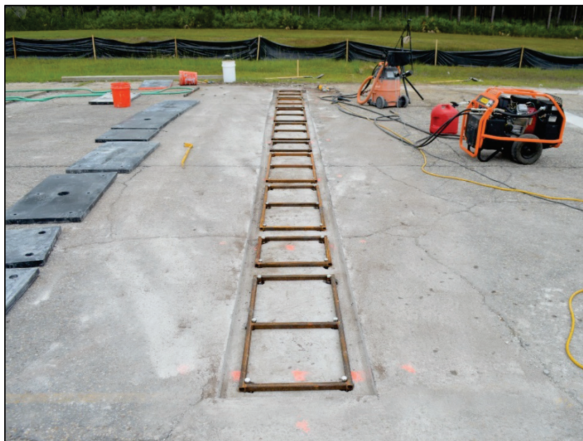
Figure 37. Tri-talon installation formwork.
