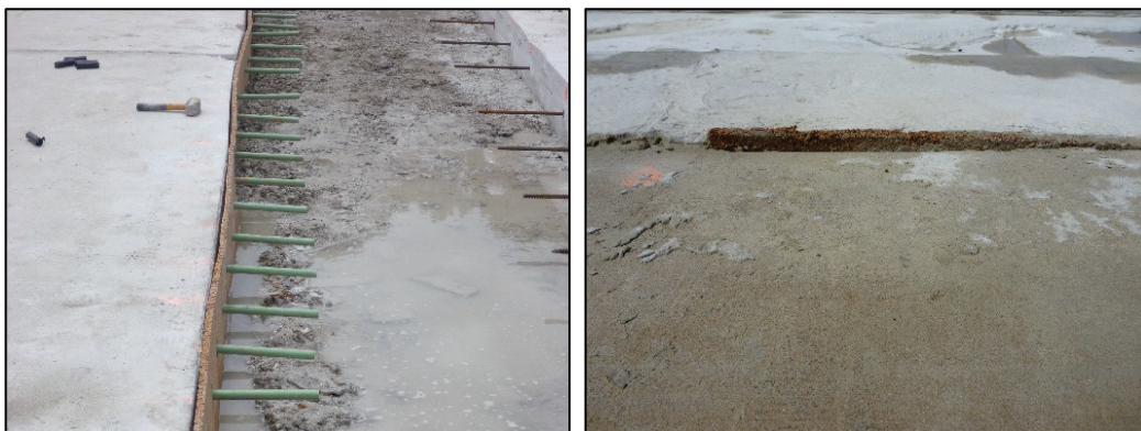
Figure 22. Poor installation of compressible insert.
