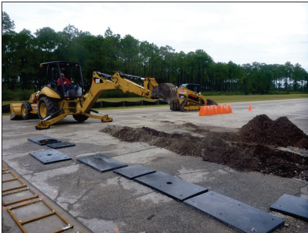
Figure B-6. Pavement surface removal.
