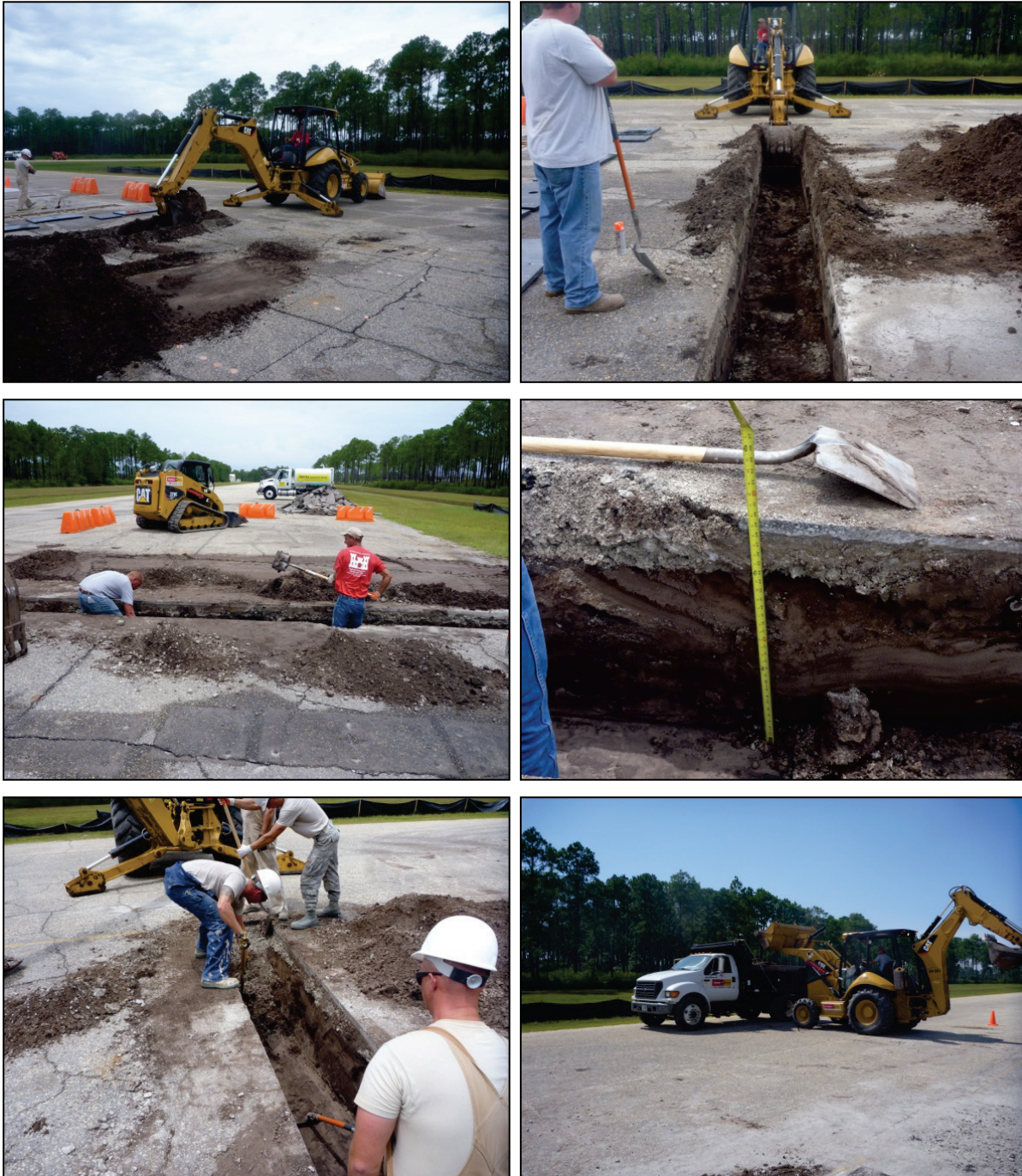
Figure E-30. Sublayer material removal.
