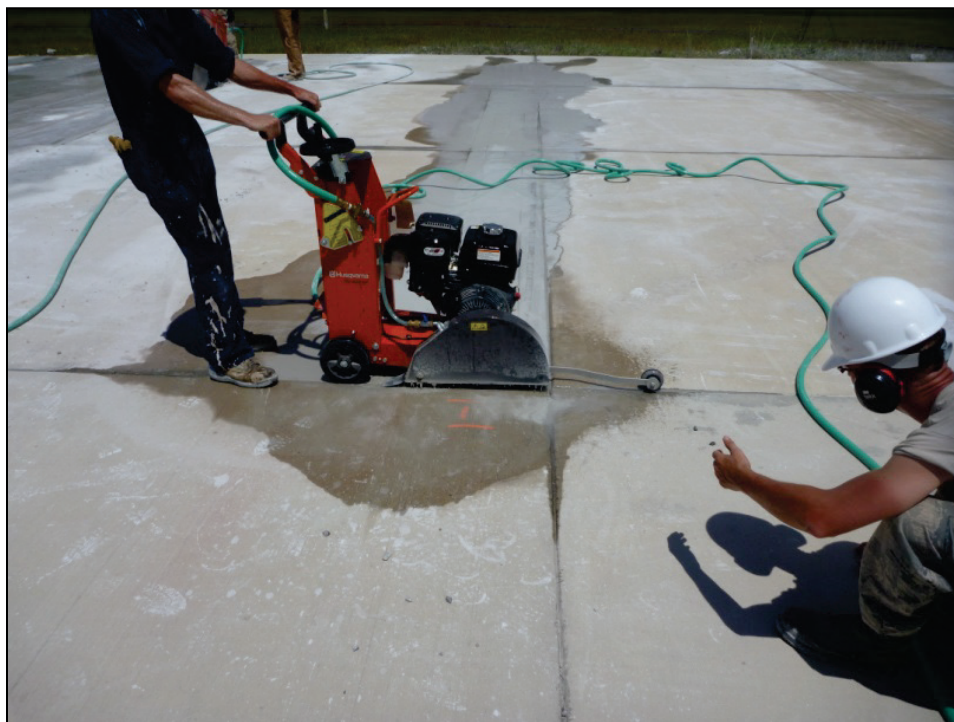
Figure D-11. Making longitudinal cuts.
