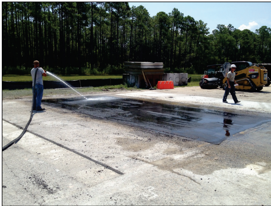
Figure C-13. Watershocking freshly compacted asphalt pavement by hand.
