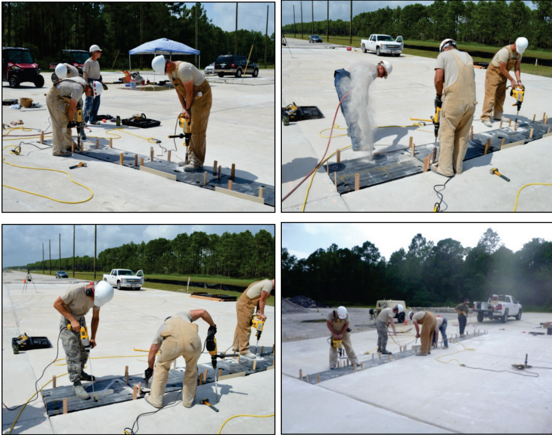
Figure E-39. Layout anchors.
