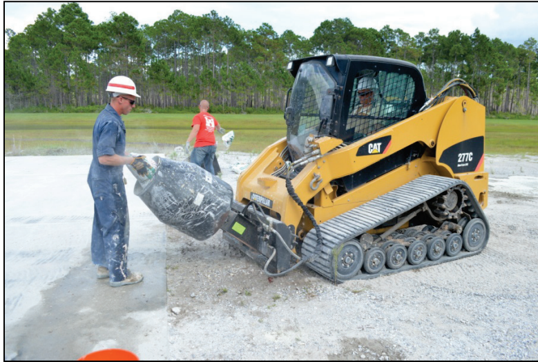
Figure C-18. Batching concrete with CTL.
