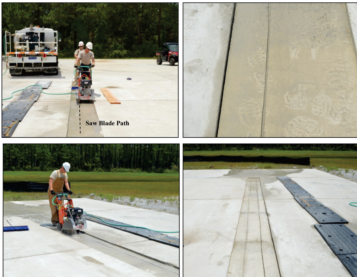
Figure C-24. Cutting drain slots.
