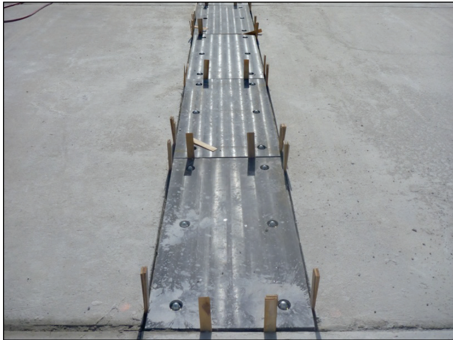
Figure B-22. After all anchors are installed.
