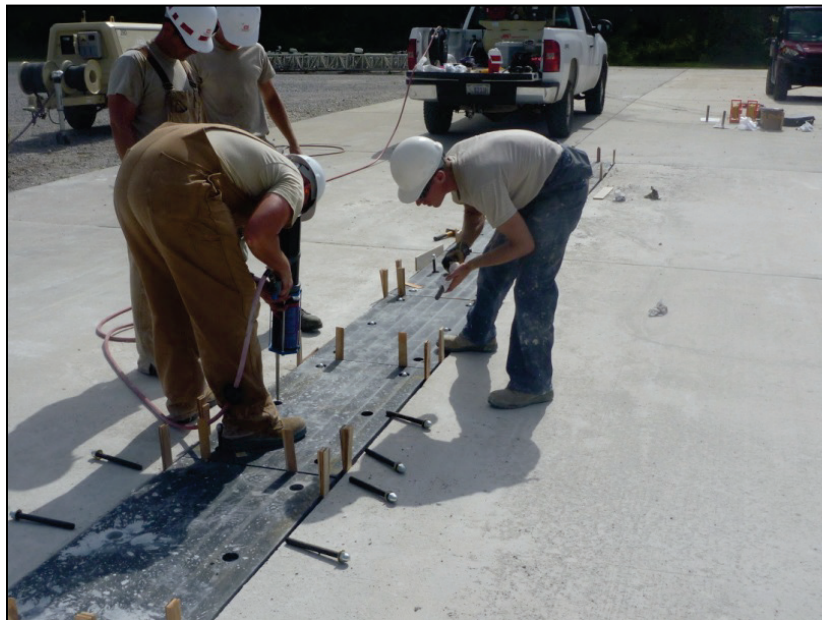
Figure A-24. Anchor installation.
