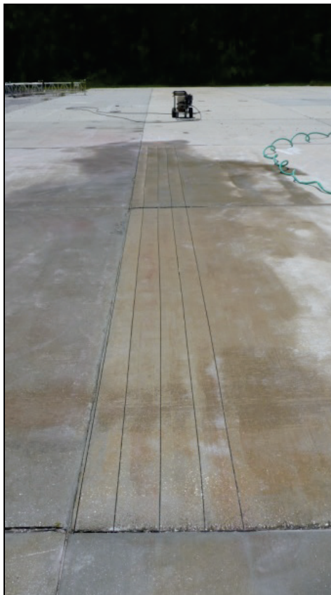
Figure A-6. Completed transverse cuts.
