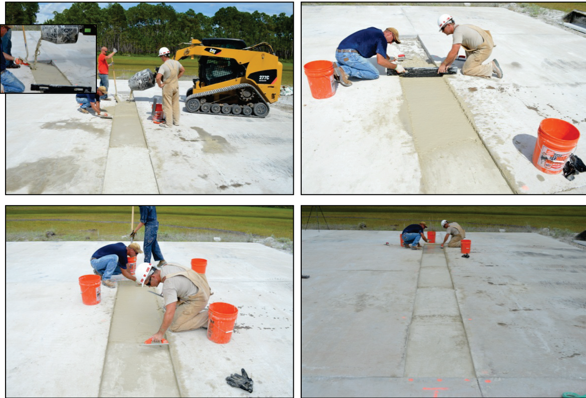
Figure E-15. Placing and finishing the bedding material.
