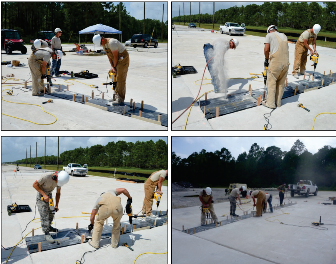
Figure B-18. Anchor hole production line.
