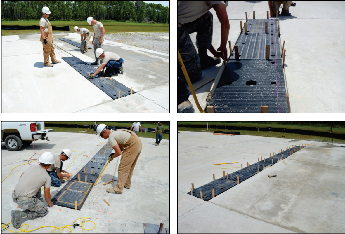
Figure A-20. Aligning panels within the slot.
