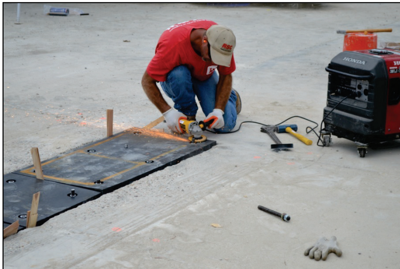
Figure B-25. Grinding anchor head flush with the panel surface.
