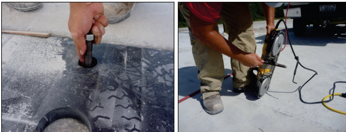
Figure B-20. Trimming a panel anchor.
