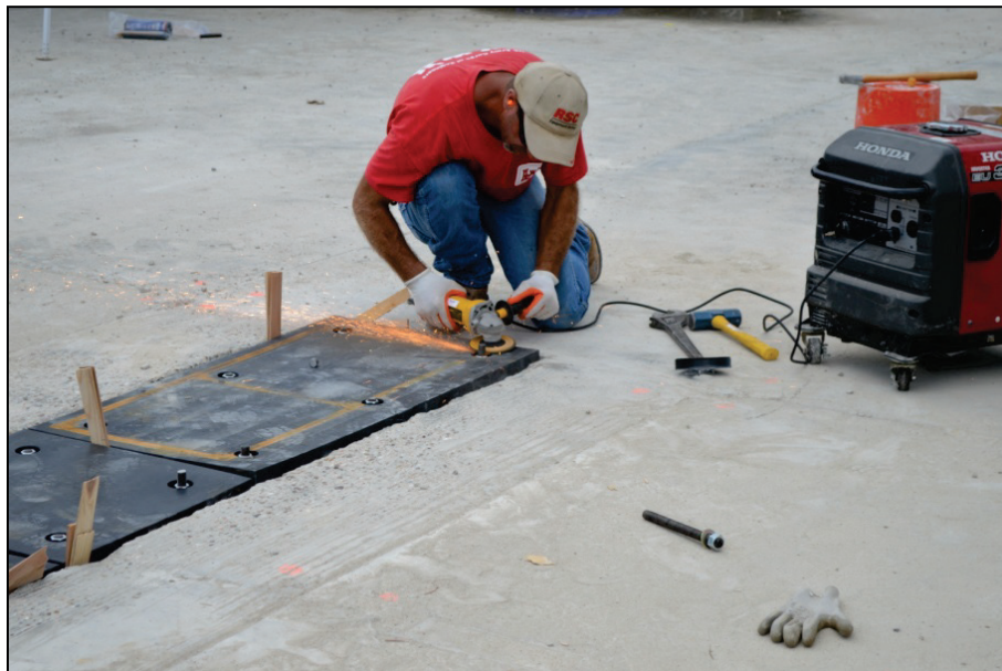
Figure D-6. Grinding an anchor head flush with the panel surface.
