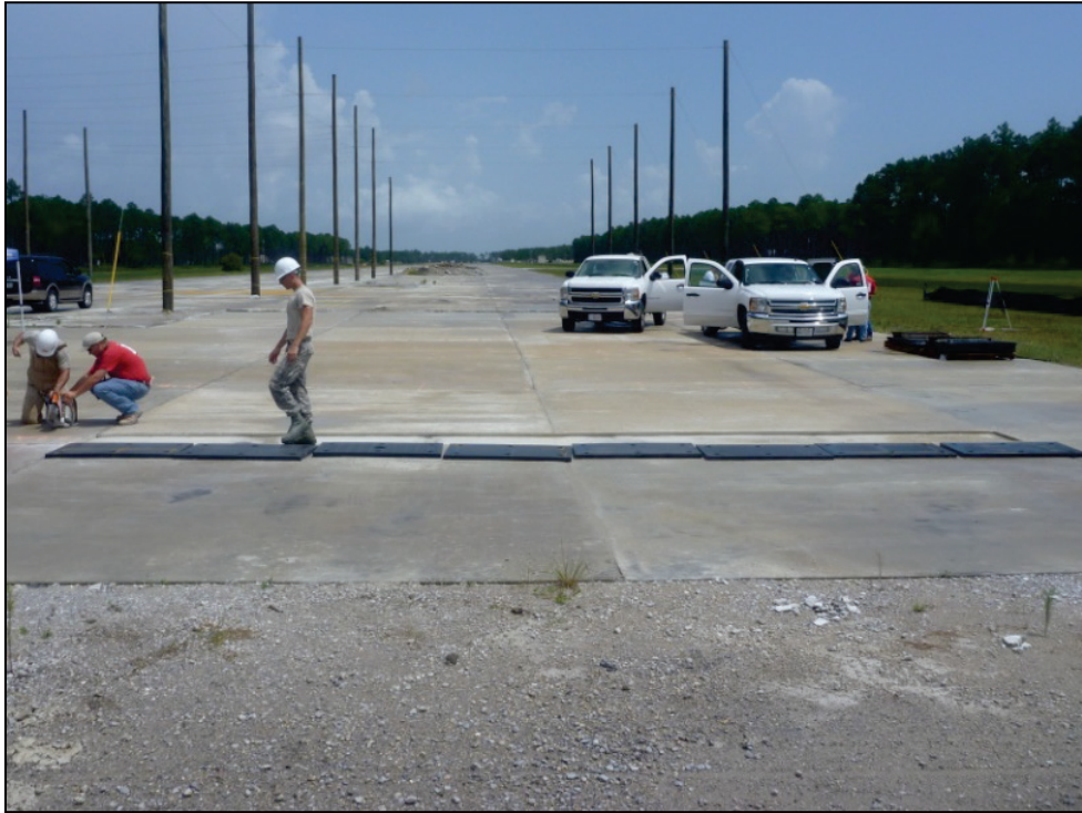
Figure C-20. Arranging panels.
