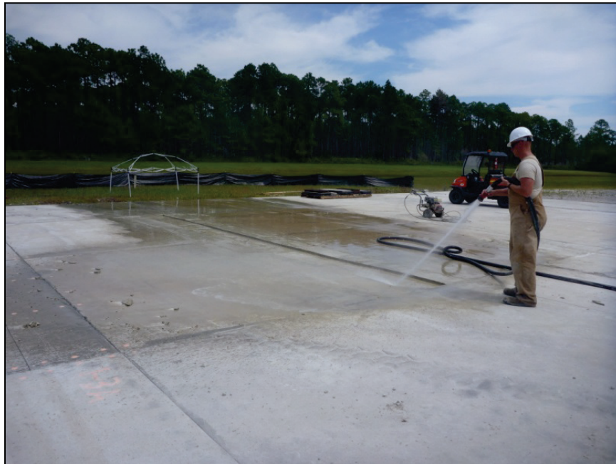
Figure E-5. Lightly rinsing the surface while sawing.
