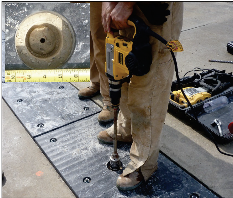
Figure 8. Dry cutting core barrel.
