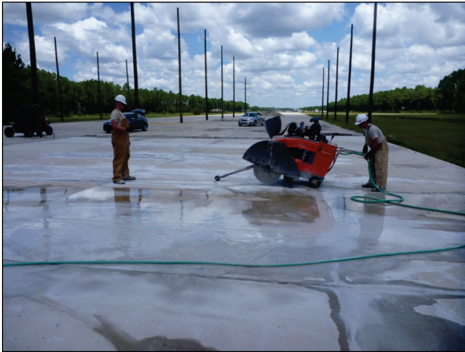
Figure C-2. Making transverse cuts with the floor saw.
