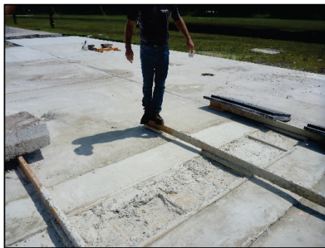
Formwork lifted from surface
