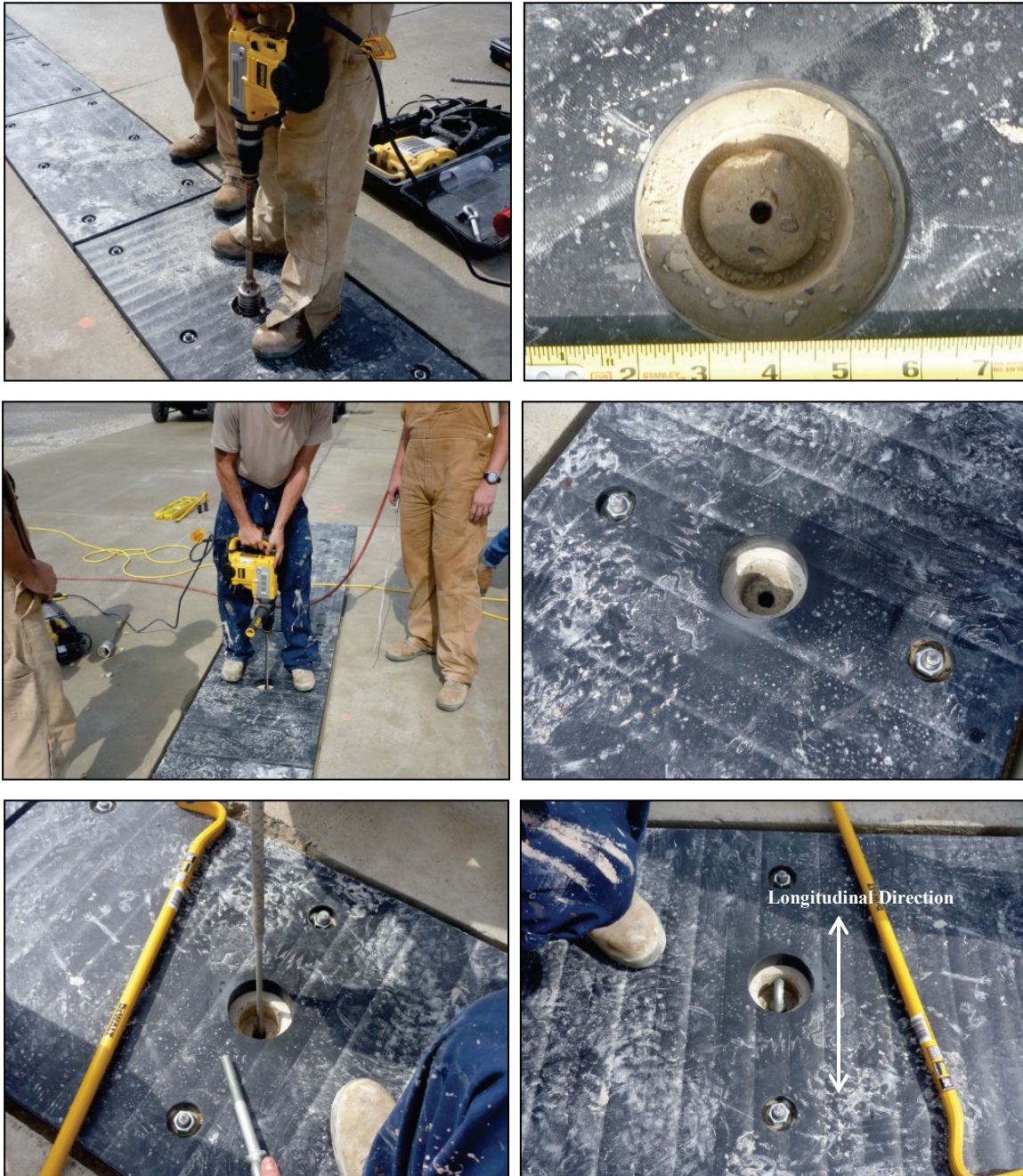
Figure D-1. Tie-down anchorage installation.
