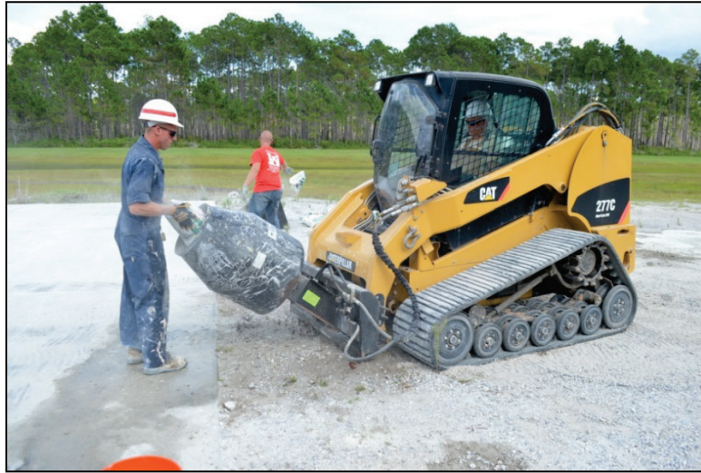
Figure A-13. Batching concrete with CTL.
