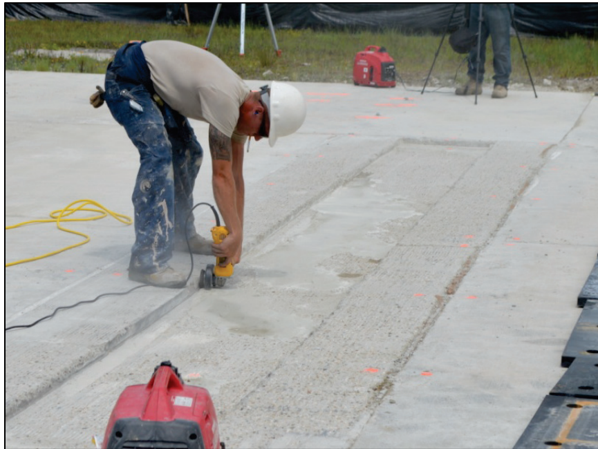
Figure E-18. Cleaning slot perimeter.
