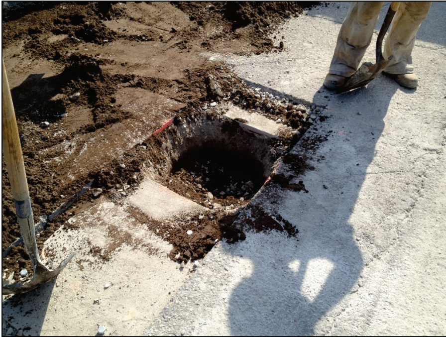
Figure 45. Augered hole after construction.
