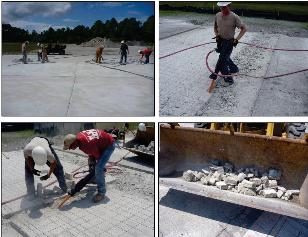
Figure E-11. Chiseling concrete within the repair void.
