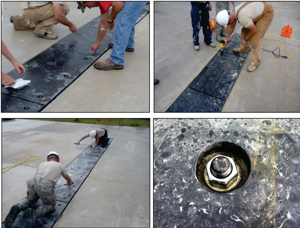
Figure C-29. Permanent hardware installation.
