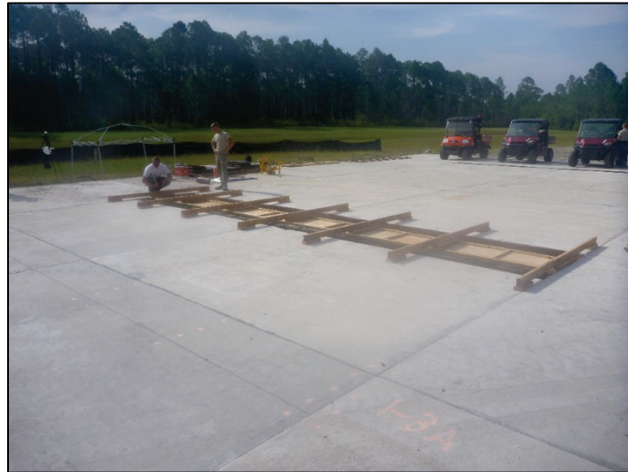
Figure 20. Wooden formwork used for the panel slot in new concrete placement.
