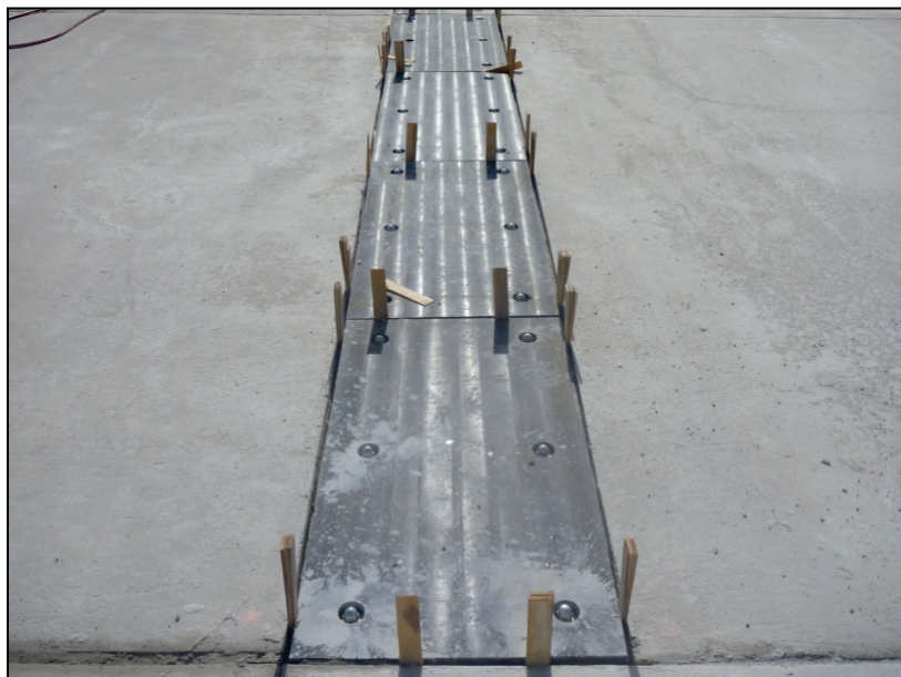
Figure A-25. After all anchors are installed.
