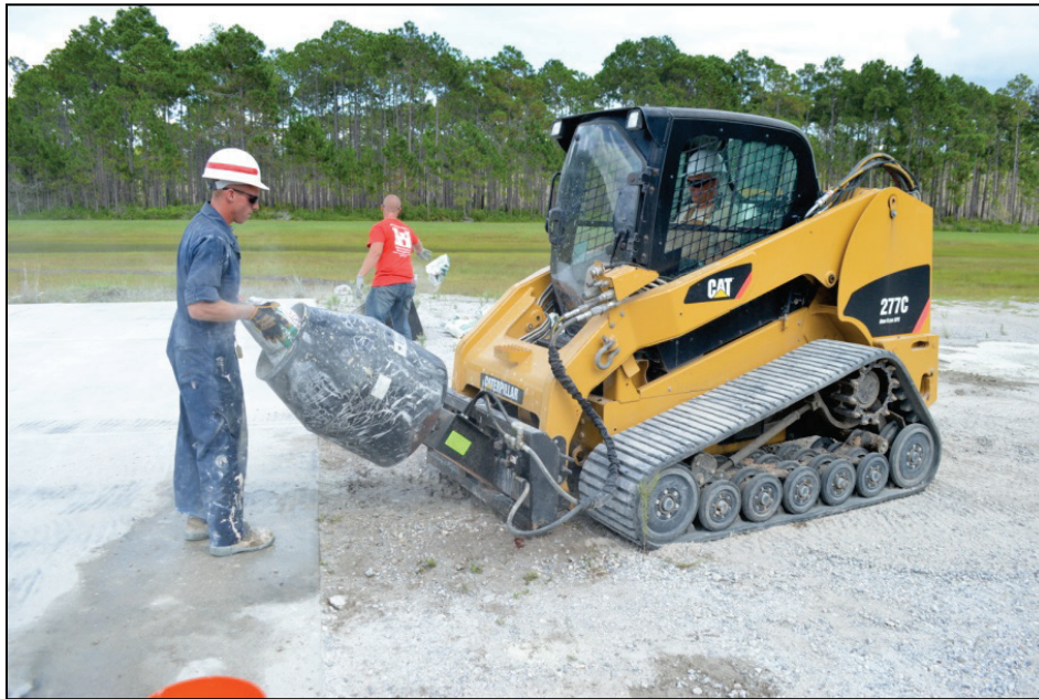
Figure E-14. Batching concrete with CTL.
