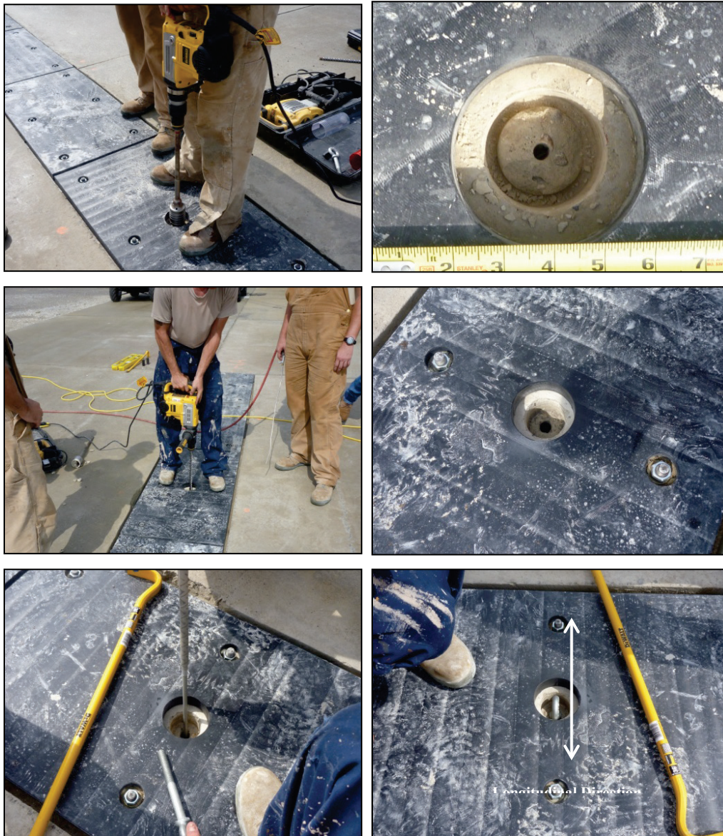
Figure A-26. Tie-down anchorage installation.
