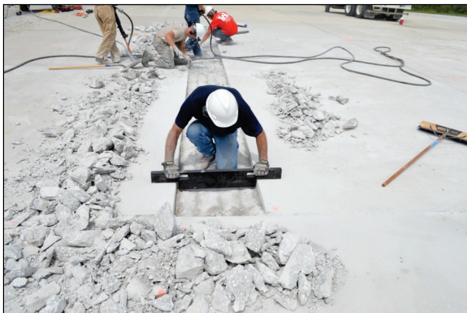
Figure E-13. Checking the slot depth.
