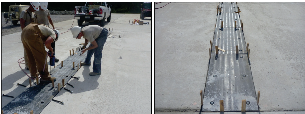
Figure D-4. Anchor installation.
