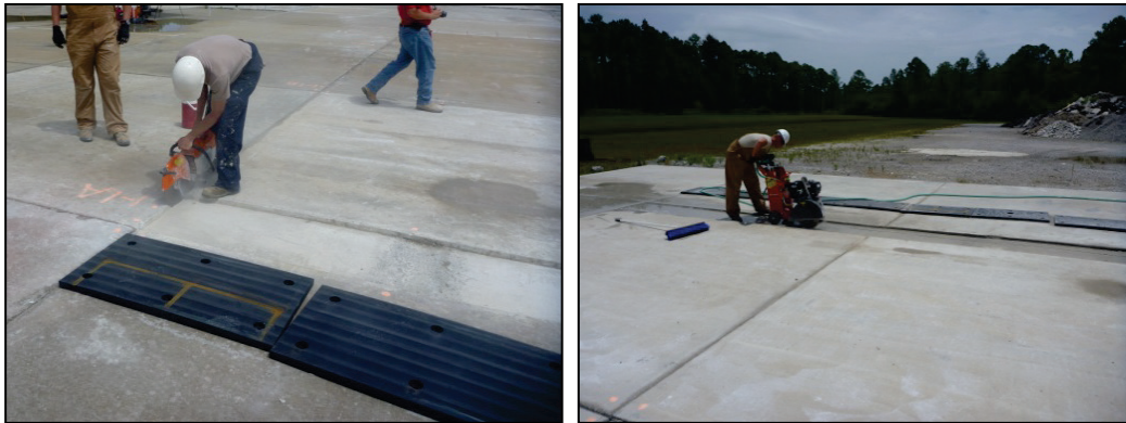
Figure E-17. Joint cutting.
