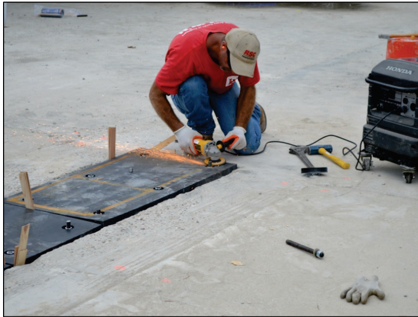
Figure A-28. Grinding an anchor head flush with the panel surface.
