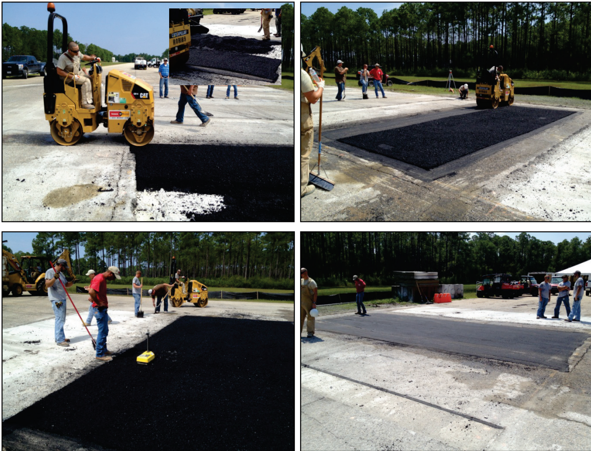
Figure C-12. Compacting asphalt patch.
