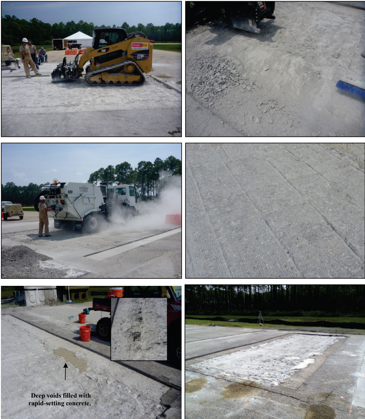
Figure C-10. Milling rough surface of patch area.
