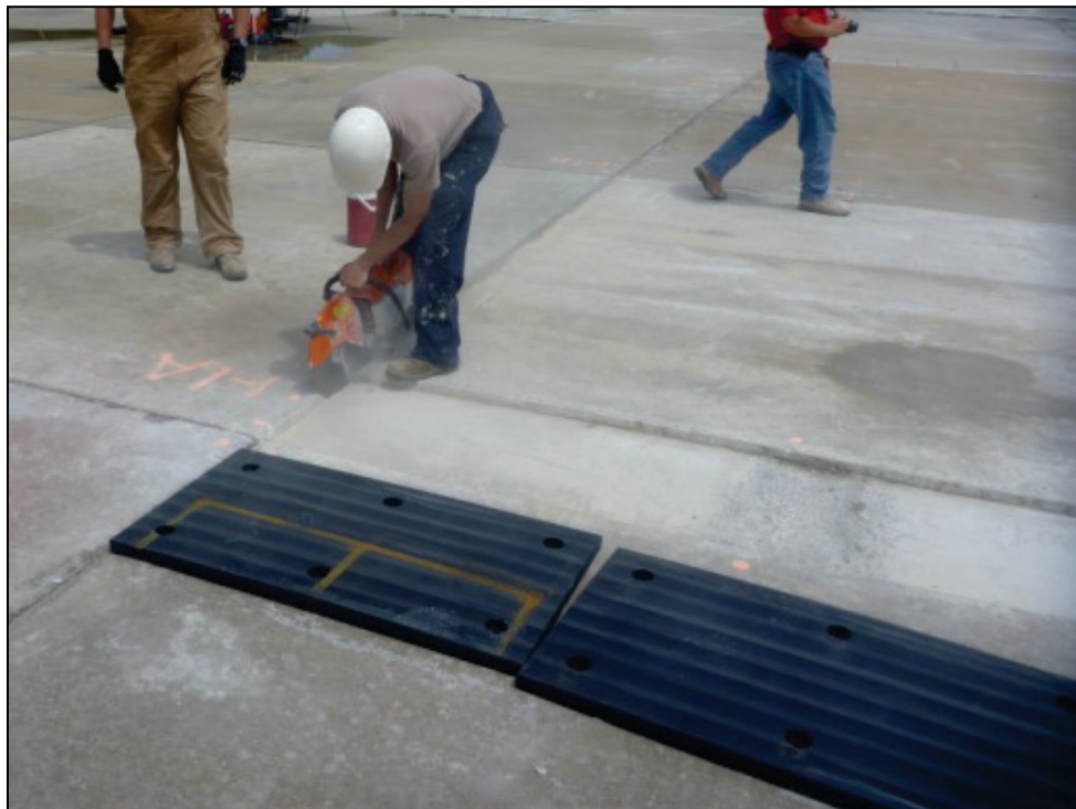
Figure C-21. Joint cutting.
