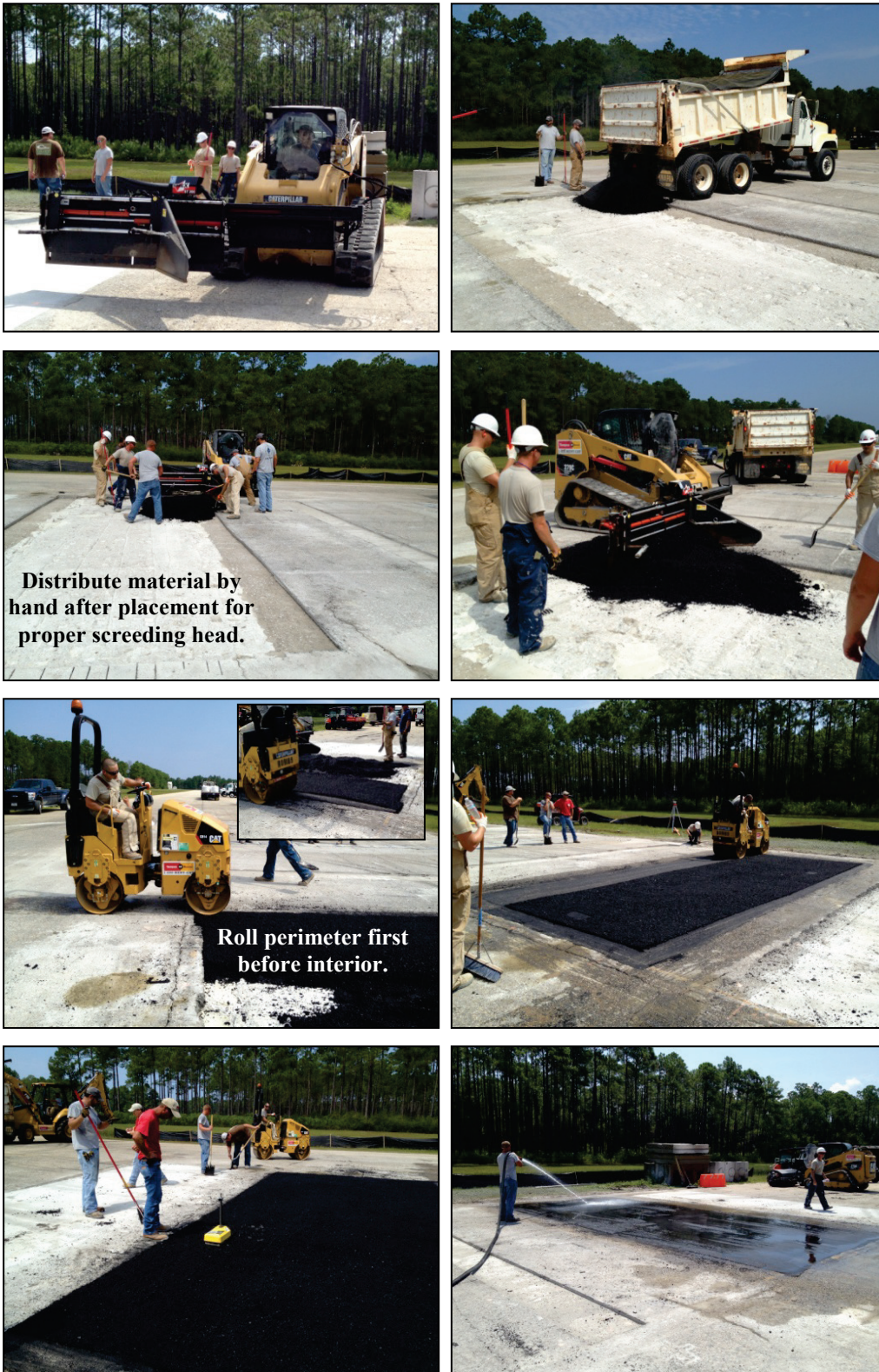
Figure E-42. Asphalt placement.
