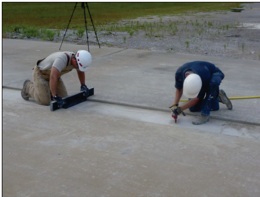
Figure E-37. Final leveling of the panel slot.
