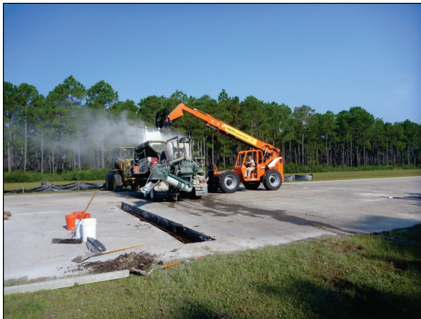
Figure E-35. Placing rapid setting concrete.
