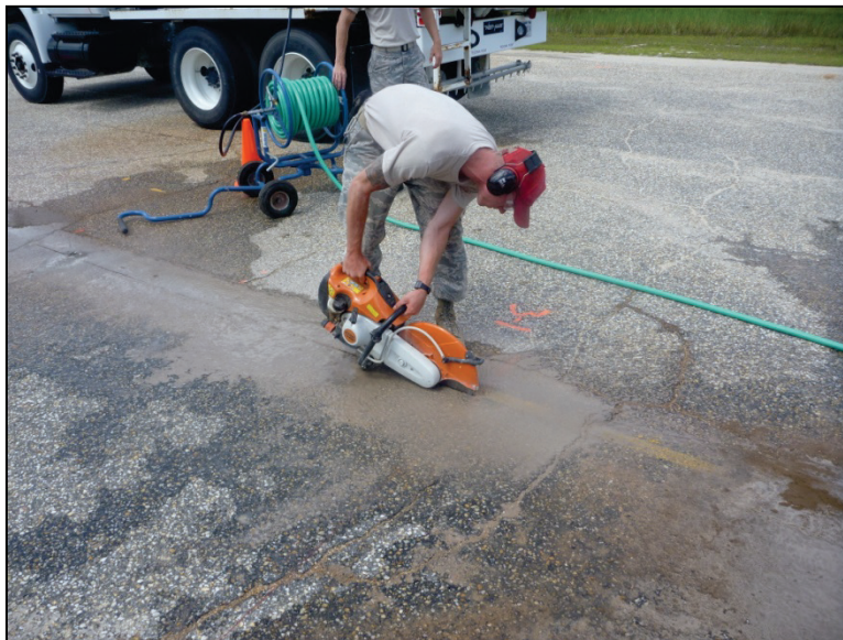
Figure B-4. Making longitudinal cuts.
