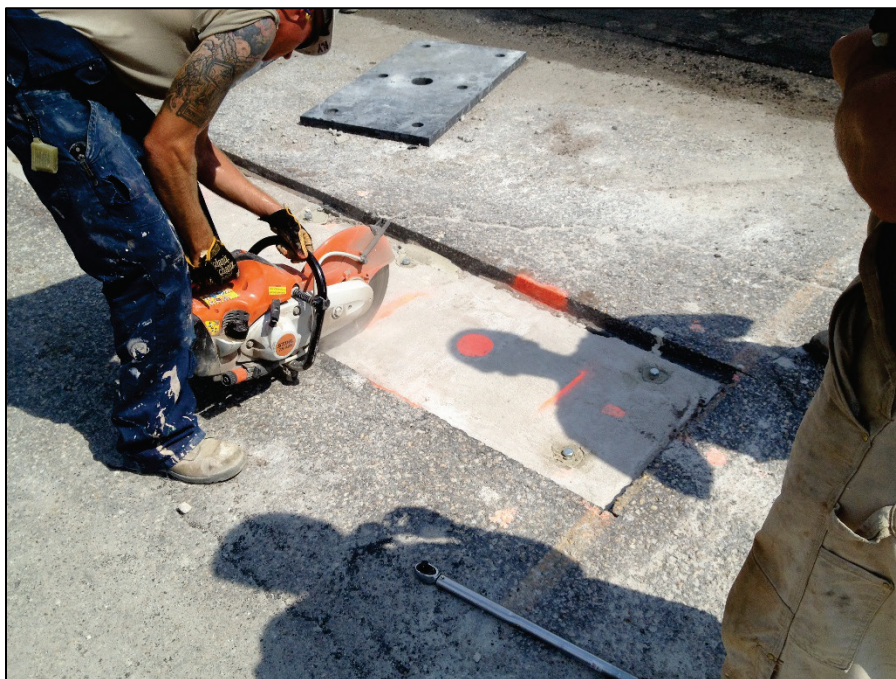
Figure 42. Demolishing filling material for tie-down anchor installation.
