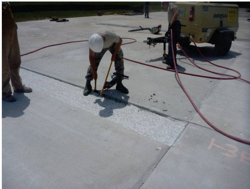
Figure 26. Removal of unmilled portion of concrete with hand tools.
