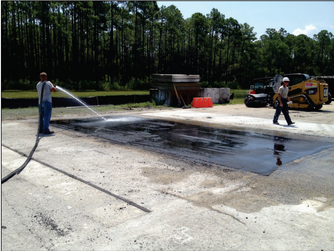
Figure D-18. Watershocking freshly compacted asphalt pavement by hand.
