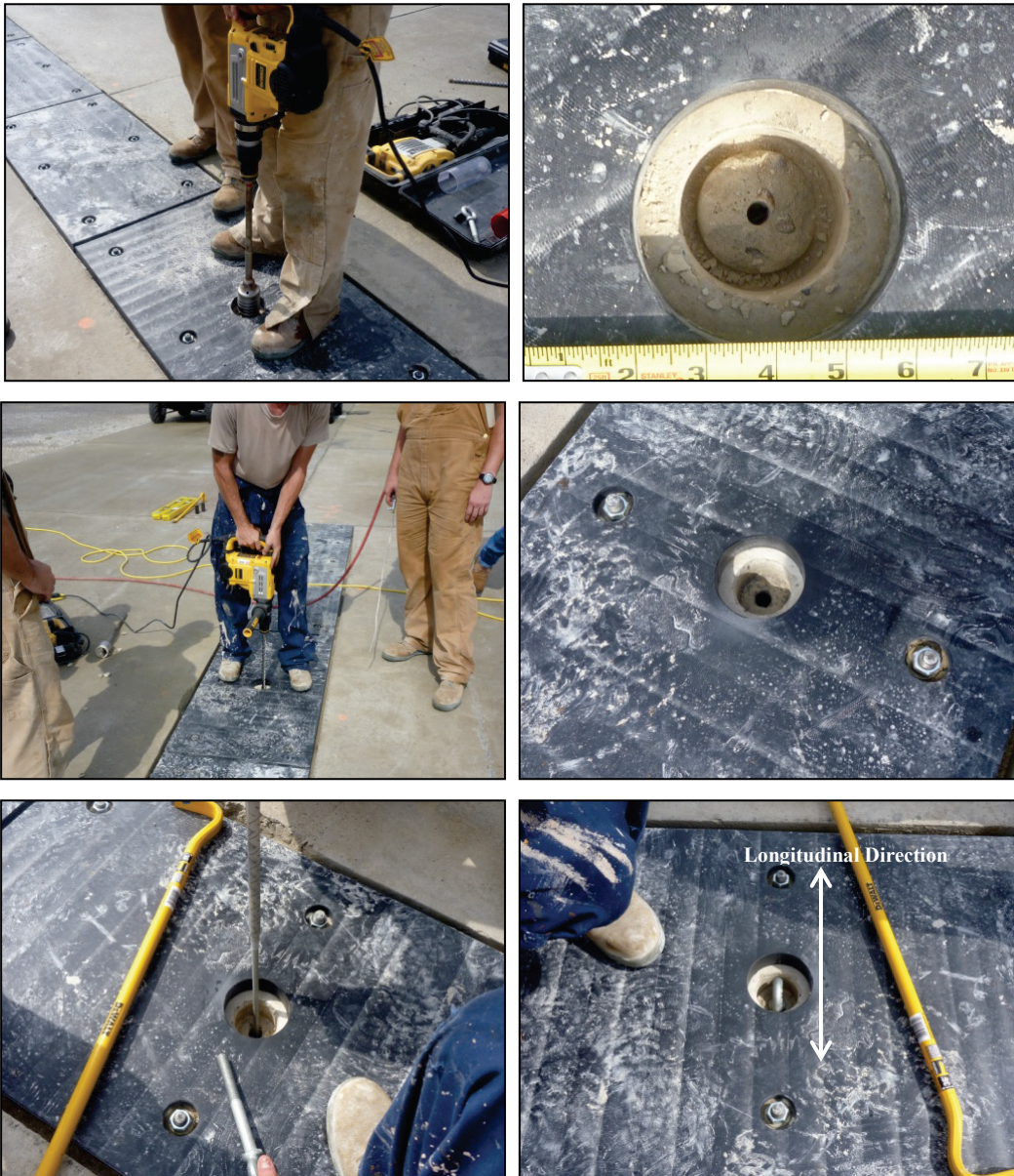
Figure B-23. Tie-down anchorage installation.
