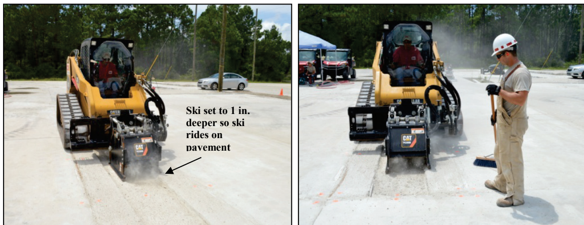
Figure E-41. Milling the pavement for the patch.
