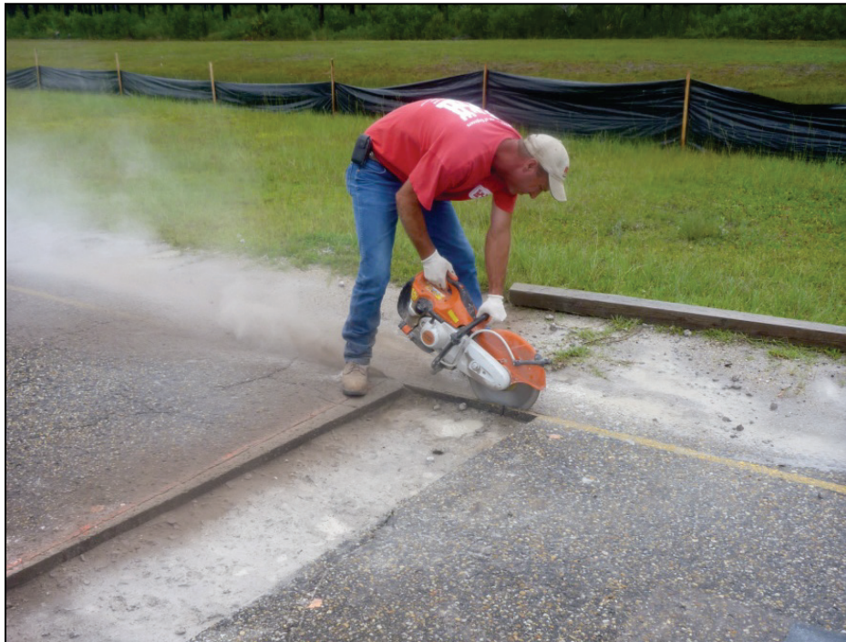
Figure B-7. Trimming the remaining pavement.
