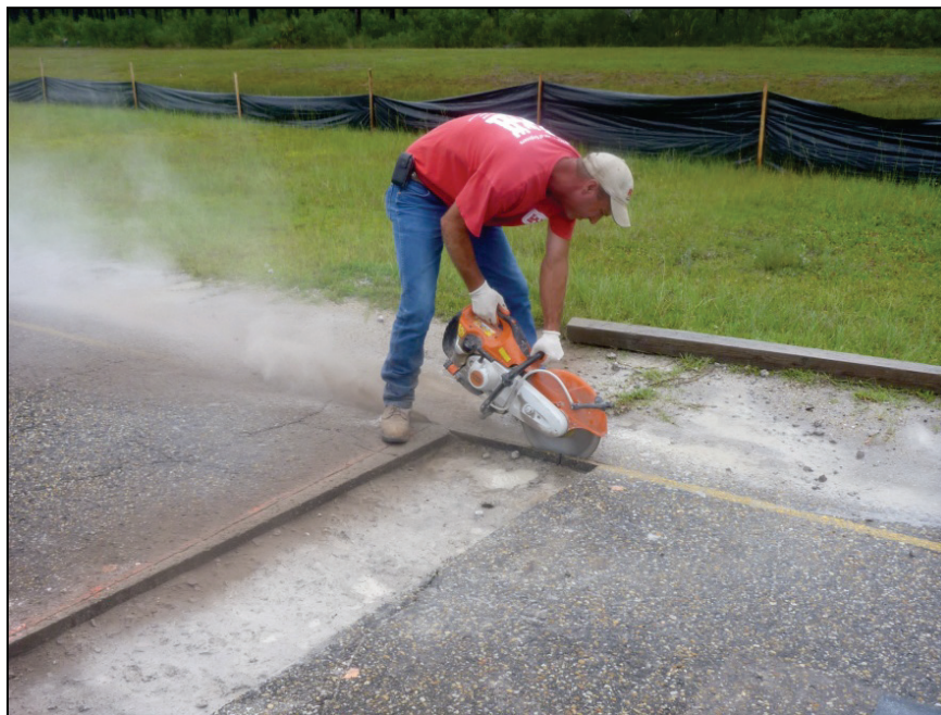
Figure E-29. Trimming the remaining pavement.
