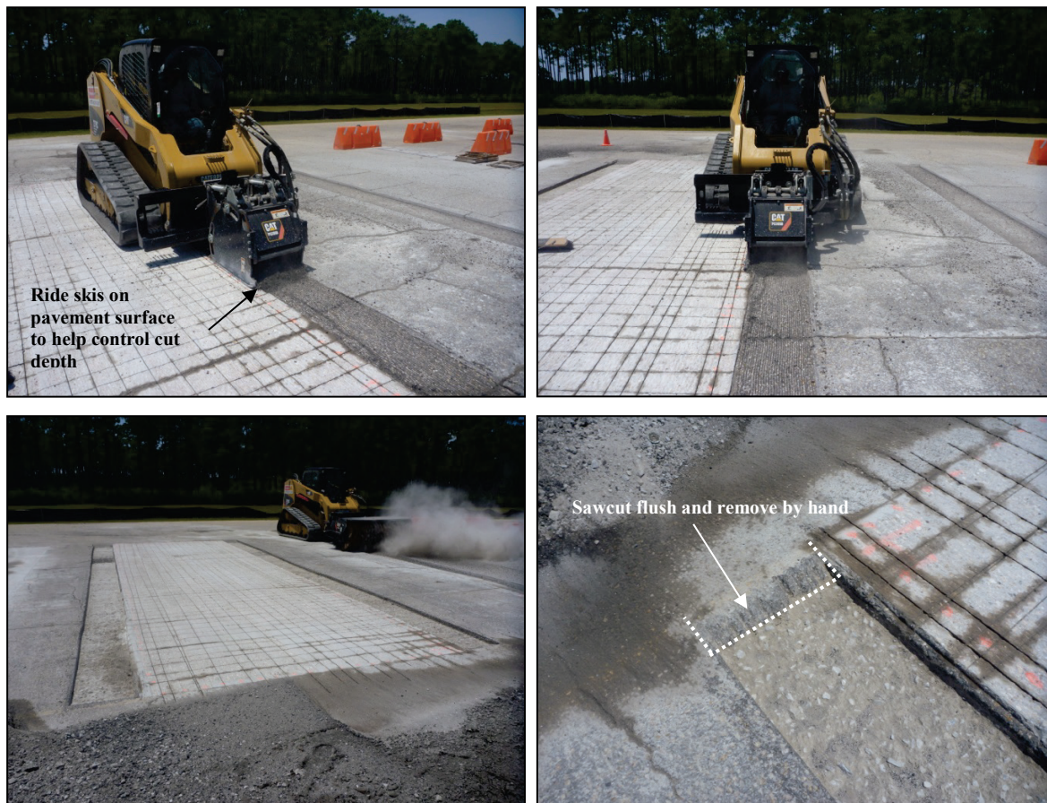
Figure D-13. Milling AC at construction joint.
