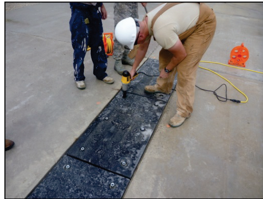
Gross tightening with impact hammer installing permanent hardware.
