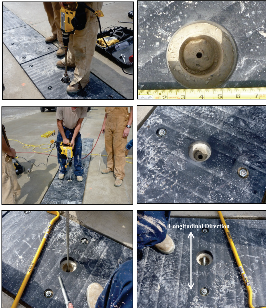
Figure E-43. Tie-down anchorage installation.
