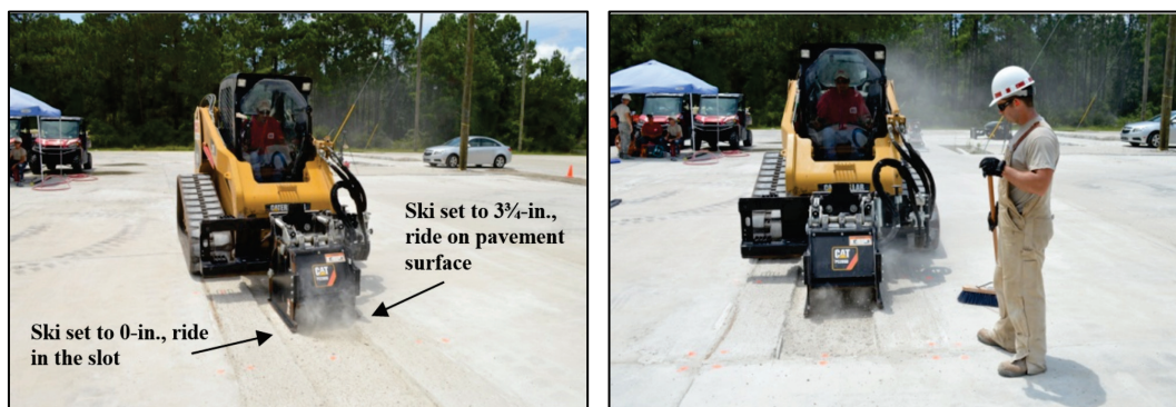
Figure A-11. Milling the panel slot.
