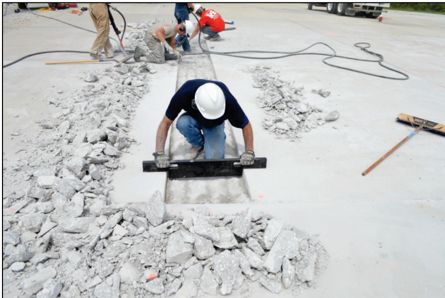
Figure A-12. Checking the slot depth.
