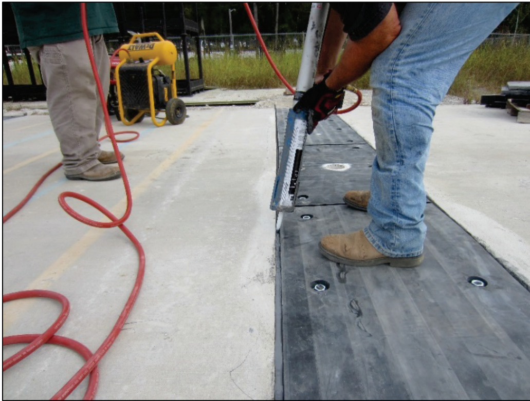
Figure E-45. Joint sealant installation.
