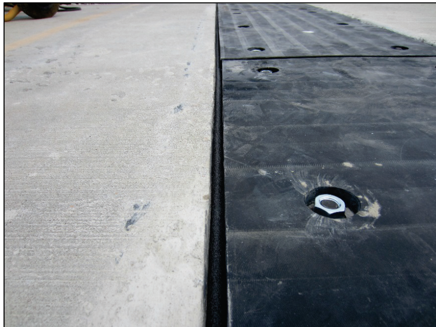
Figure D-22. Backer rod installation.
