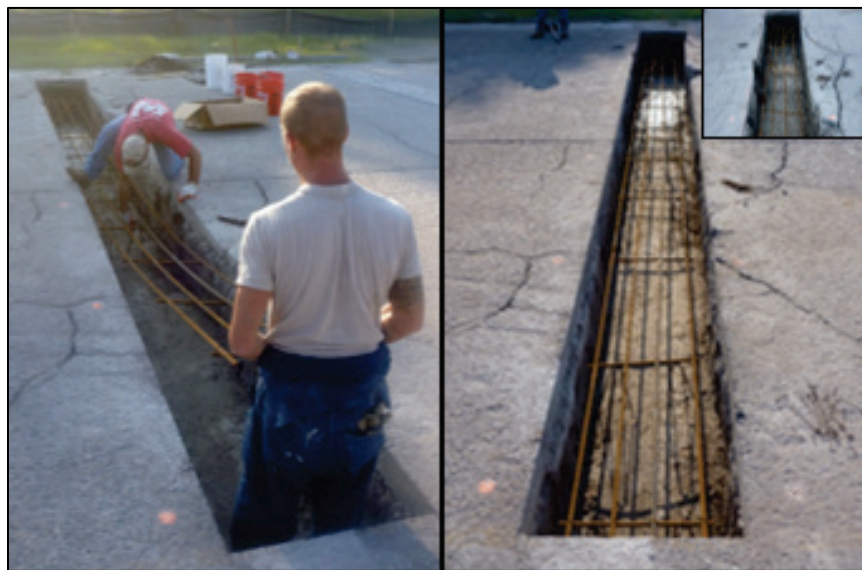
Figure 32. Reinforcement grid in traditional AC installation.
