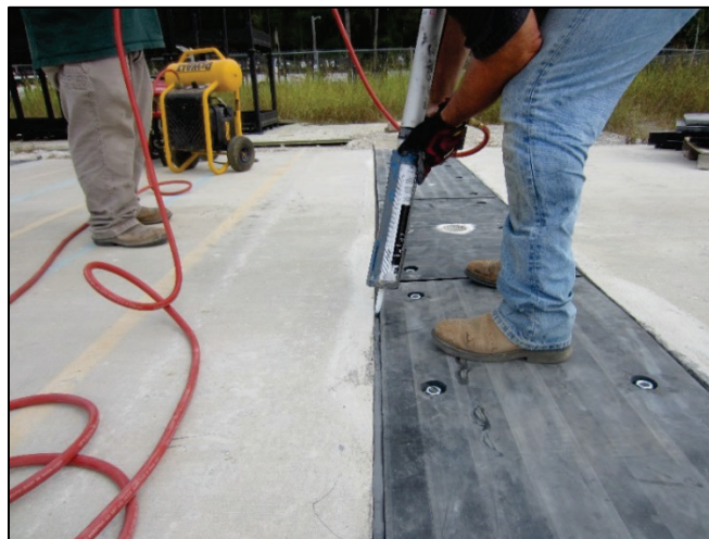
Figure A-31. Joint sealant installation.
