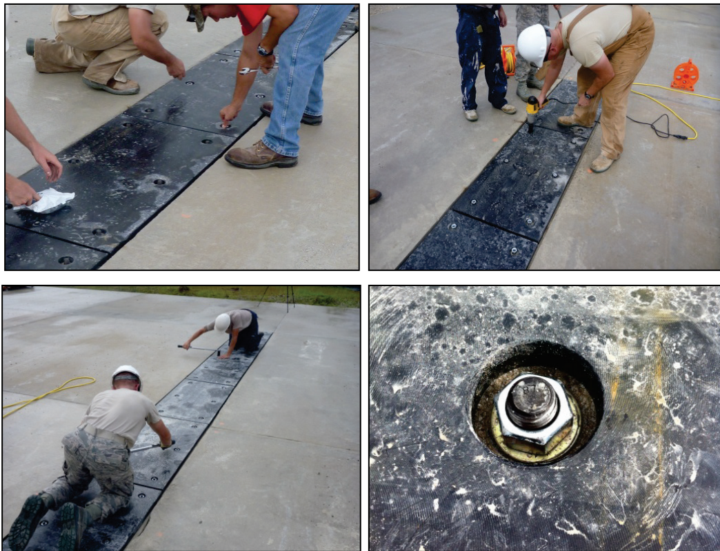
Figure A-27. Permanent hardware installation.
