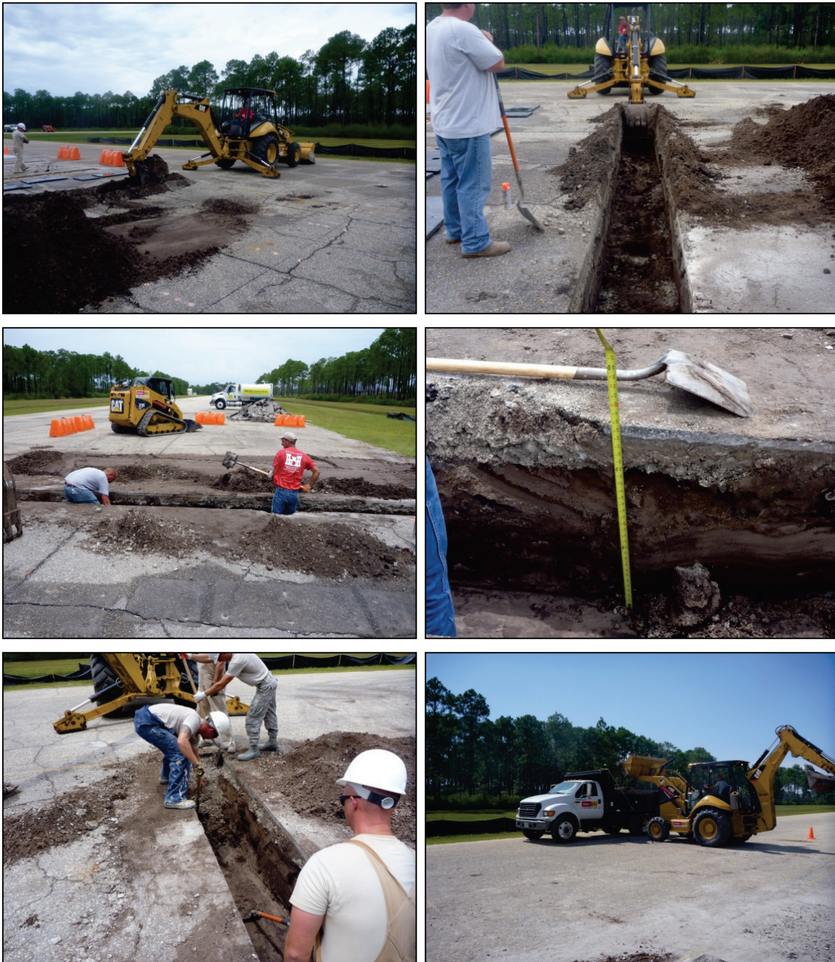
Figure B-8. Sublayer material removal.
