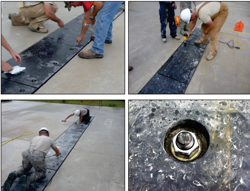
Figure E-25. Permanent hardware installation.
