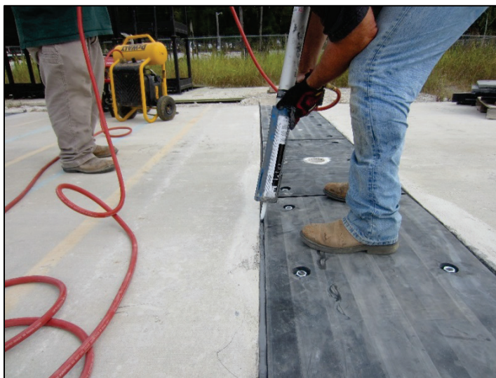
Figure D-23. Joint sealant installation.
