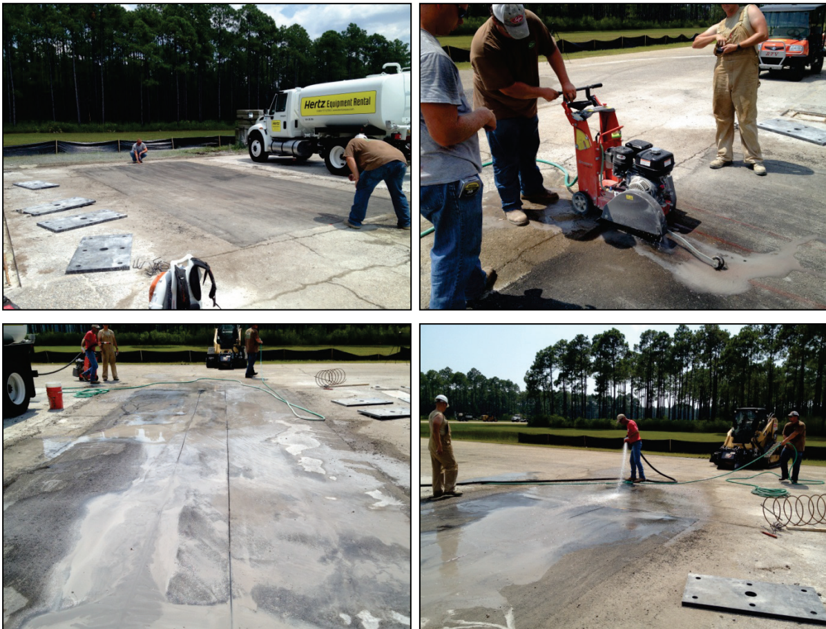
Figure C-16. Sawcutting new panel slot area.
