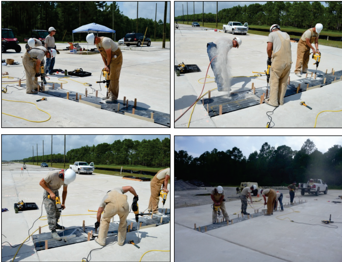
Figure D-3. Anchor hole installation.
