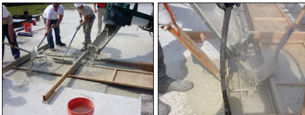
Figure 23. Concrete splatter during volumetric mixer placement.
