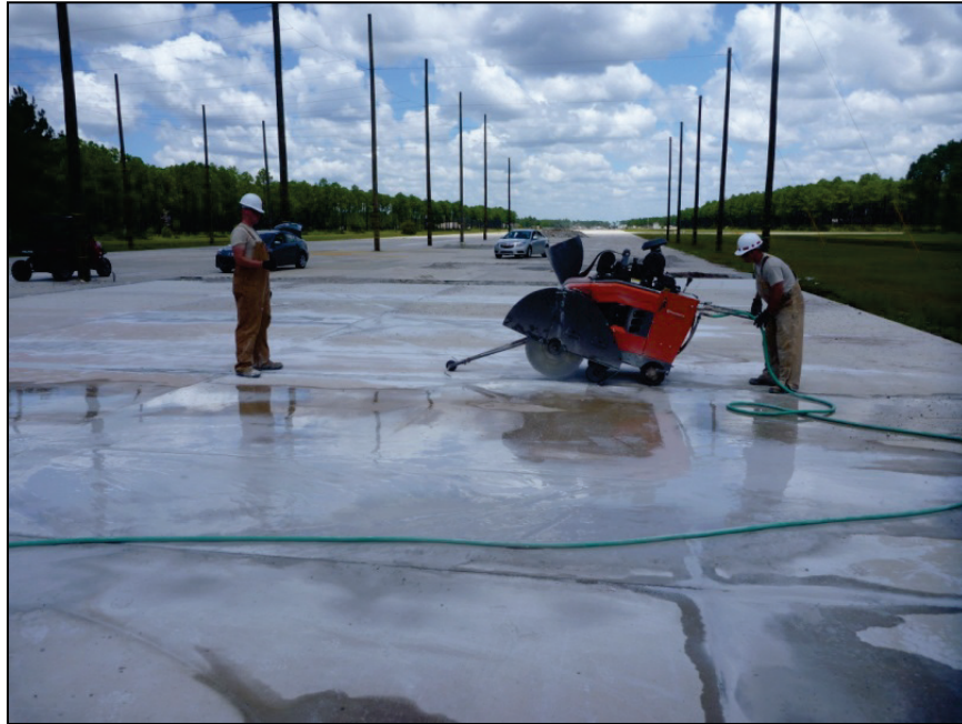
Figure E-6. Making transverse cuts on PCC areas.
