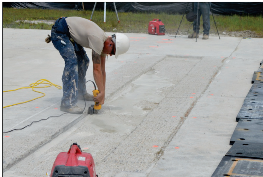
Figure A-17. Cleaning slot perimeter.
