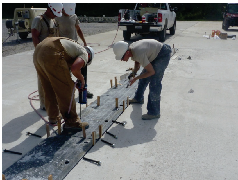
Figure B-21. Anchor installation.
