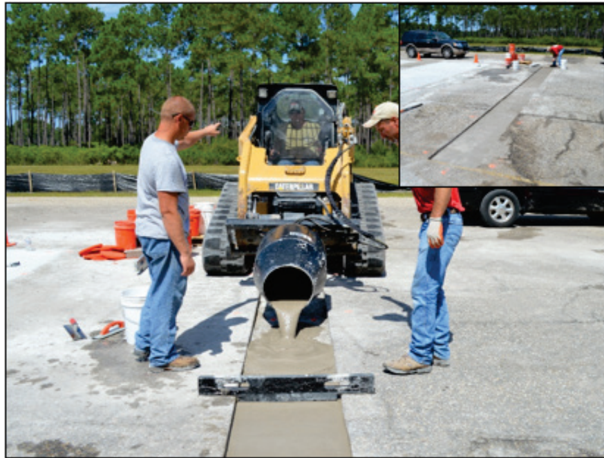
Figure 41. Installation of flowable fill for thin asphalt pavement surfaces.
