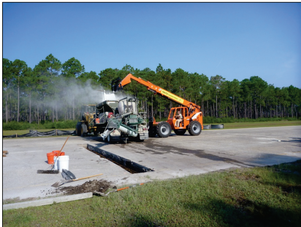
Figure B-13. Placing rapid setting concrete.
