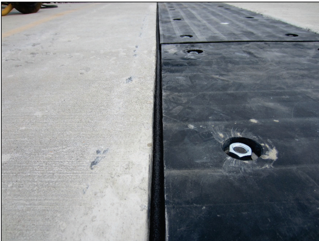
Figure B-29. Backer rod installation.
