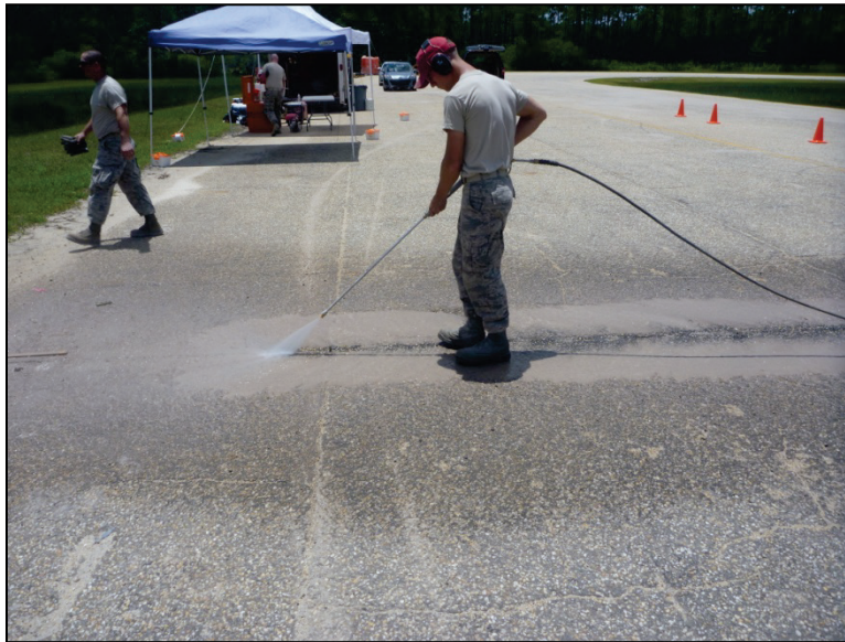
Figure B-5. Waterblasting saw slurry.
