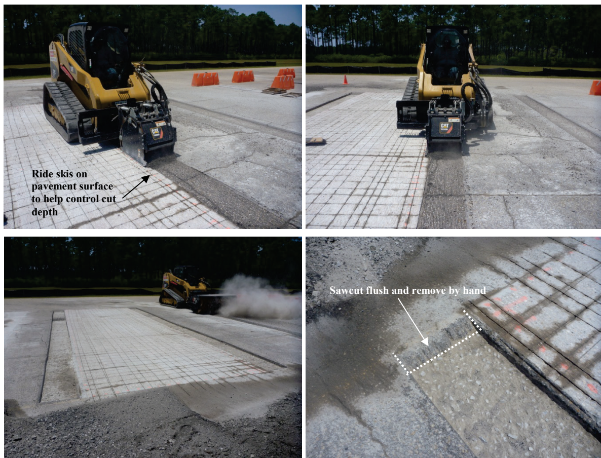
Figure C-8. Milling AC at construction joint.
