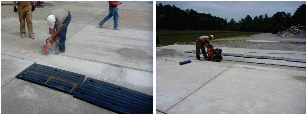
Figure A-16. Joint cutting.
