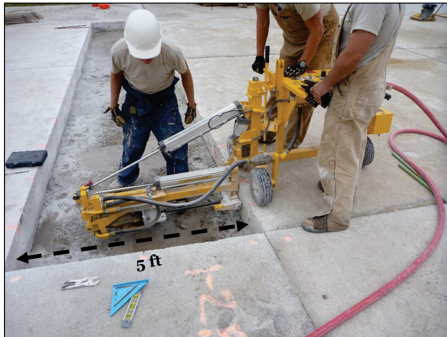
Figure 17. Concrete drill used in repair void.
