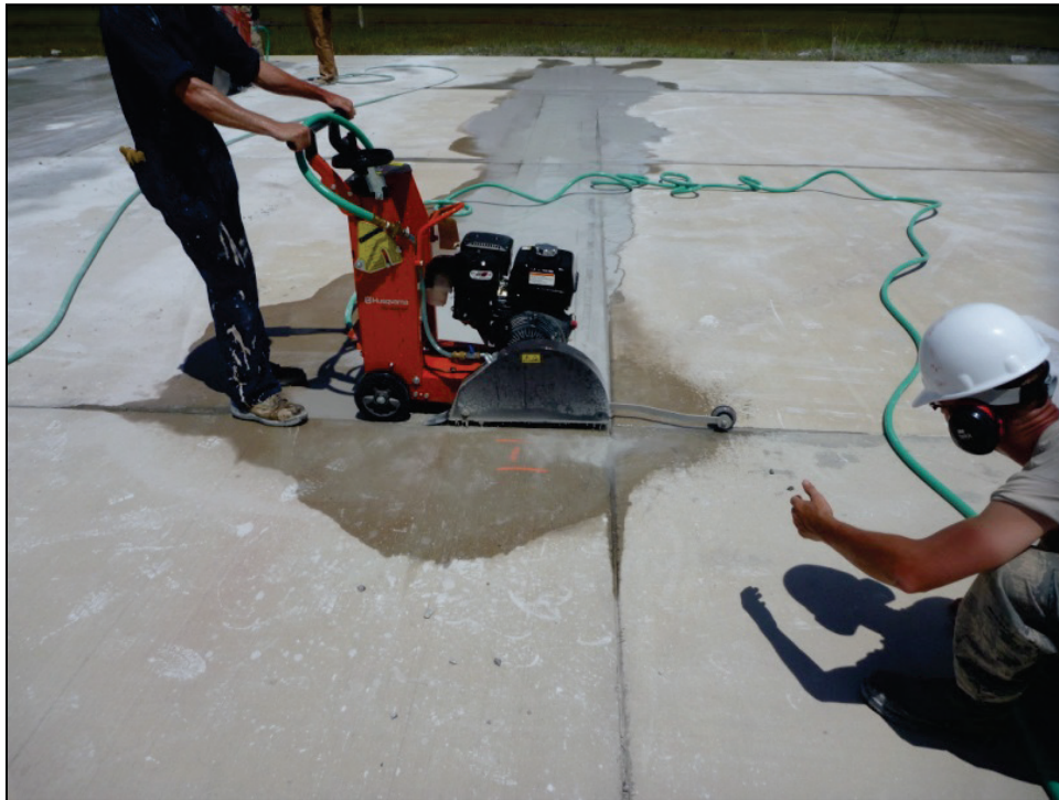
Figure C-6. Making longitudinal cuts.
