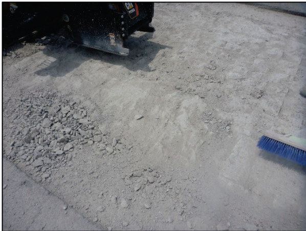
(c) 40 lb hammer with relief cuts.
