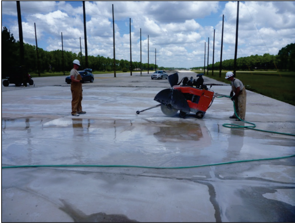
Figure A-3. Making transverse cuts.
