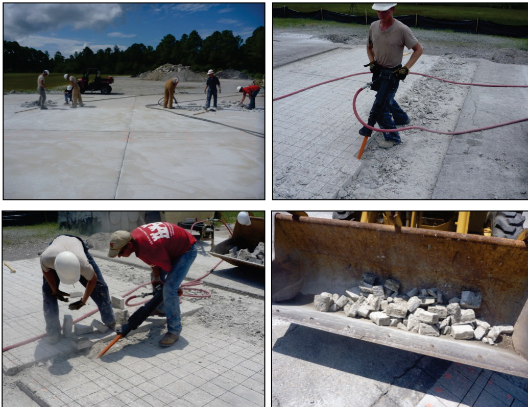
Figure A-10. Chiseling concrete within the repair void.
