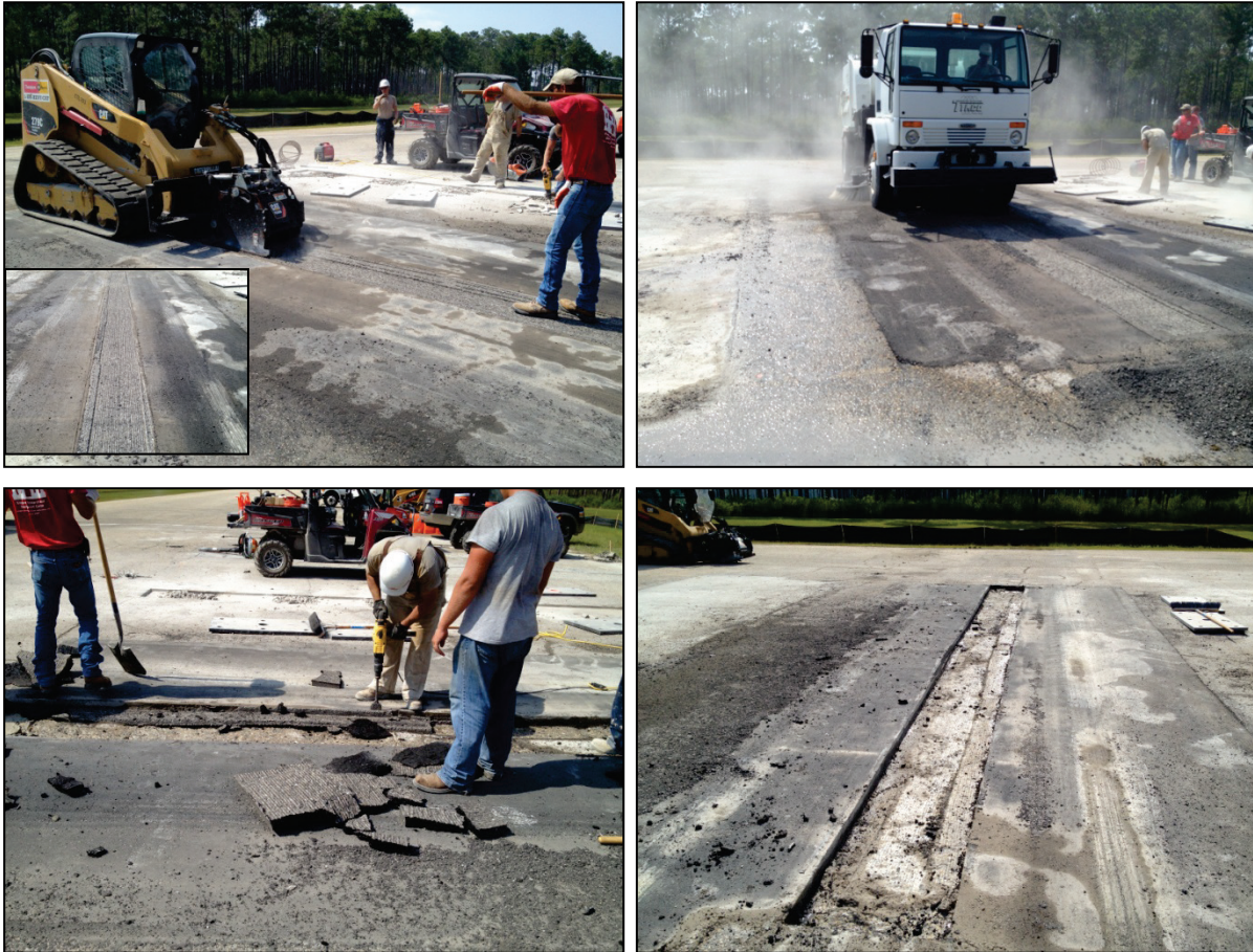
Figure C-17. Milling panel slot location.
