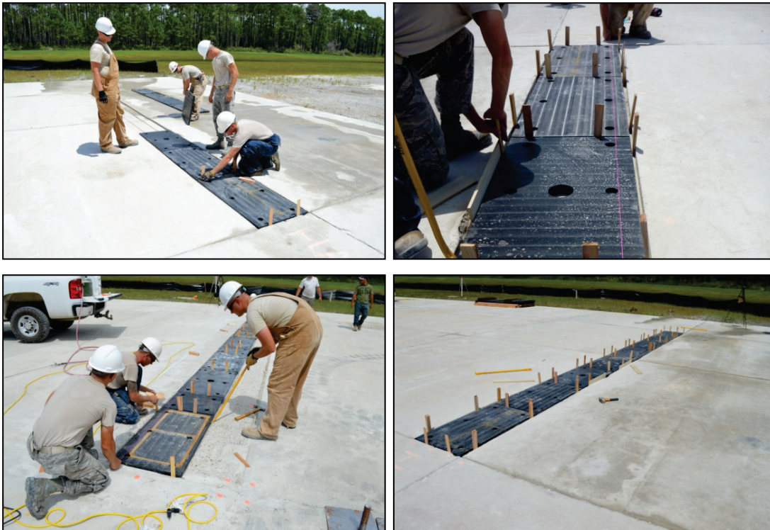
Figure E-20. Aligning panels within the slot.
