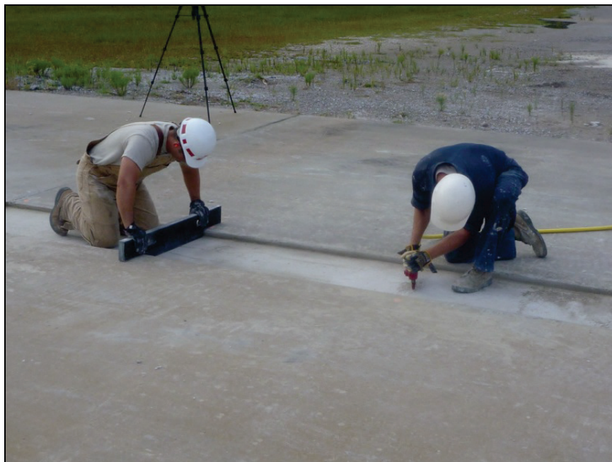
Figure E-19. Final leveling of the panel slot.
