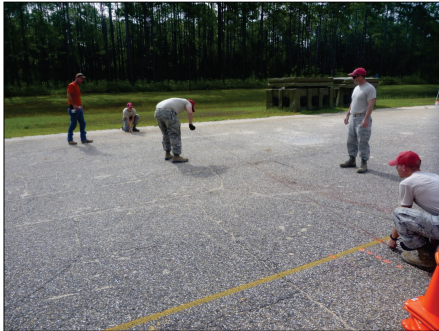
Figure B-2. Snapping chalklines.
