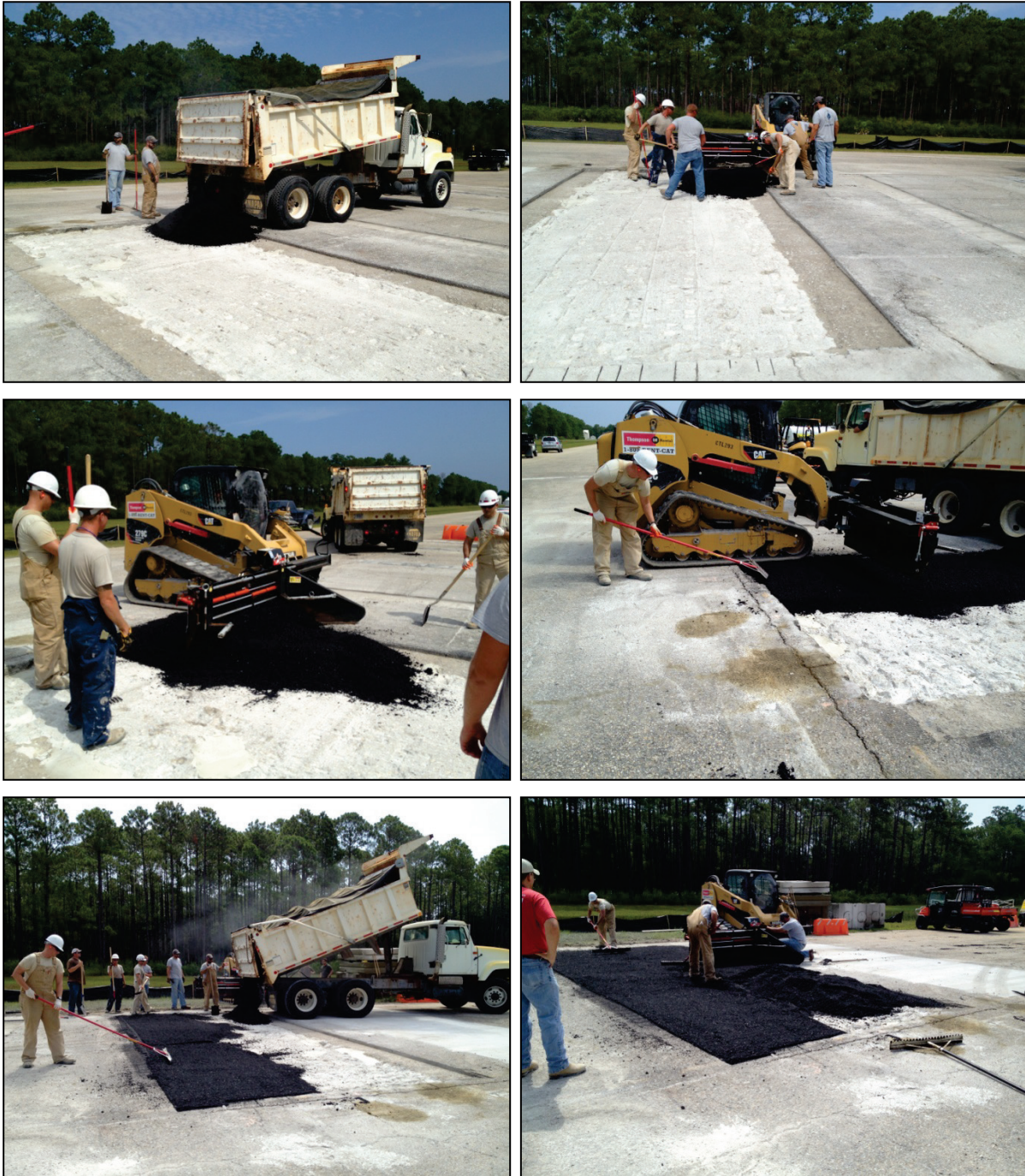
Figure C-11. Asphalt placement.
