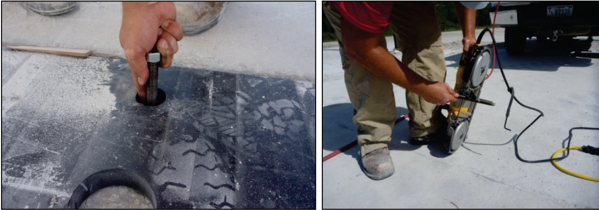
Figure A-23. Trimming a panel anchor.
