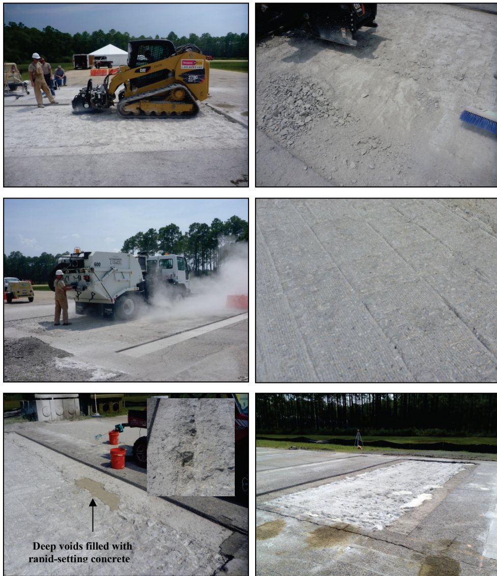
Figure D-15. Milling rough surface of patch area.
