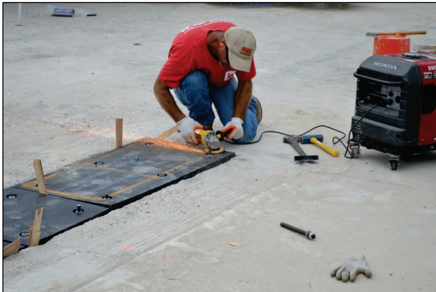
Figure C-30. Grinding an anchor head flush with the panel surface.
