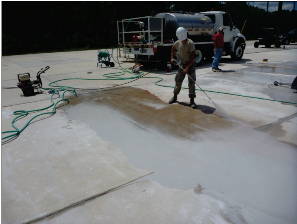
Figure D-9. Waterblasting saw slurry.
