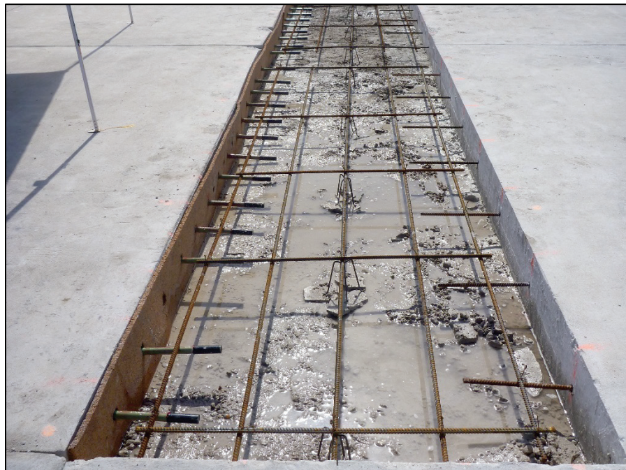
Figure 18. Repair reinforcement.
