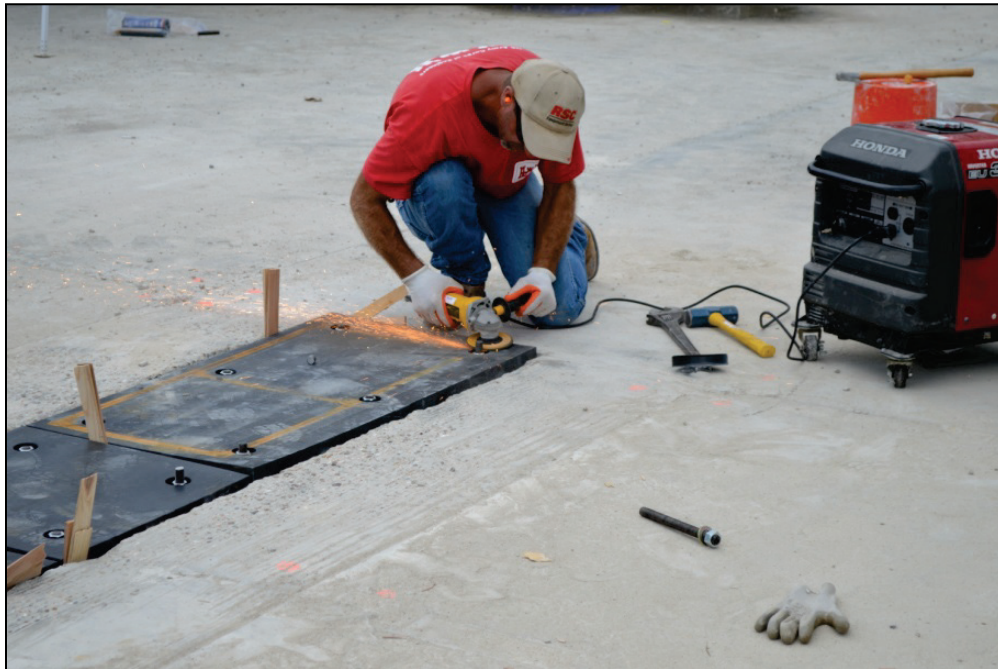
Figure E-26. Grinding an anchor head flush with the panel surface.
