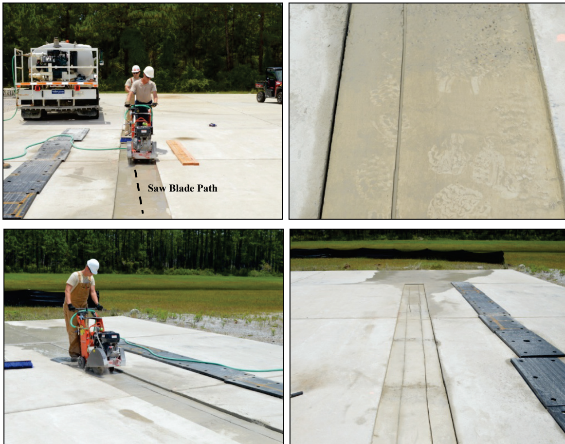
Figure B-16. Cutting drain slots.
