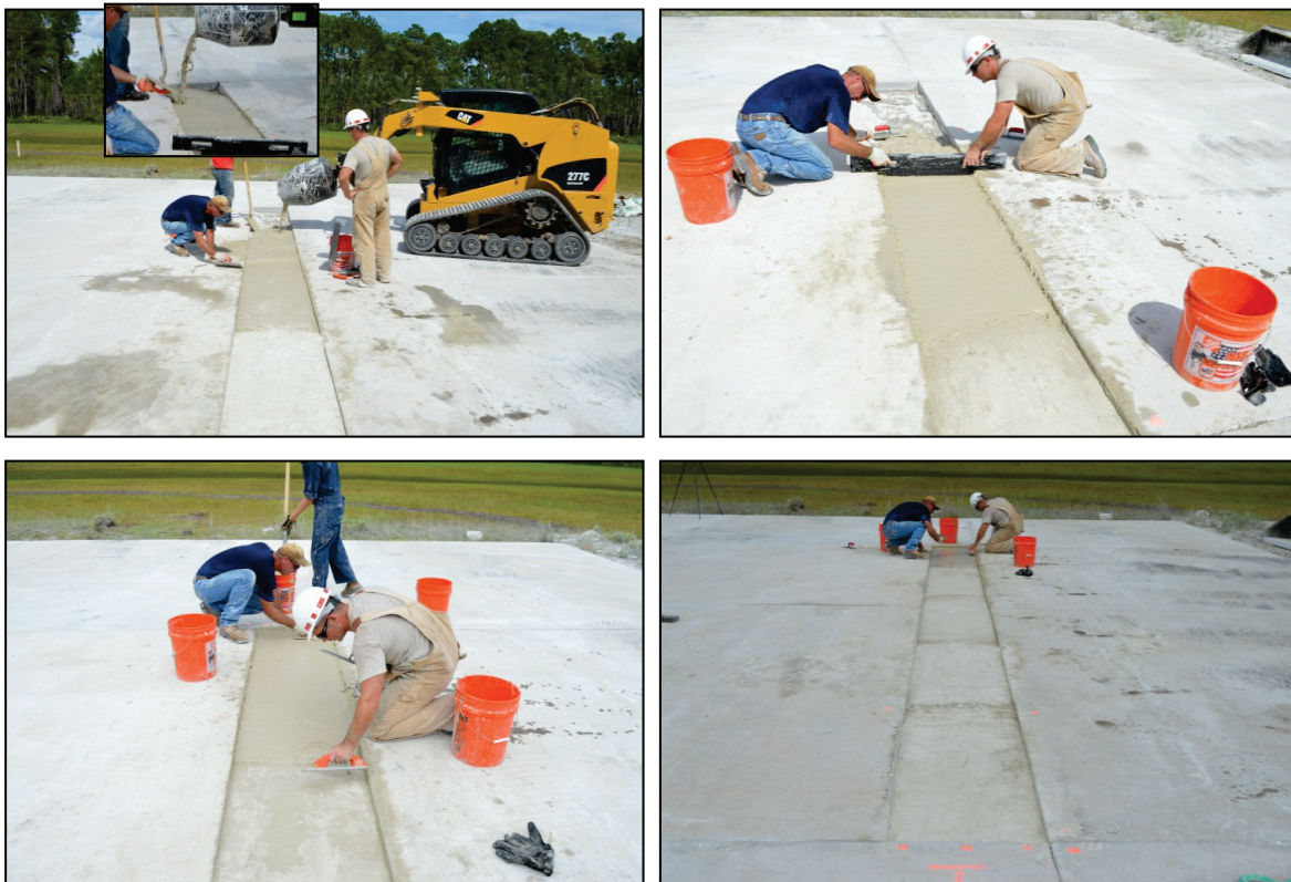
Figure C-19. Placing and finishing the bedding material.
