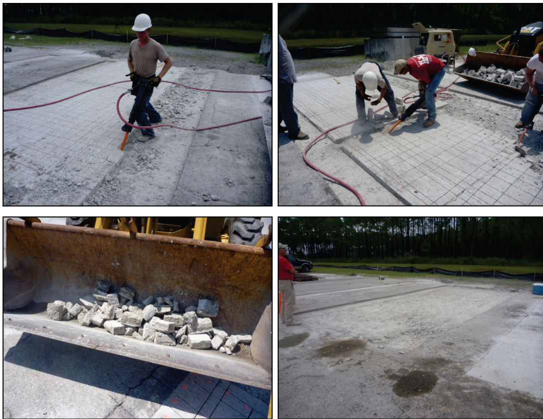
Figure D-14. Concrete foundation surface removal.
