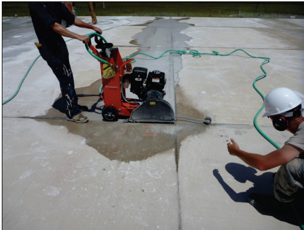
Figure A-8. Making longitudinal cuts.
