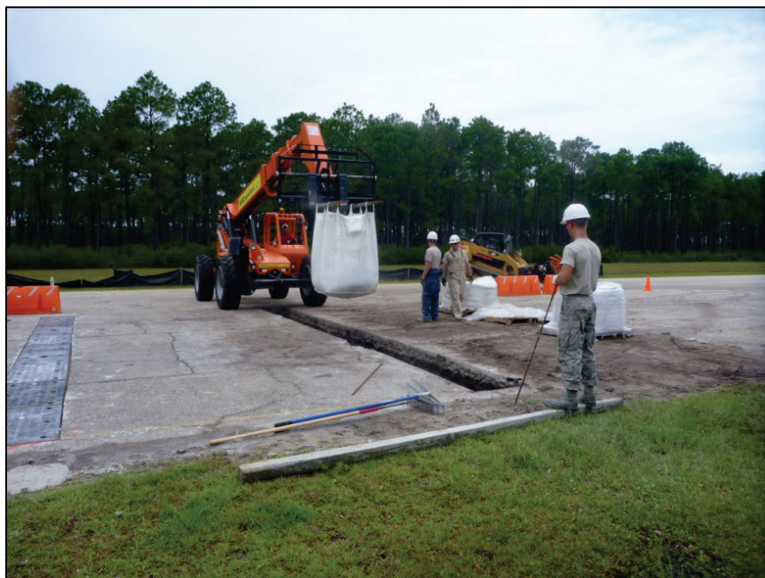
Figure E-31. Placing flowable fill (dry method).
