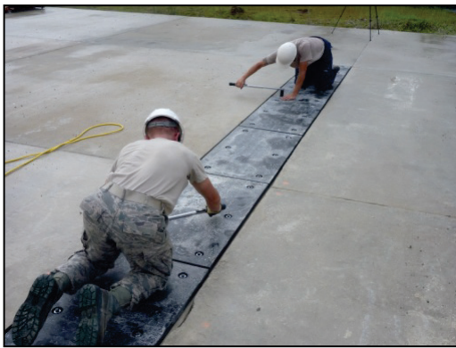
Fine tightening with torque wrench.
