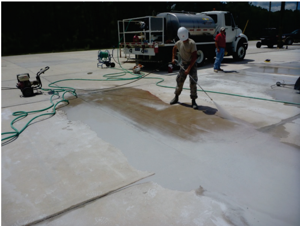
Figure C-4. Waterblasting saw slurry.
