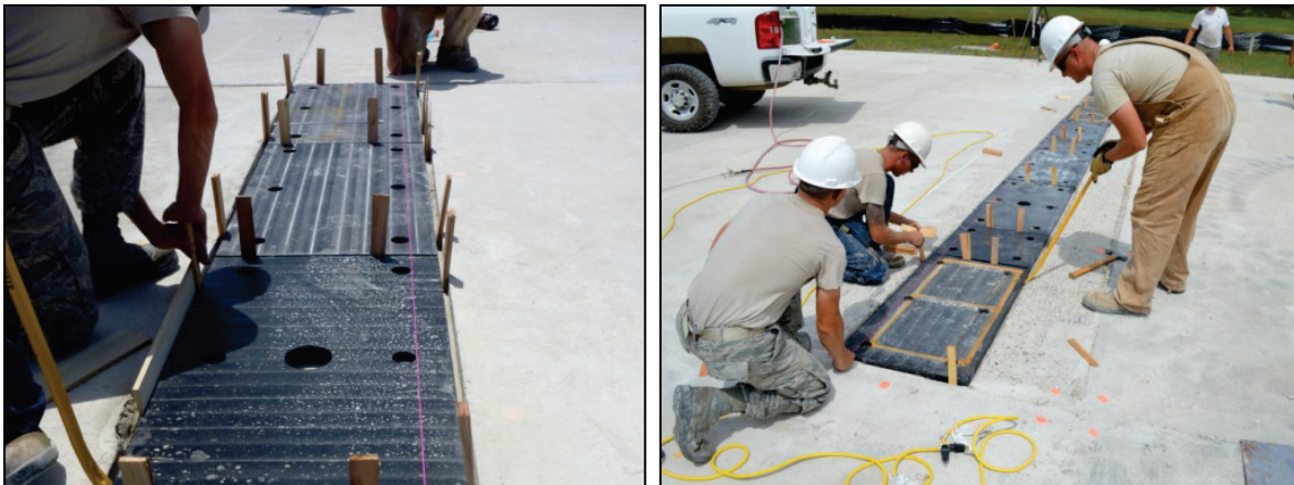
Figure D-2. Shimming panels.
