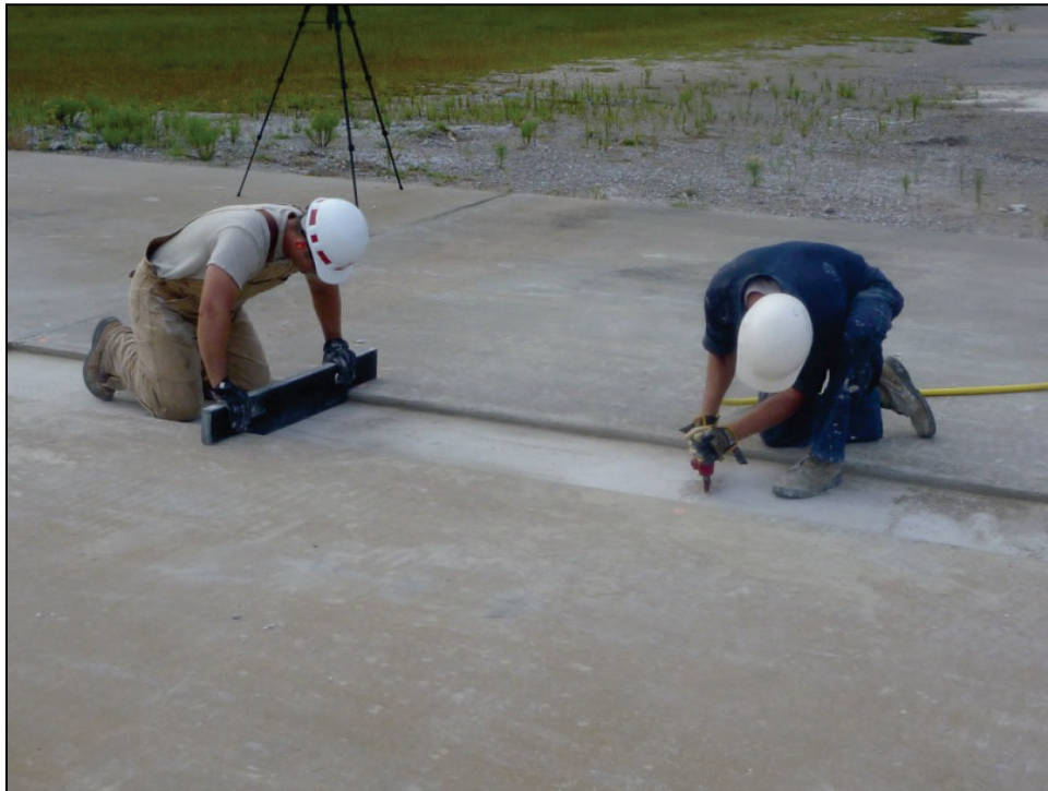
Figure B-15. Final leveling of the panel slot.
