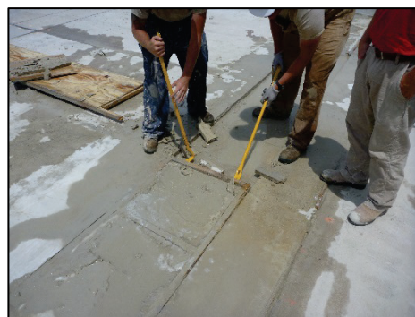
Form destroyed to remove
