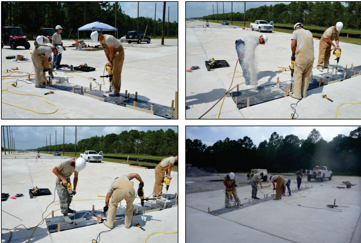
Figure A-21. Anchor hole production line.
