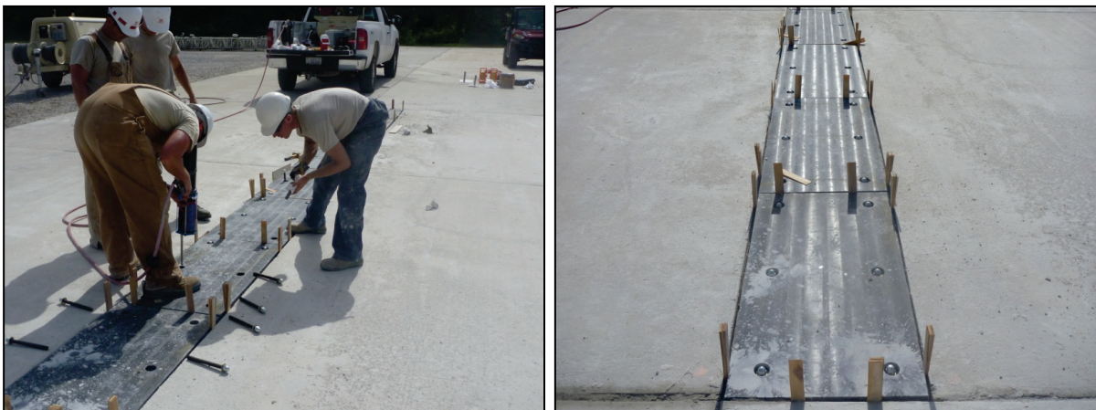
Figure C-27. Anchor installation.
