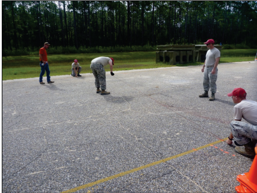
Figure E-3. Snapping chalk lines.
