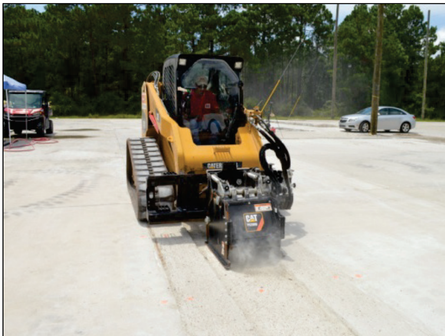
Figure 12. Compact track loader (CTL) milling concrete.
