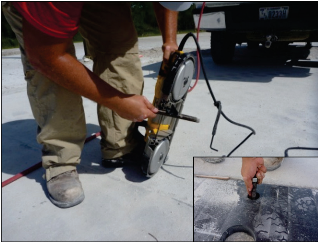
Figure 13. Field modification of panel anchoring rods.
