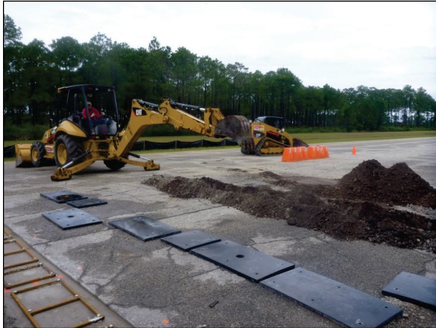
Figure E-28. Pavement surface removal.
