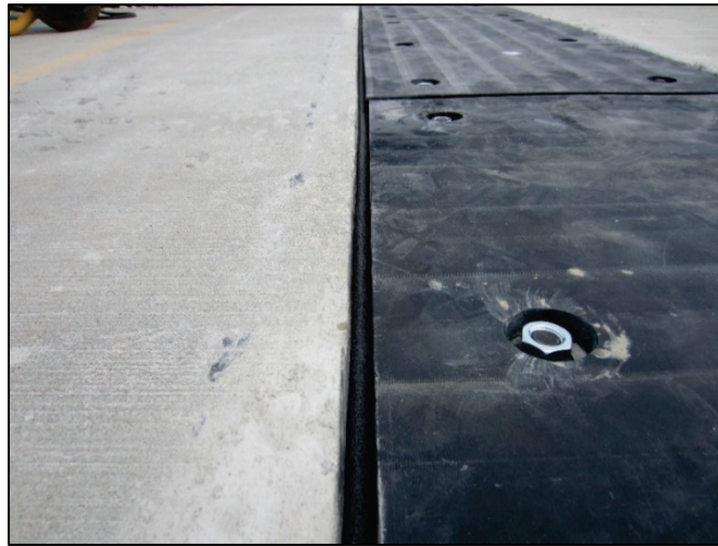
Figure A-30. Backer rod installed.
