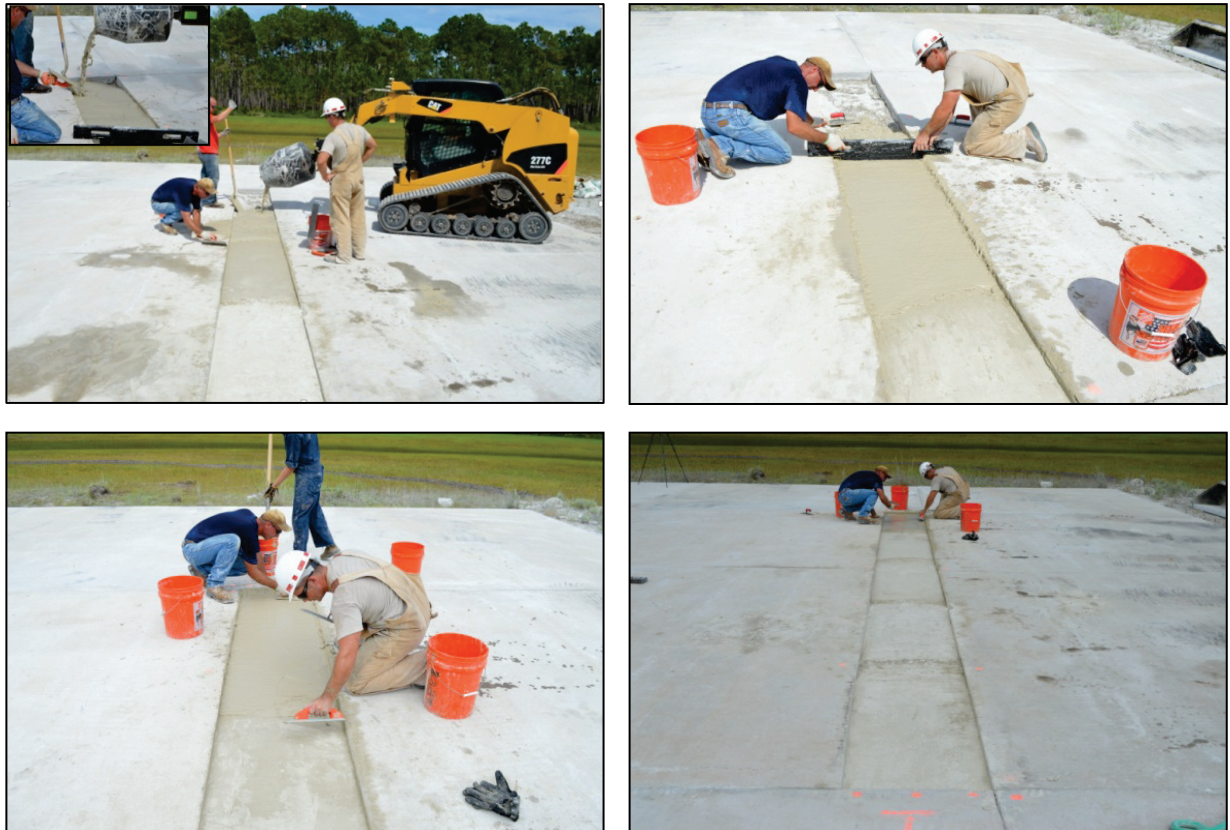
Figure A-14. Placing and finishing the bedding material.
