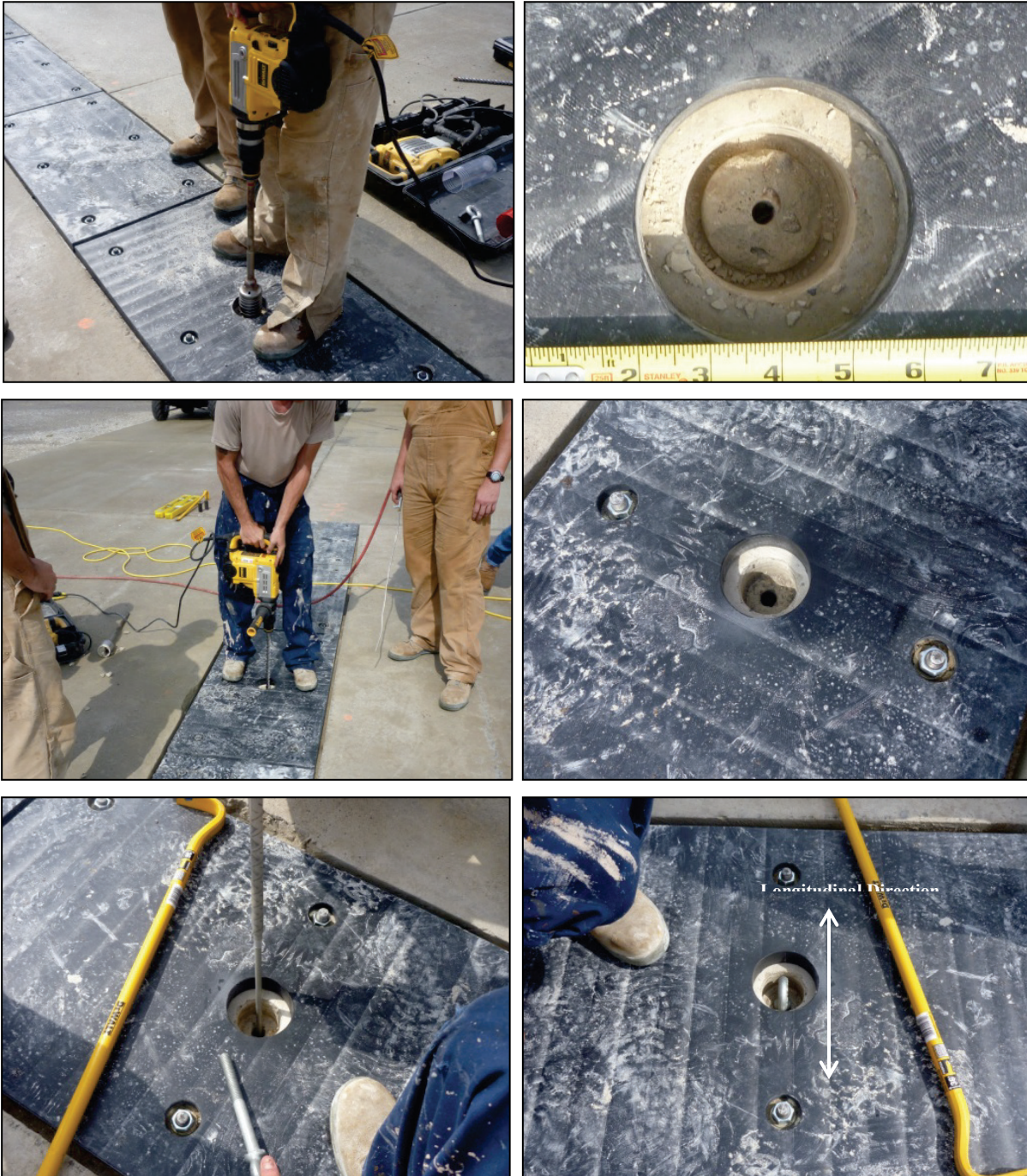
Figure C-28. Tie down anchorage installation.
