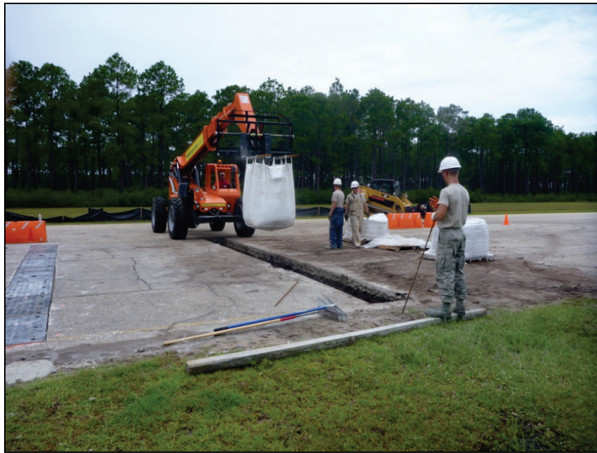
Figure B-9. Placing flowable fill (dry method).
