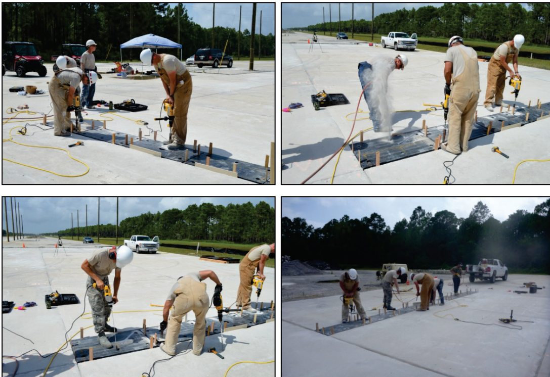
Figure E-21. Anchor hole production line.
