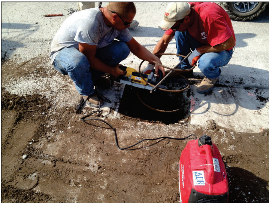
Figure 46. Field modification of tie-down anchoring reinforcement.
