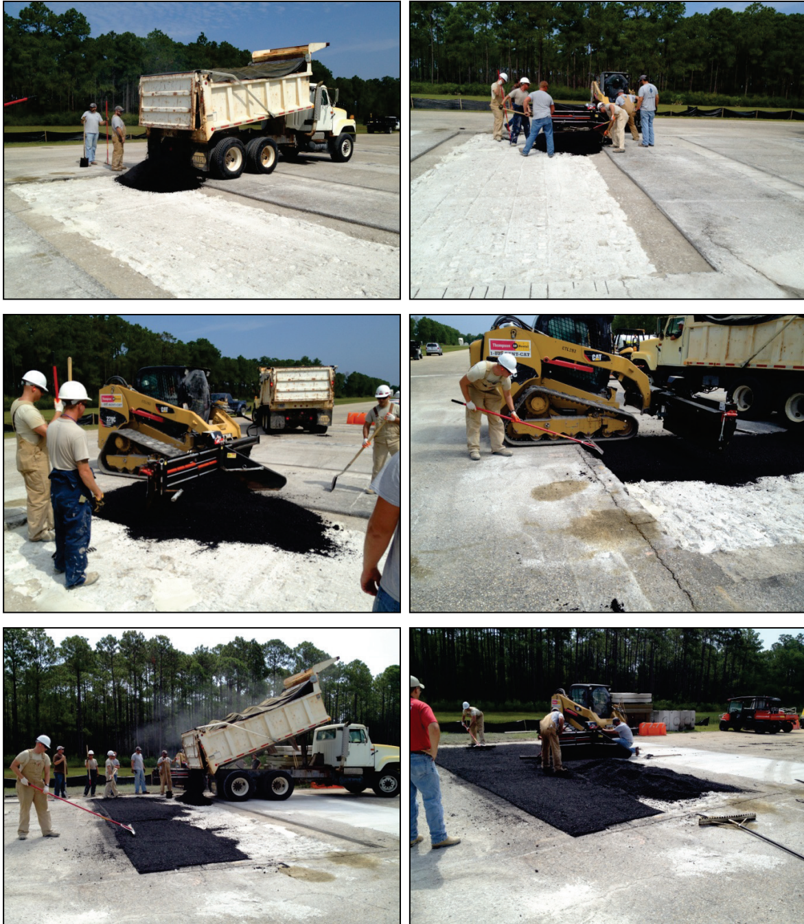
Figure D-16. Asphalt placement.
