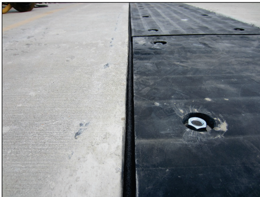
Figure E-44. Backer rod installed.
