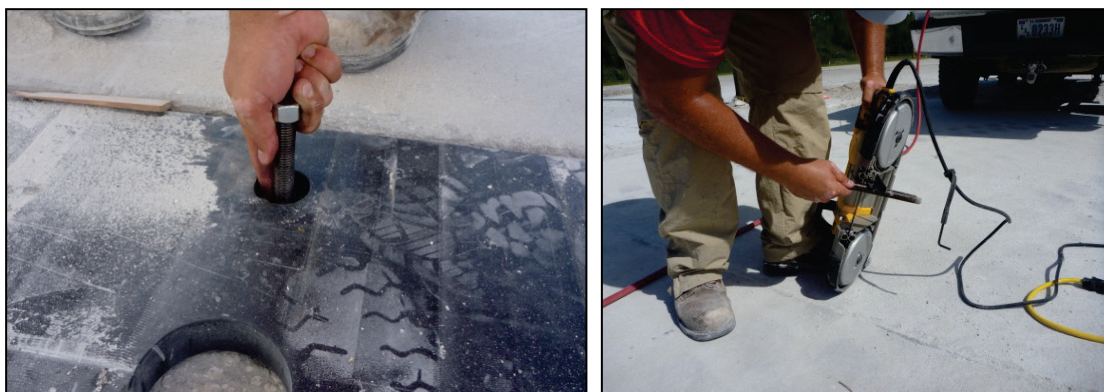
Figure E-23. Trimming a panel anchor.
