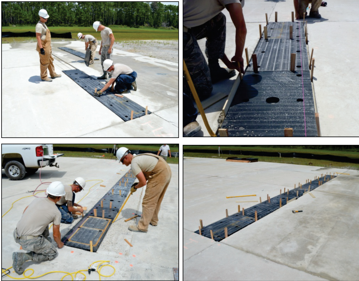
Figure B-17. Aligning panels within the slot.
