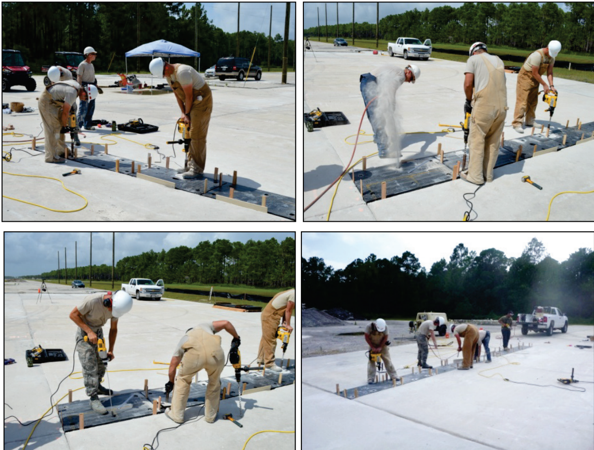
Figure C-26. Anchor hole production line.
