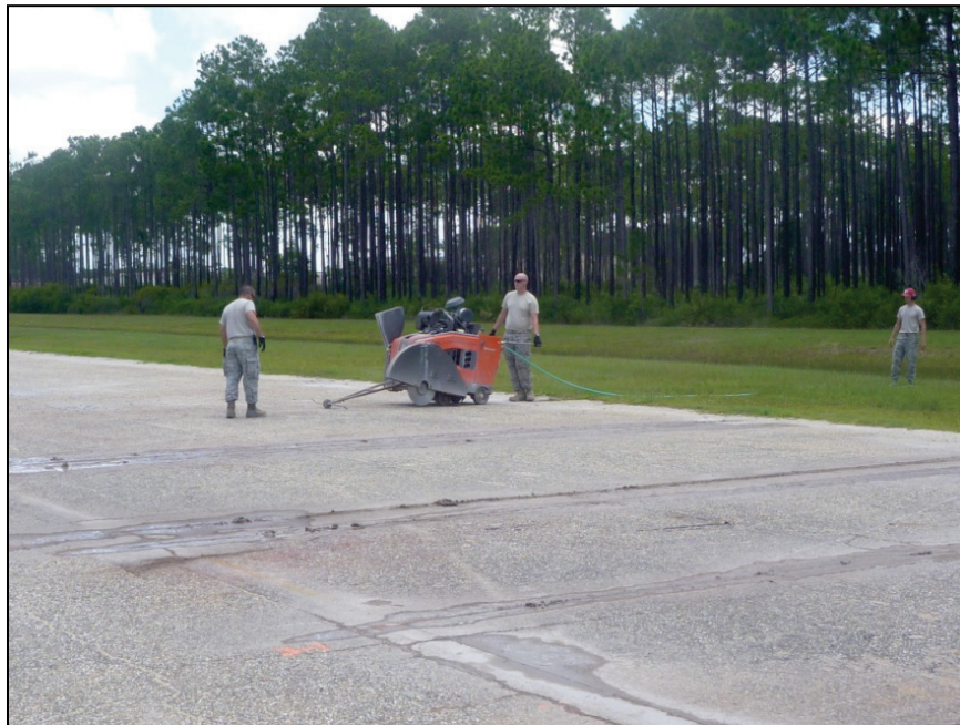
Figure E-4. Transverse cutting on AC areas.
