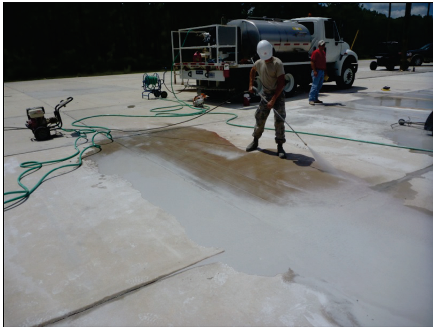
Figure E-7. Waterblasting saw slurry.
