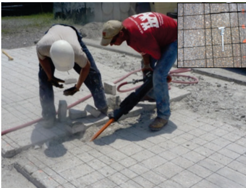
Figure 11. Additional relief cut construction and removal of smaller concrete pieces.
