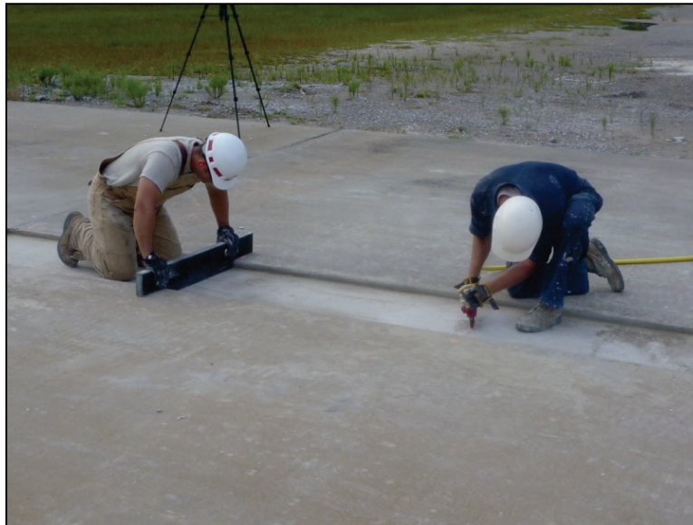
Figure A-18. Final leveling of the panel slot.
