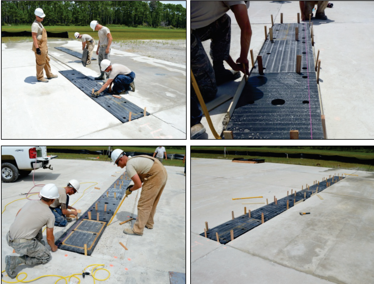
Figure C-25. Aligning panels within the slot.
