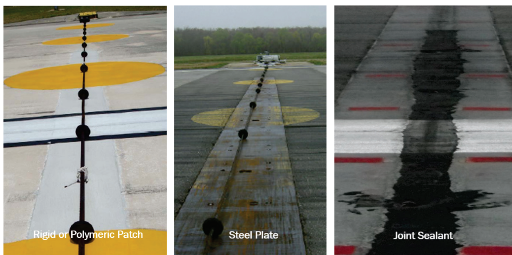
Figure 3. Typical pavement repairs made to correct pendant damage 1 (Rutland 2013).
