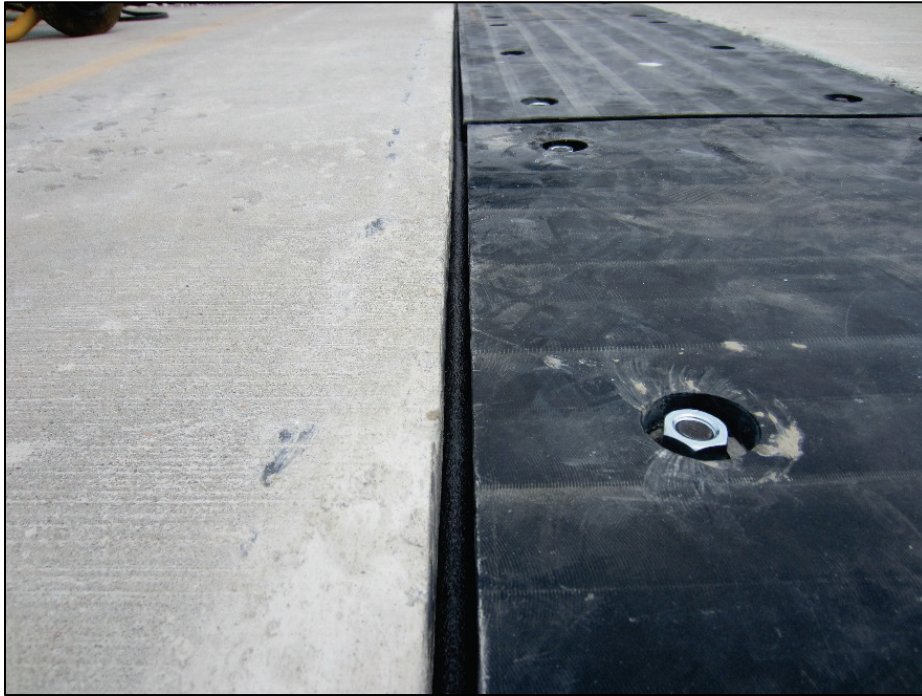
Figure C-31. Backer rod installation.
