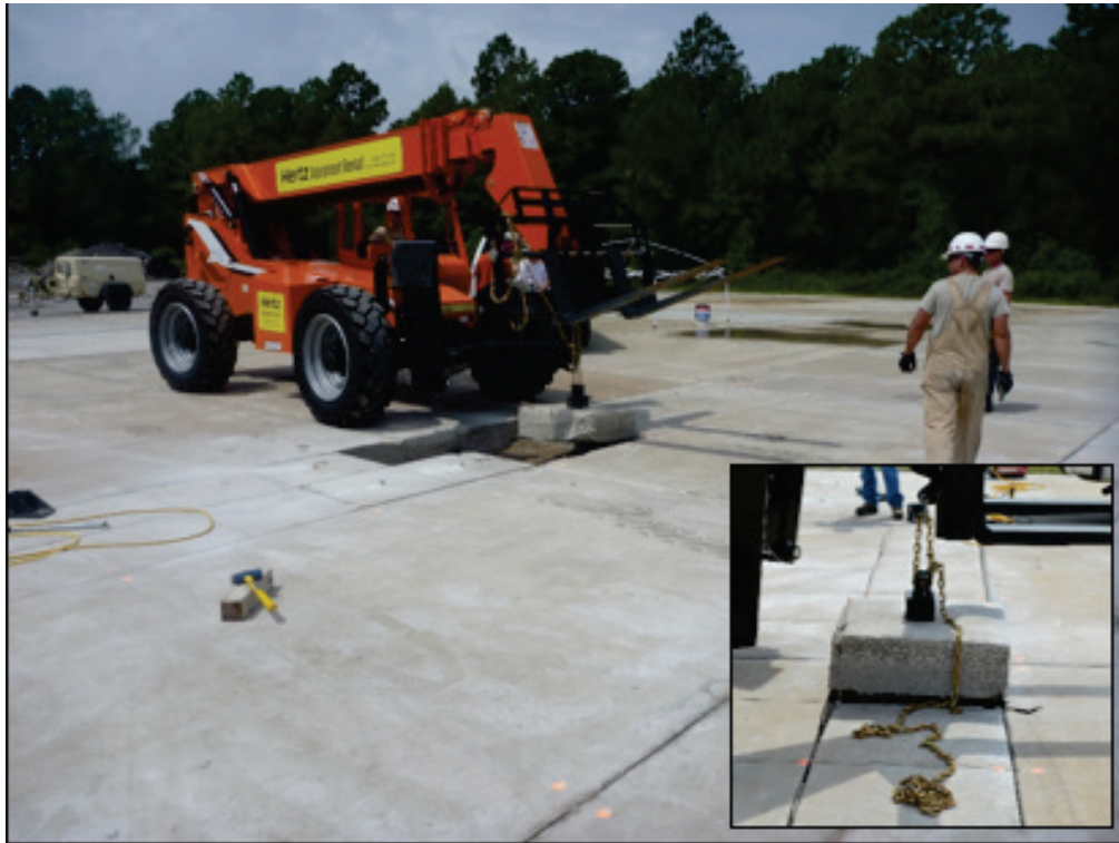
Figure 19. Slab removal by forklift.
