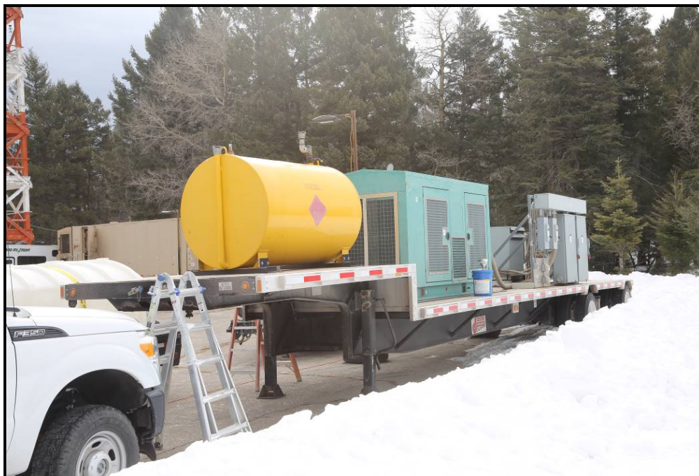
Figure B-5. Generator (350 kilowatt). Displaying fuel tank, generator, and electrical panel.
