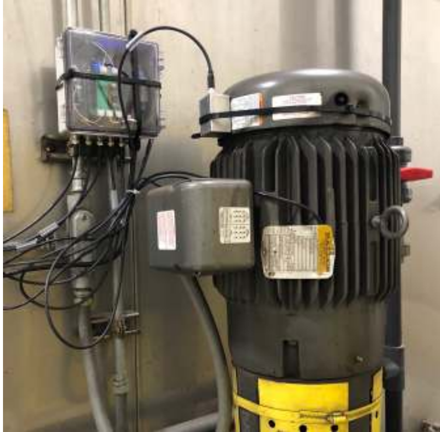
Figure 2. A retrofit kit mounted to a critical motor in the Steelcase factory.
