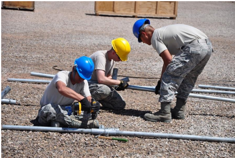
Figure 5.5. Air Force Civil Engineers Assemble an Experimental PV Array.
