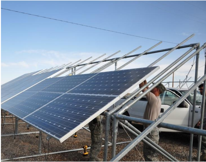
Figure 5.4. Air Force Engineers Assemble an Experimental PV Array at Holloman AFB, NM.
