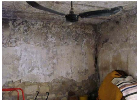
Figure 8-8. Burned interior of Jassim's brother's house 404
