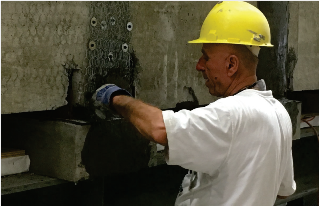
Figure 15. Applying cementitious stucco over the joints between exterior wall panels, and between the panels and a frame footing.
