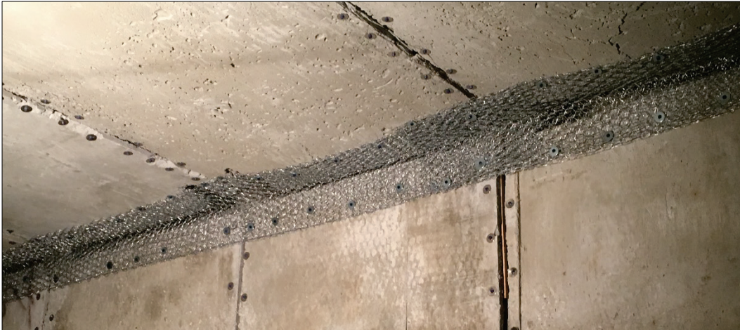
Figure 13. Mat of chicken wire mesh installed over ceiling to interior wall panel joints.
