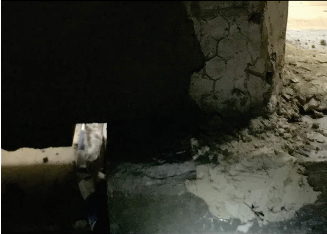
Figure 33. Limited damage to stucco at interior of North door frame column to footing connection, 50% test.
