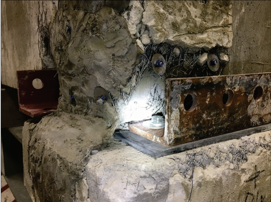
Figure 32. Stucco damage at the northeast column to footing connection, 50% test.
