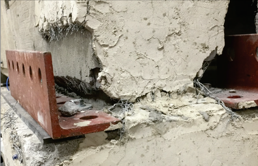
Figure 27. Stucco damage at the southeast column to footing connection, 25% test.
