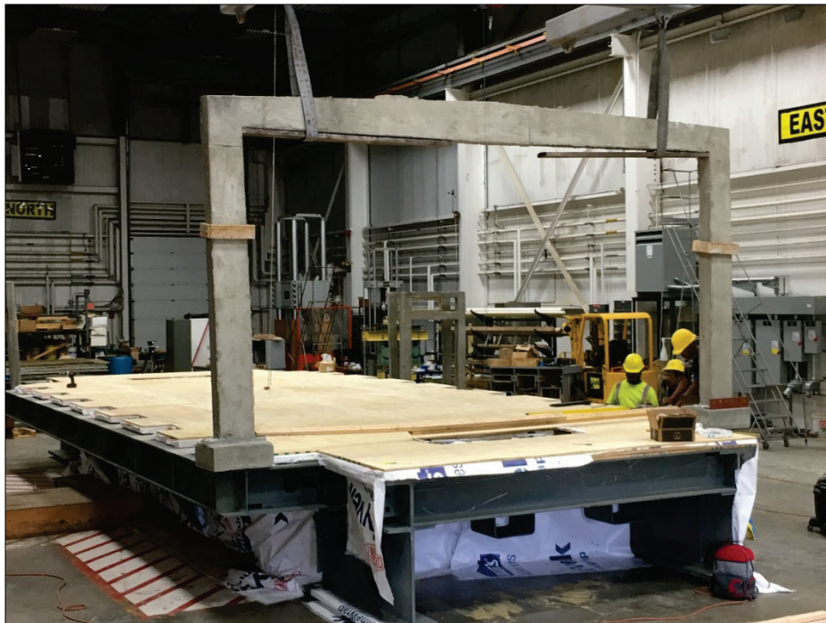
Figure 4. Test fixture with completed wood deck and house wrap, as the first frame is being installed.
