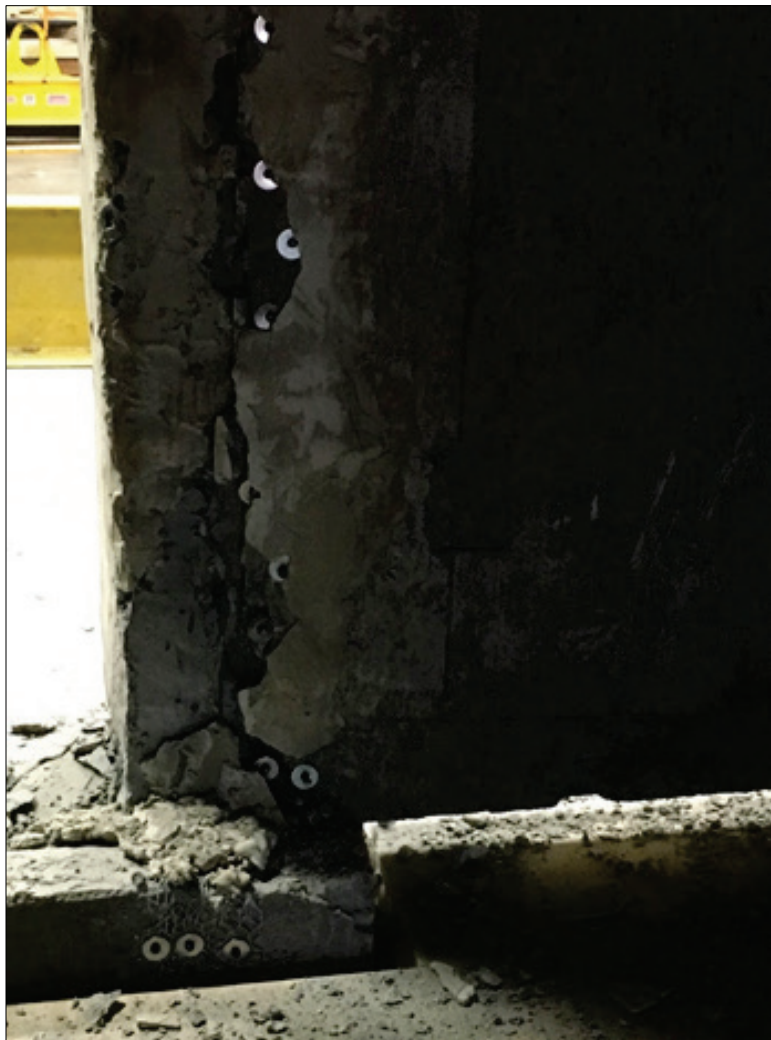
Figure 45. Interior view of North door frame column shows cracks in stucco and wall panel, 100% test.
