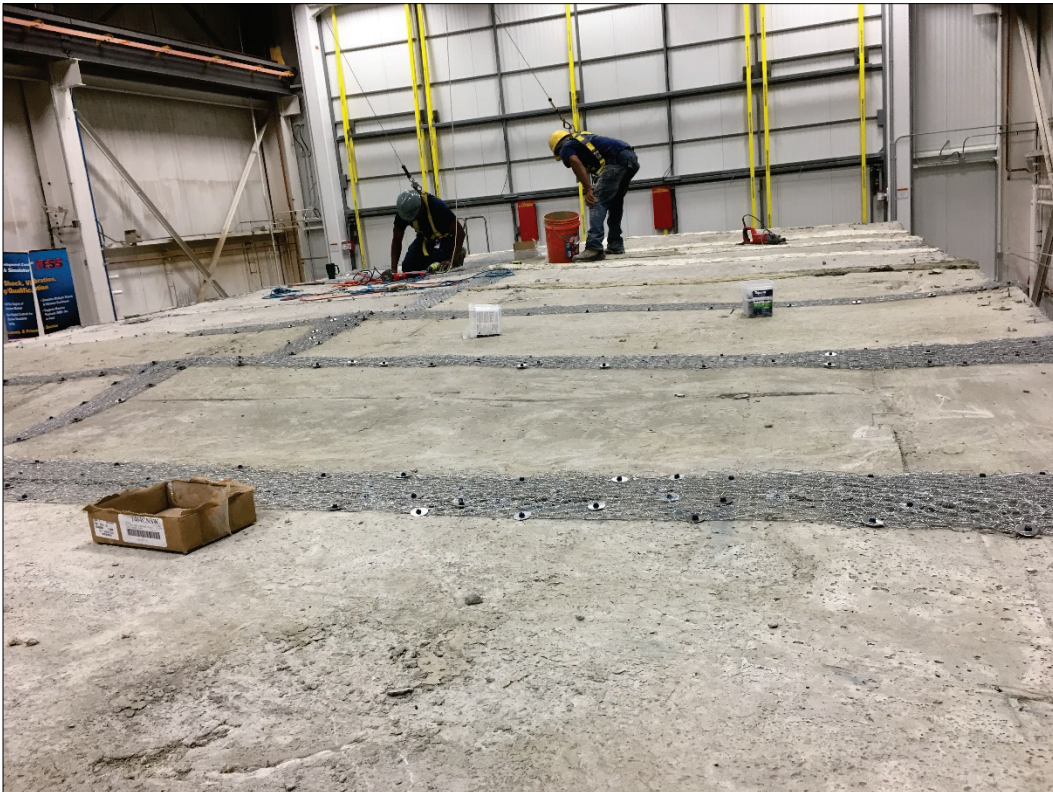
Figure 16. Applying stucco over roof panel joints. (Note the mesh in the foreground.)
