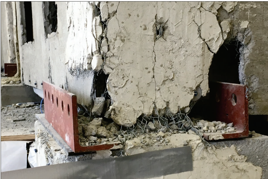
Figure 36. Bottom of column at Southeast corner showing concrete rubble and partly fracture chicken mesh, 100% test.
