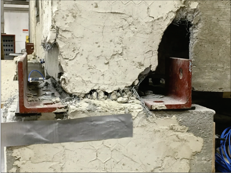
Figure 31. Stucco damage at the southeast column to footing connection, 50% test.
