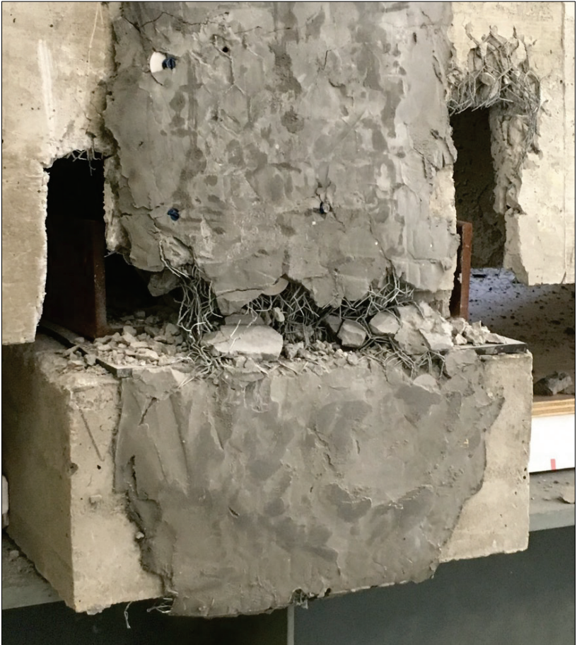
Figure 38. Bottom column at the west face, 100% test.
