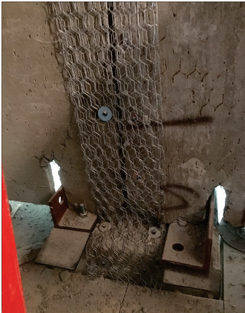
Figure 14. Chicken wire mesh installed over joint between interior wall panels, and between interior wall panels and frame footings.
