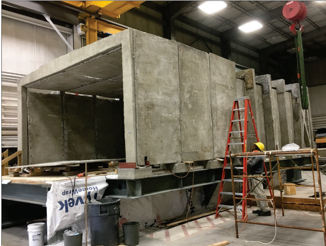
Figure 8. Exterior wall panels being installed.
