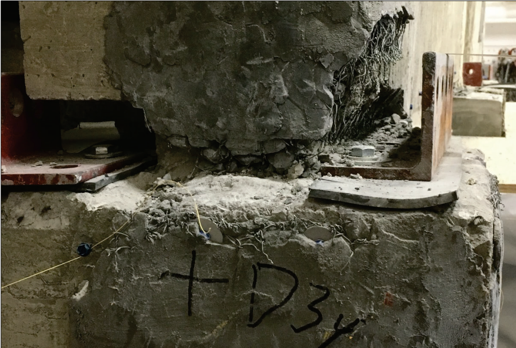
Figure 28. Stucco damage at the southwest column to footing connection, 25% test.
