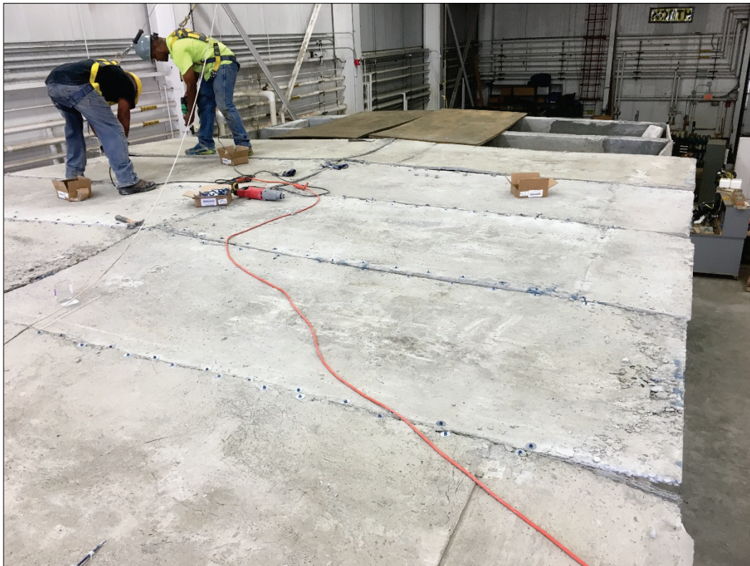
Figure 11. Roof panels being installed.
