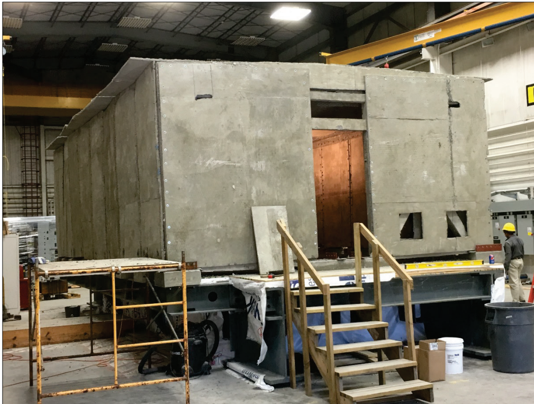
Figure 12. Indigenous building after roof panel installation showing the roof eaves.
