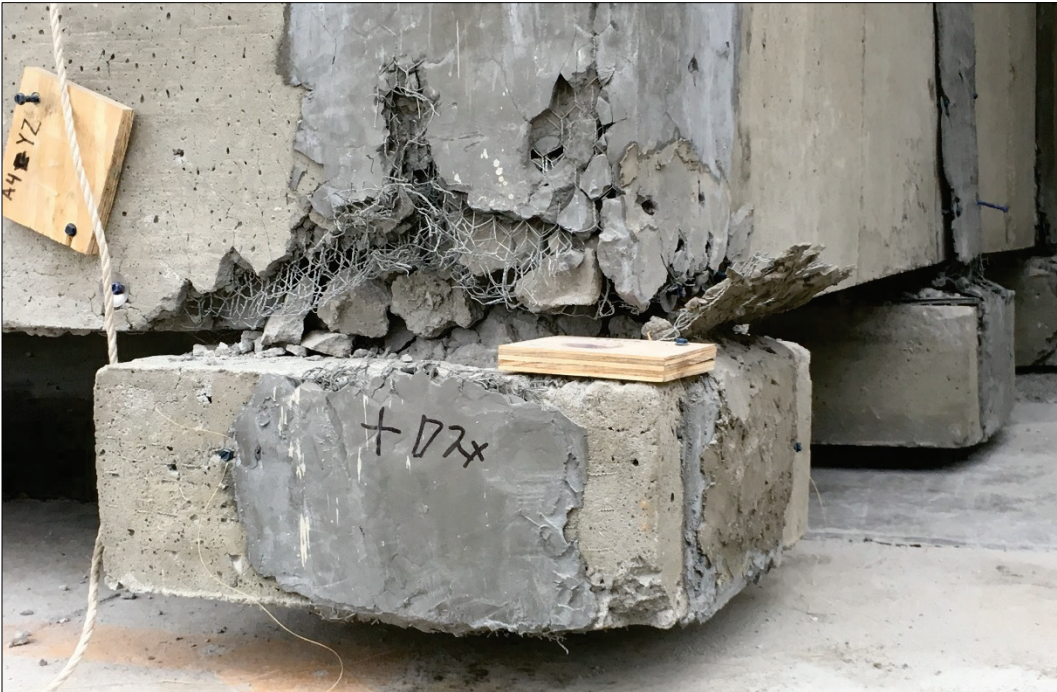
Figure 42. Bottom of northwest column, after removing the building from the test fixture, 100% test.
