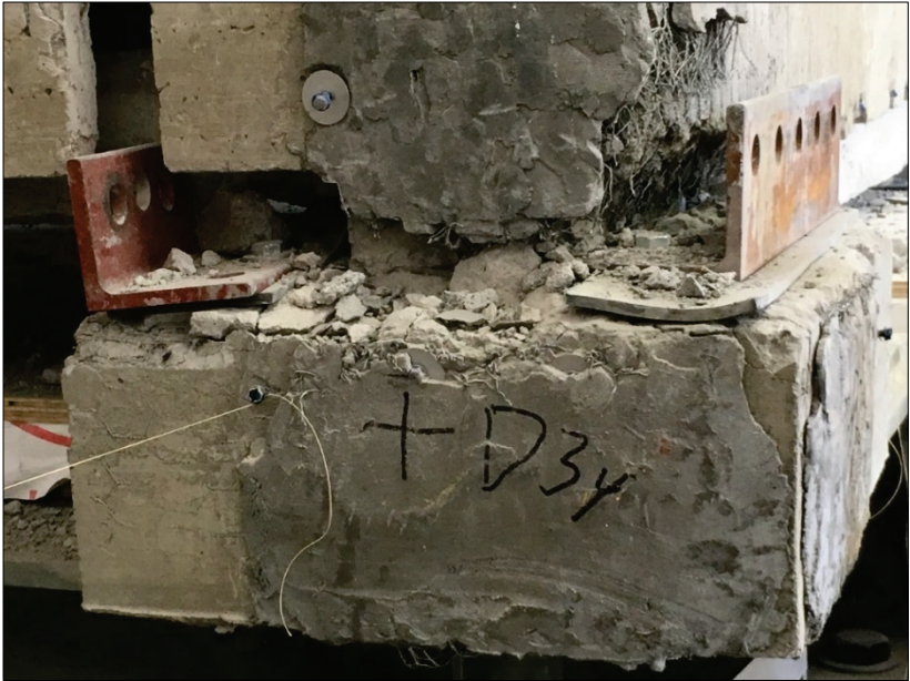
Figure 37. Bottom column at southwest corner, 100% test.
