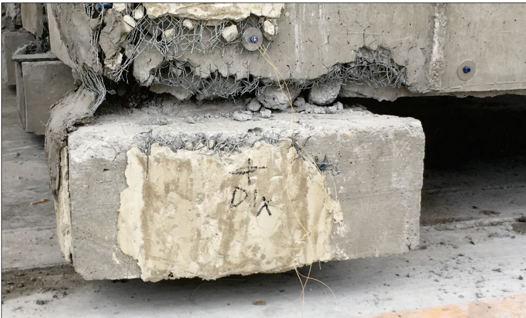
Figure 40. Bottom of northeast column, after removing the building from the test fixture, 100% test.
