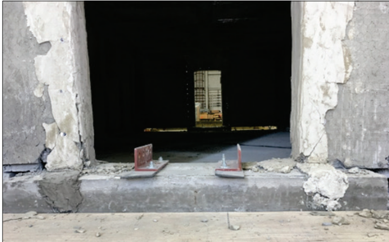
Figure 44. Bottom of south wall door frame columns with large cracks, 100% test.
