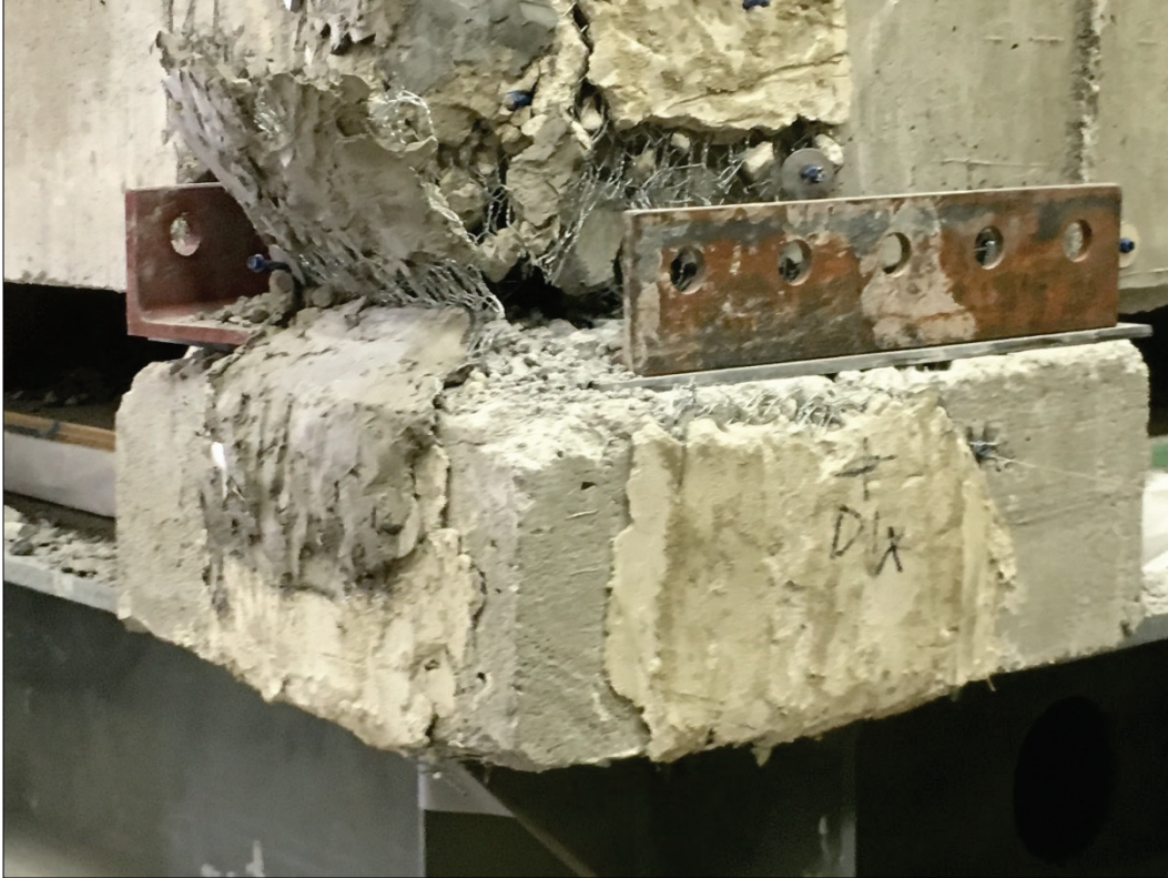
Figure 39. Bottom of northeast column, 100% test.
