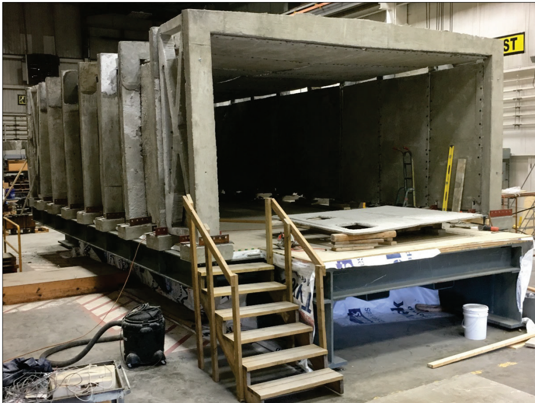
Figure 6. Indigenous building with frames, ceiling and interior wall panels installed.
