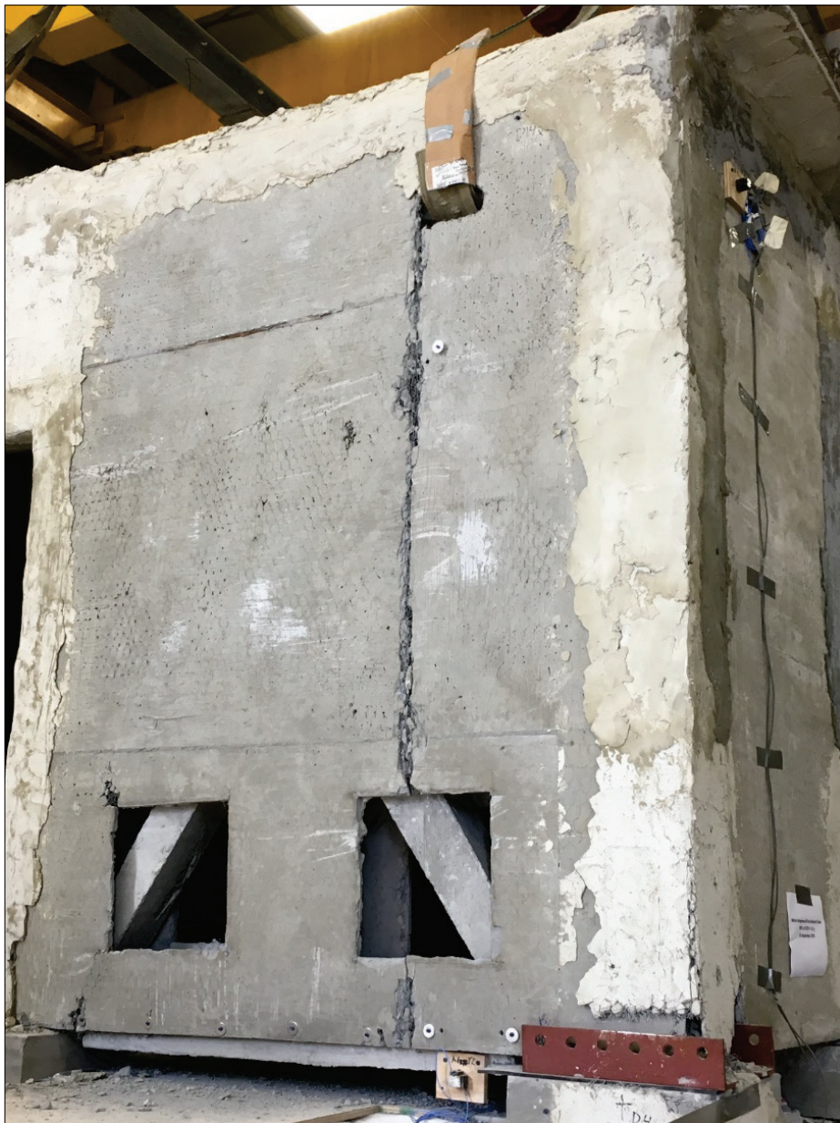
Figure 43. East side of south short wall, where brace and wall panel connections partly failed at the bottom left corner of picture – note the vertical crack in the wall panel, 100% test.
