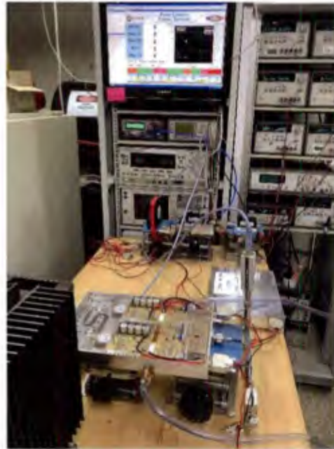
Figure 96. Experimental setup for measuring Individually tested output powers of 2 kW SSPA modules
