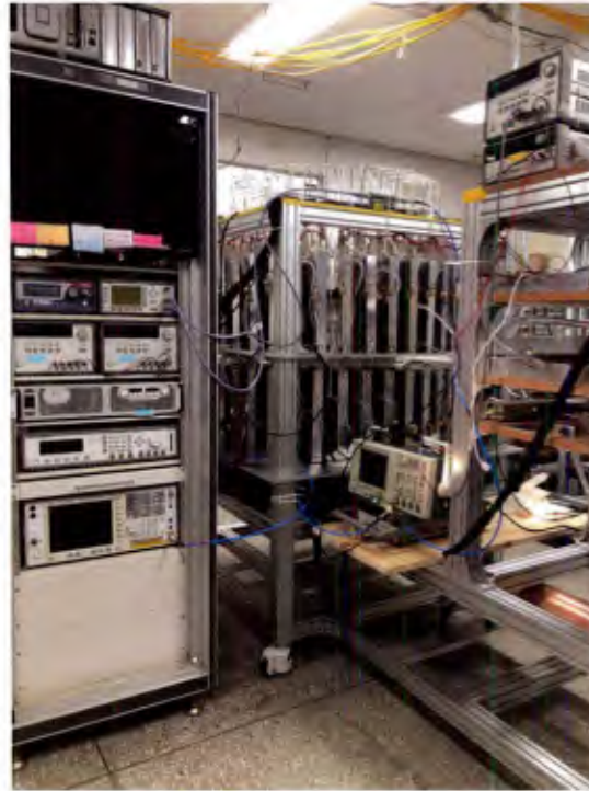
Figure 120. Photo of 80-way power combiner system operating at high duty cycle
