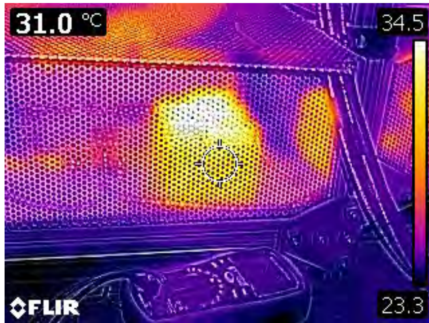
Figure 12. Capacity sensor controller under operation.
