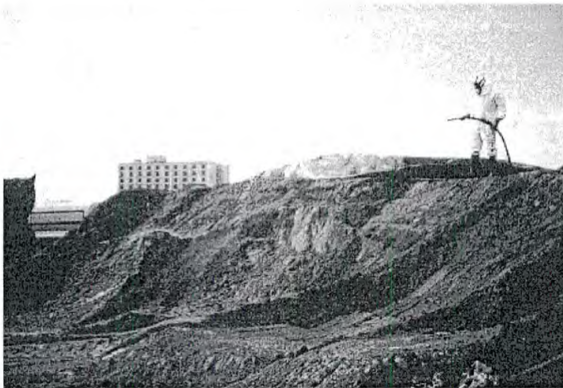
Photo 3-1. Wetting down the grit pile during screening operations to control fugitive emissions, protecting human health and the environment.
