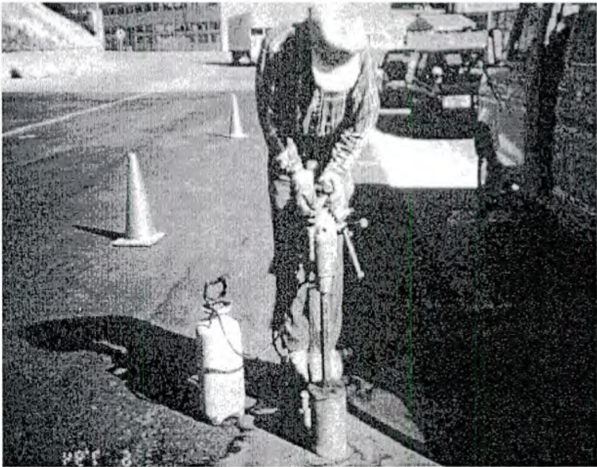
Photo 6-2. Core sampling of an asphalt test strip.
