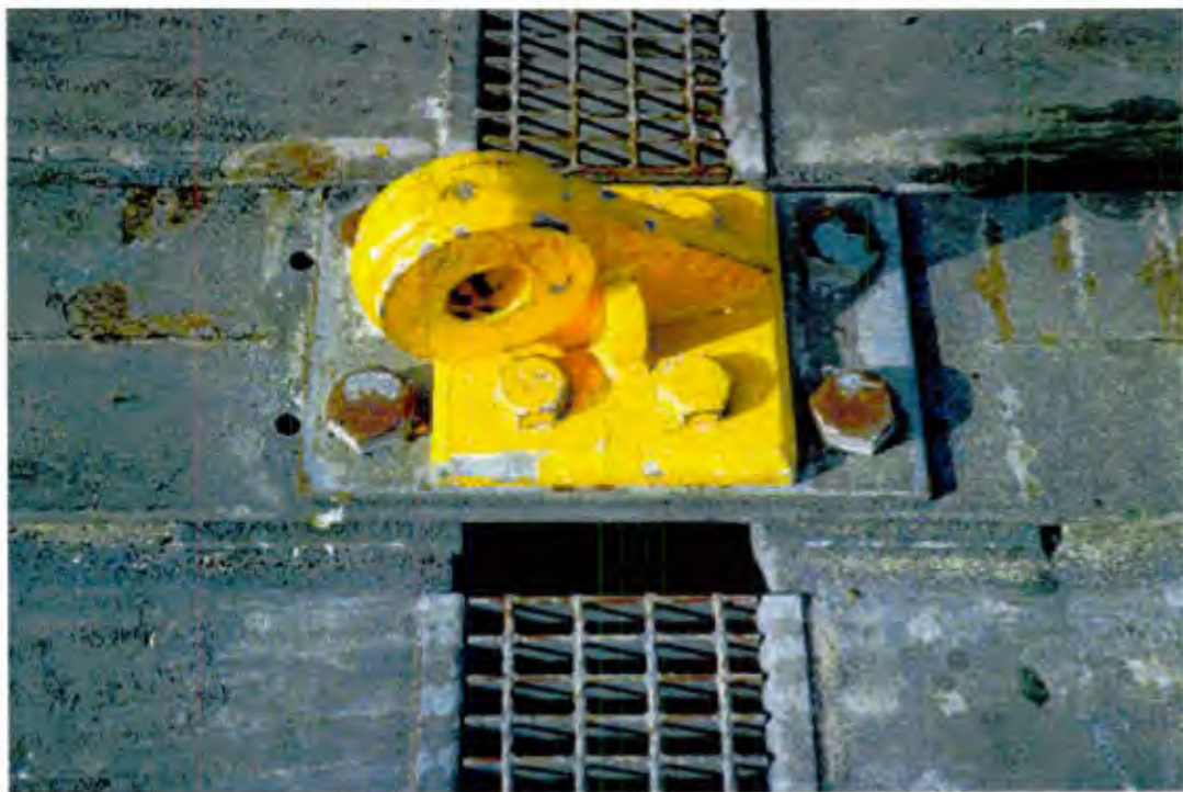
Figure 17 PH-11 padeye bolted to double angle.
