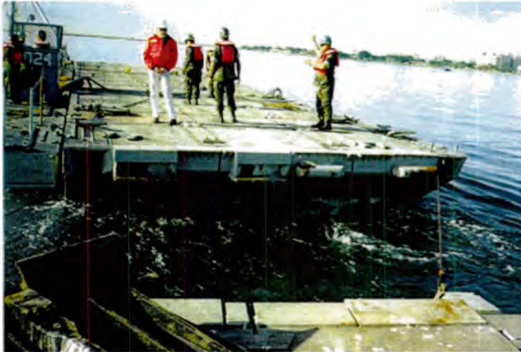
Figure 12 Misalignment of sections during bridle inhaul.
