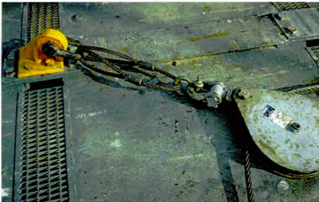
Figure 11 PH-11 padeye rigged to place 18-inch snatch block on the centerline of the causeway.
