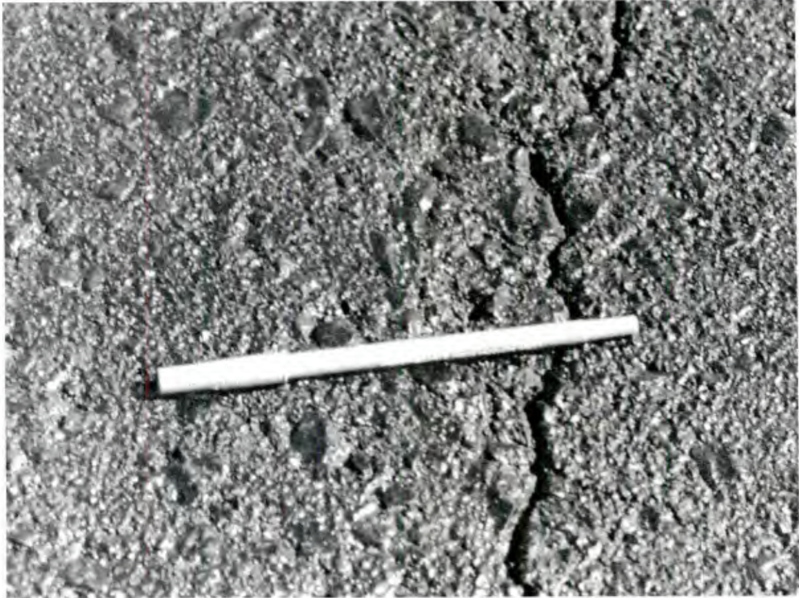
FIGURE 8. TYPICAL PAVEMENT DEFECTS (CRACKING AND RAVELING OF LOW SEVERITY) AT NEEDLES AIRPORT, NEEDLES, CALIFORNIA.
