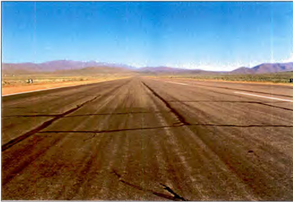
Figure 16. Low temperature thermal cracked AC pavement, Runway 14, Reno-Stead Airport.
