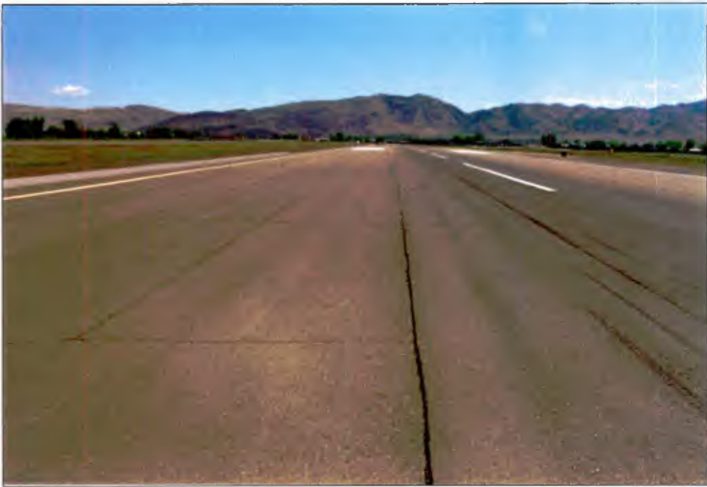
Figure 14. Low temperature thermal cracked asphalt pavement, Reno International Airport.
