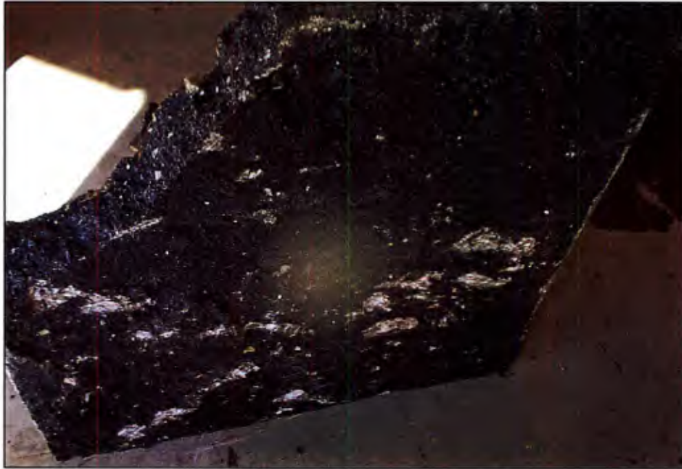
Figure 3. Bottom of surface layer after being removed from intermediate layer 2.
