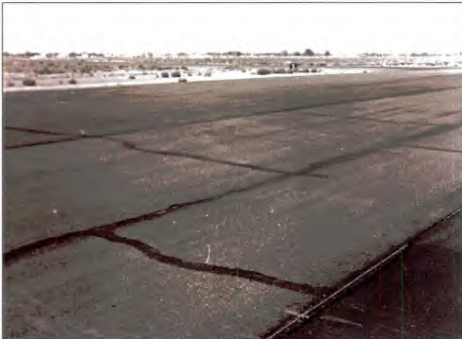
Figure 2. NAS Fallon Runway R13-31, existing cracks and new overlay (lower right) (26 August 1986).
