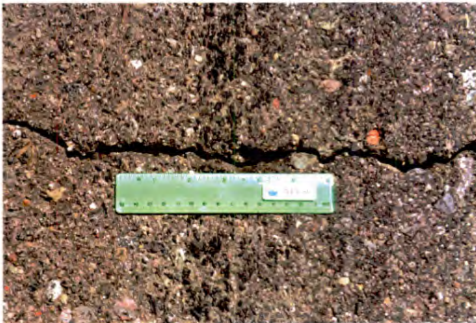
Figure 15. Low temperature induced thermal crack in AC, Reno International Airport.
