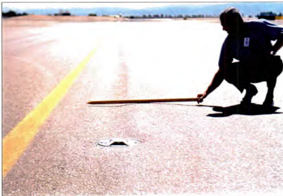
Figure 11. Rutting of asphalt pavement taxiway at McCarran International Airport.
