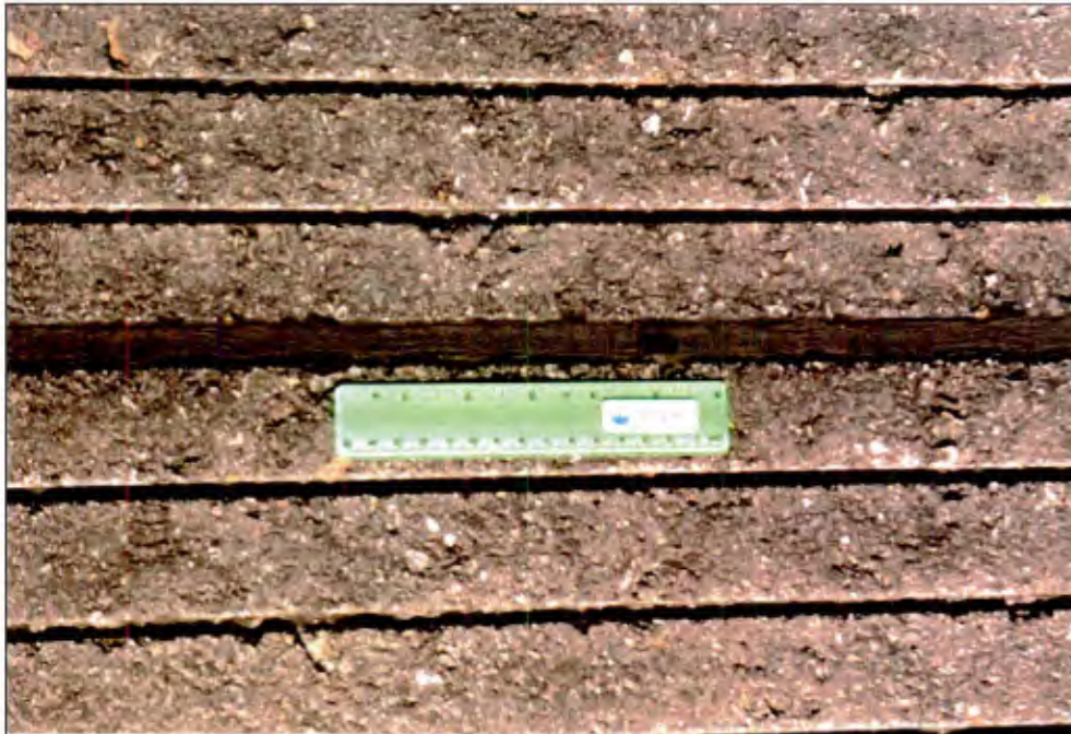
Figure 19. Saw-cut joint (sealed) and grooved AC pavement, Runway 8-26, Reno-Stead Airport.
