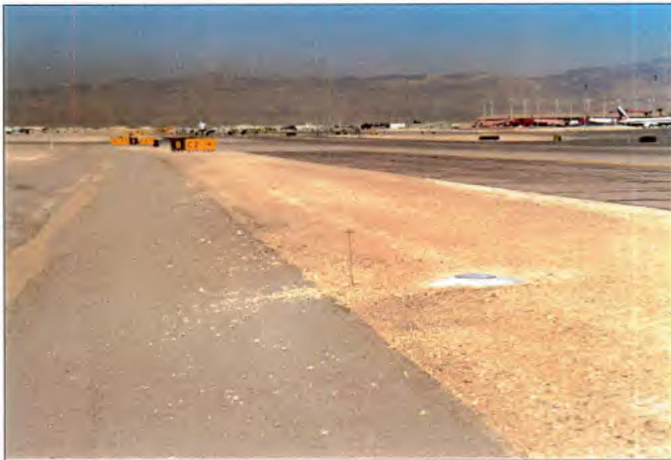
Figure 10. Asphalt drainage ditch constructed in 1992 at McCarran International Airport.
