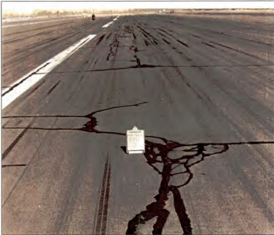
Figure 1. NAS Fallon Runway R13-31, crack sealed (1970).
