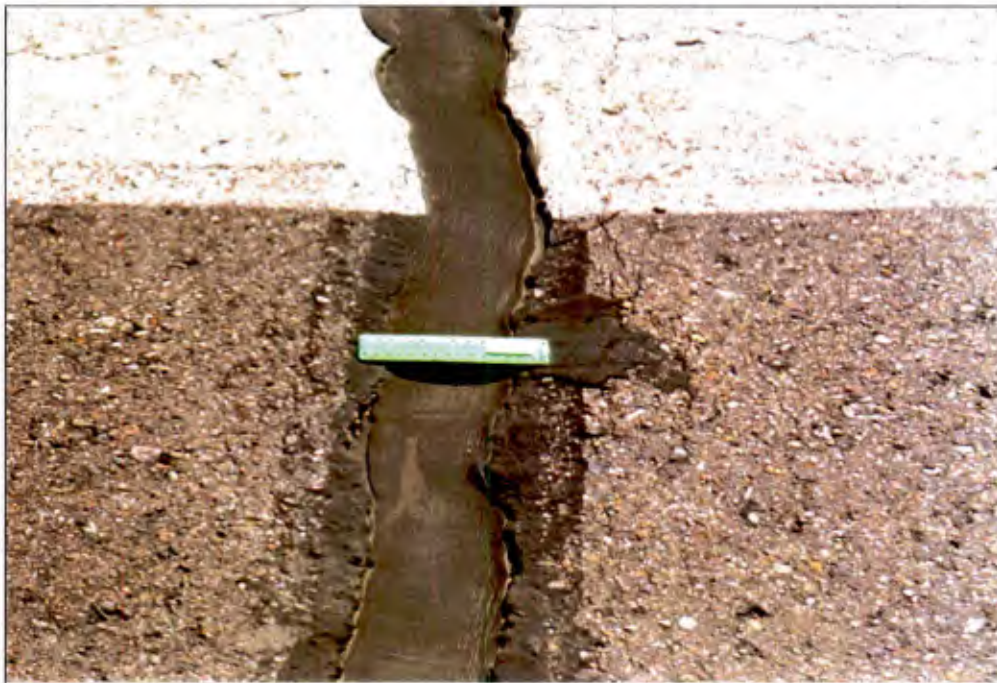
Figure 17. Sealed thermal crack in AC pavement, Runway 14-32, Reno-Stead Airport.
