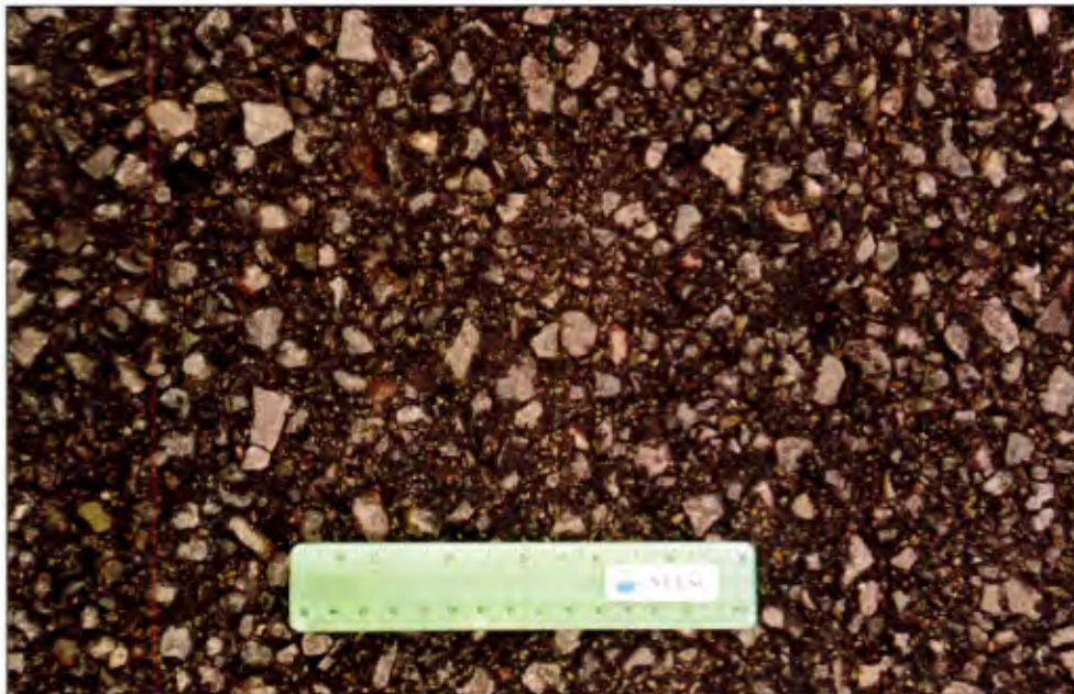
Figure 6. NAS Fallon Runway 13R-31L, close-up of surface with exposed aggregate due to stripping or asphalt deficiency.
