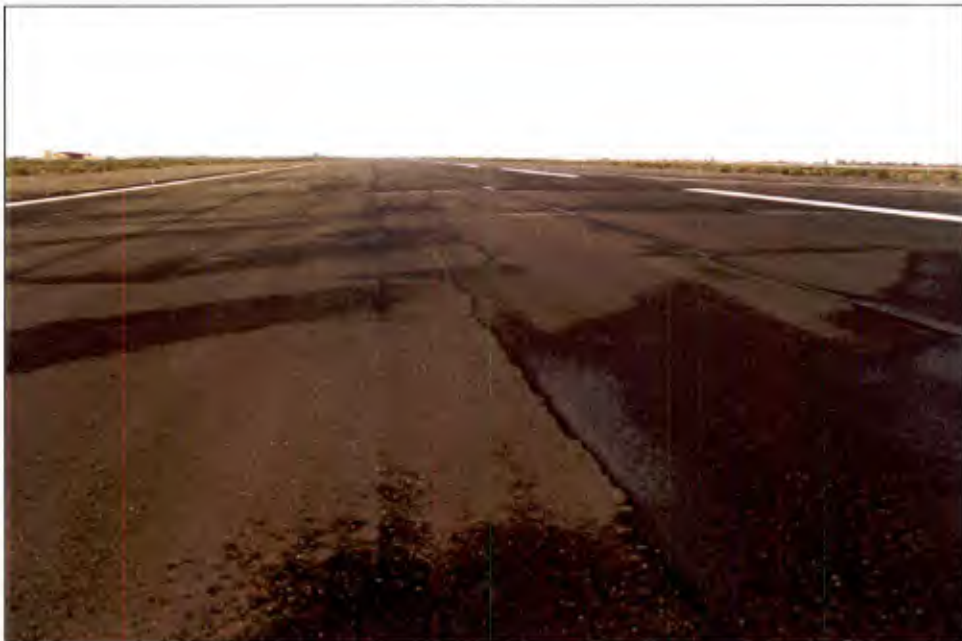
Figure 4. NAS Fallon Runway 13R-31L, cracking pattern in present overlay (22 April 1999).
