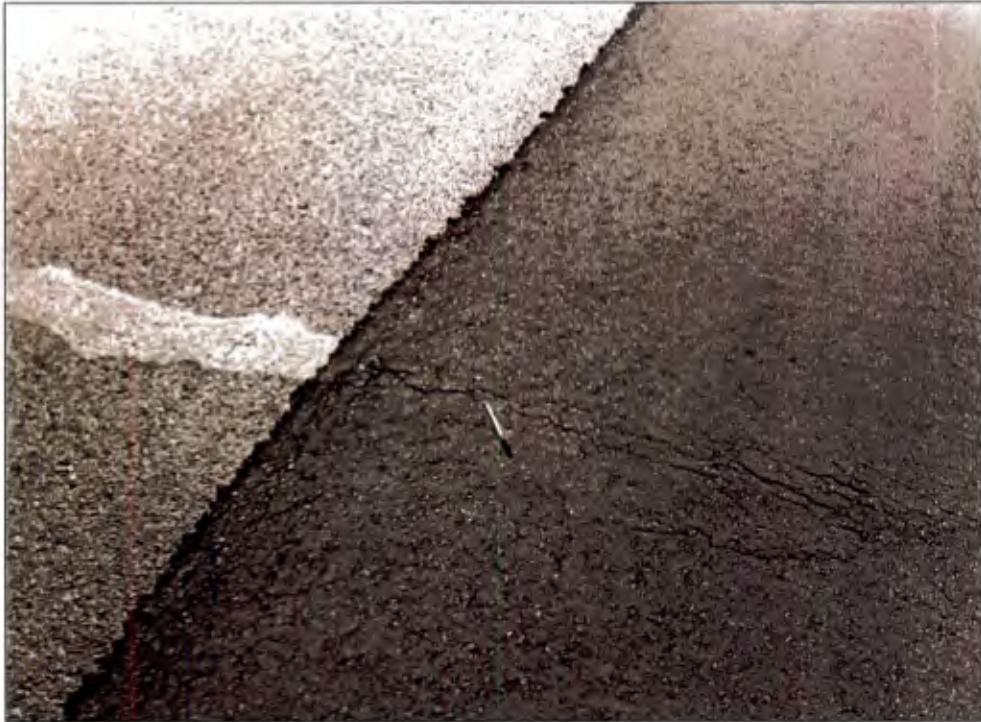
Figure 3. NAS Fallon Runway R13-31, existing cracks with sealant and cracking in new overlay (26 August 1986).
