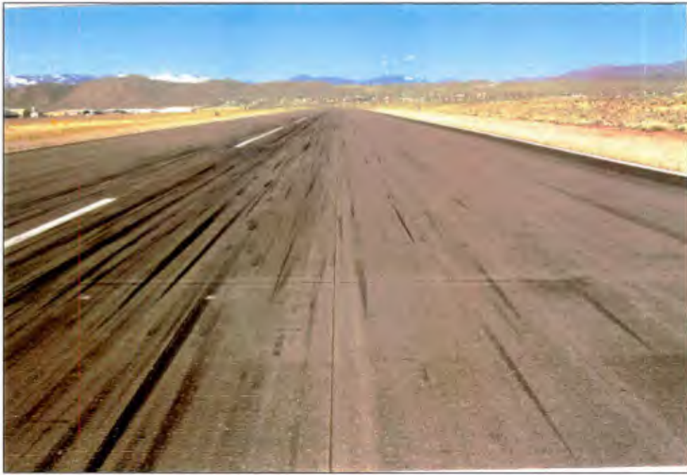
Figure 18. Saw-cut and grooved AC pavement, Runway 8-26, Reno-Stead Airport.
