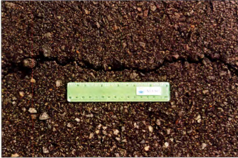
Figure 5. NAS Fallon Runway 13R-31L, close-up of typical crack (22 April 1999).
