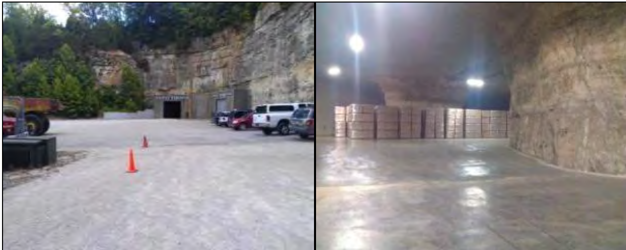
Figure 61. Marengo Warehouse entrance (left) and one of the internal storage chambers (right)
