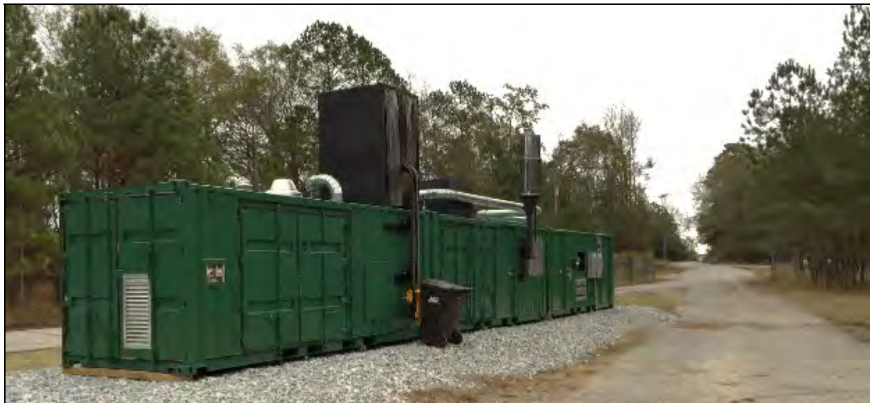
Figure 33: Photograph of the BWEC system during demonstration at Ft. Benning
