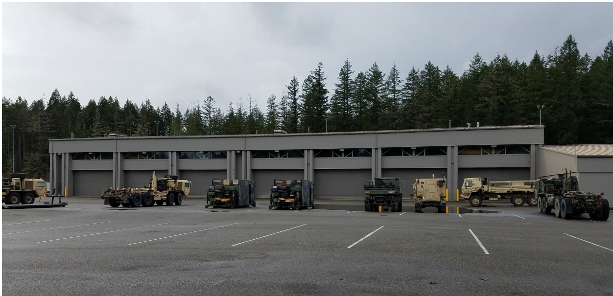
Figure ES-6. Building 3 - Motor Pool Maintenance Facility
