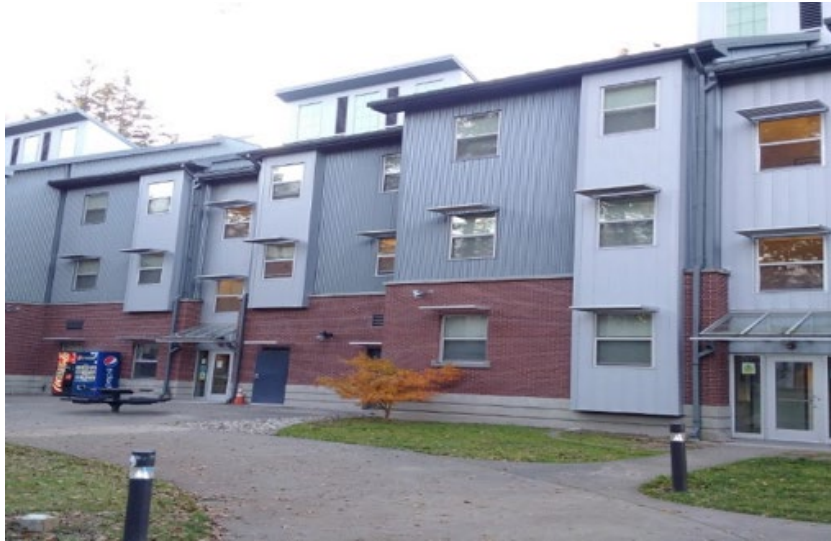
Figure ES-5. Building 2 - Barracks
