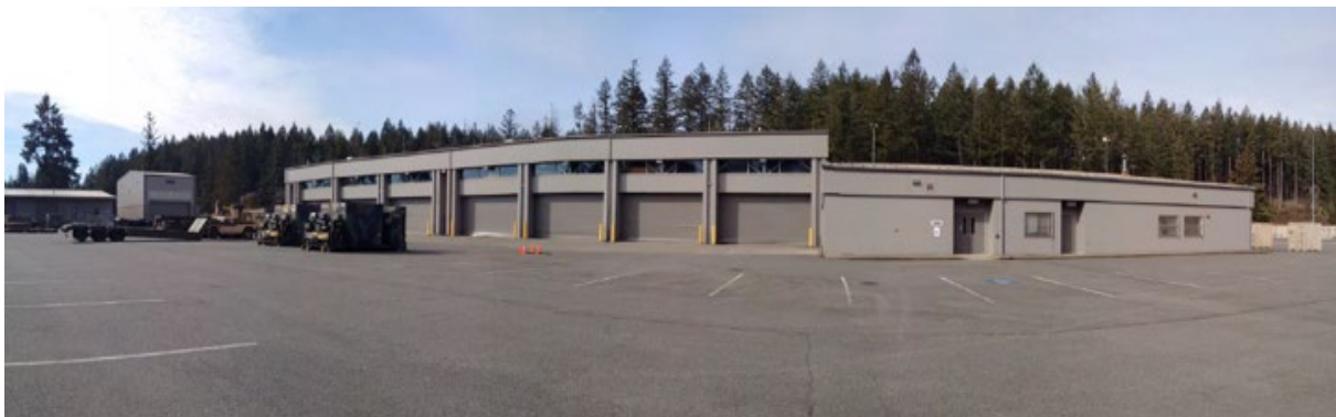
Figure 5-19. Building 3, with Sliding Doors on Left Opening into the Repair Bays, and an Office Area to the Right Side
