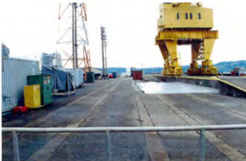
Figure 1. North pier of the Marginal Wharf looking south.
