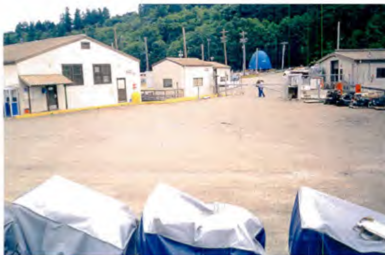
Figure 3. Marginal Wharf approach.
