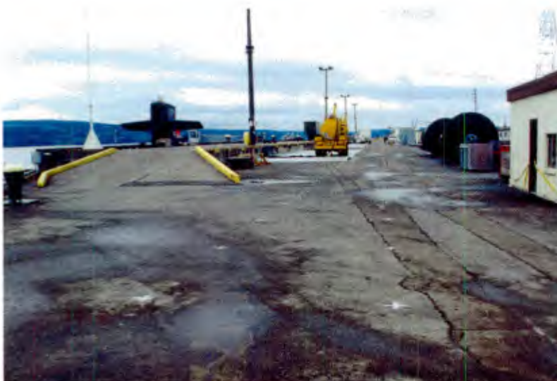
Figure 2. South pier of the Marginal Wharf looking North.
