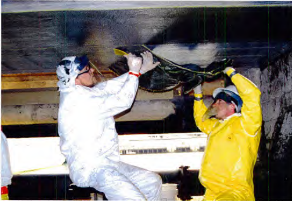
Figure 53. Applying uniaxial carbon fiber sheet to underside of pier deck.
