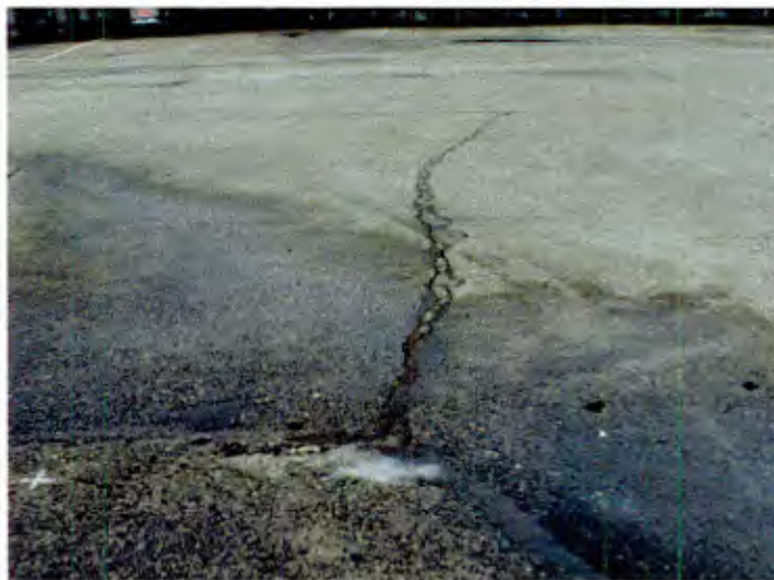
Figure 8. Crack emanating from approach addition (in the foreground) between bents 68 and 69.
