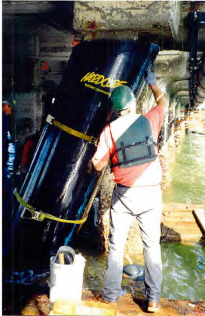
Figure 54. Placing cylindrical composite shell around rectangular concrete pile.
