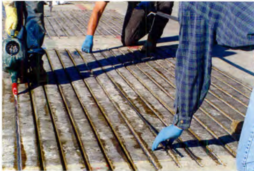
Figure 51. Embedding carbon reinforcing rods in pier deck.
