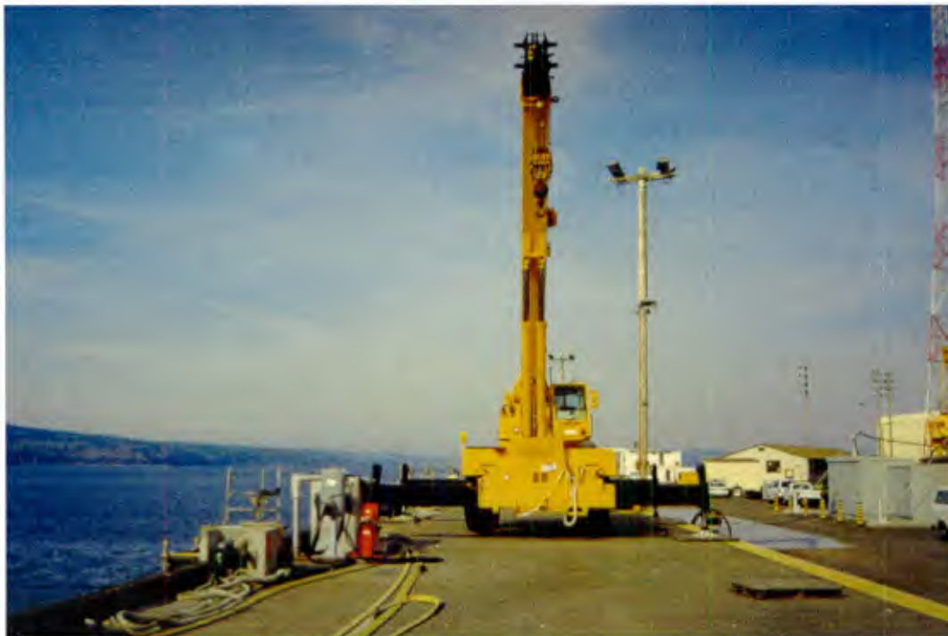
Figure 7. Truck crane on the south platform of the Marginal Wharf.
