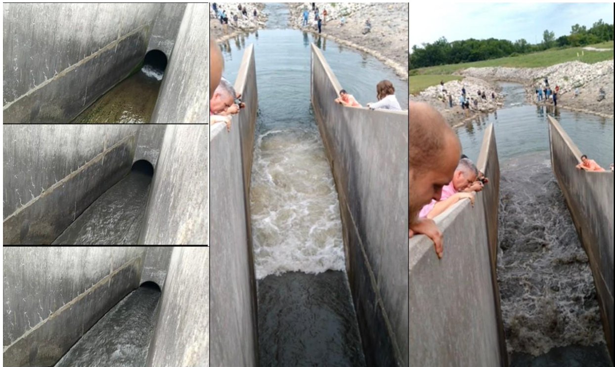
Figure 4. Silt flush at Blue Springs Lake, Missouri.
