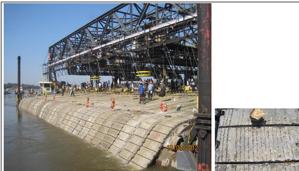
Figure 1. Mat Sinking Unit operating on the Mississippi River; inset of ACM grooves.
