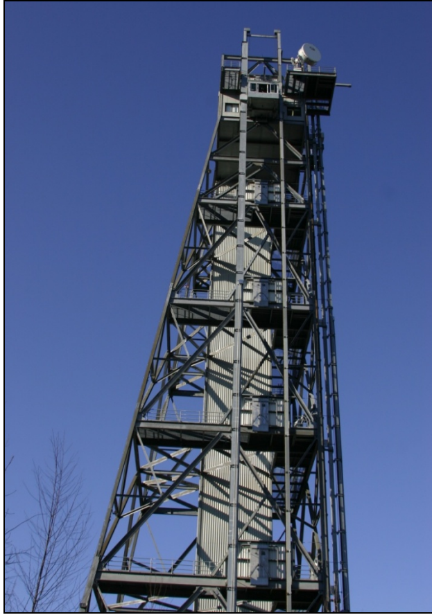
Figure 2. Precision Armaments Laboratory tower with elevator that housed the polarimetric sensor situated on the sixth floor.
