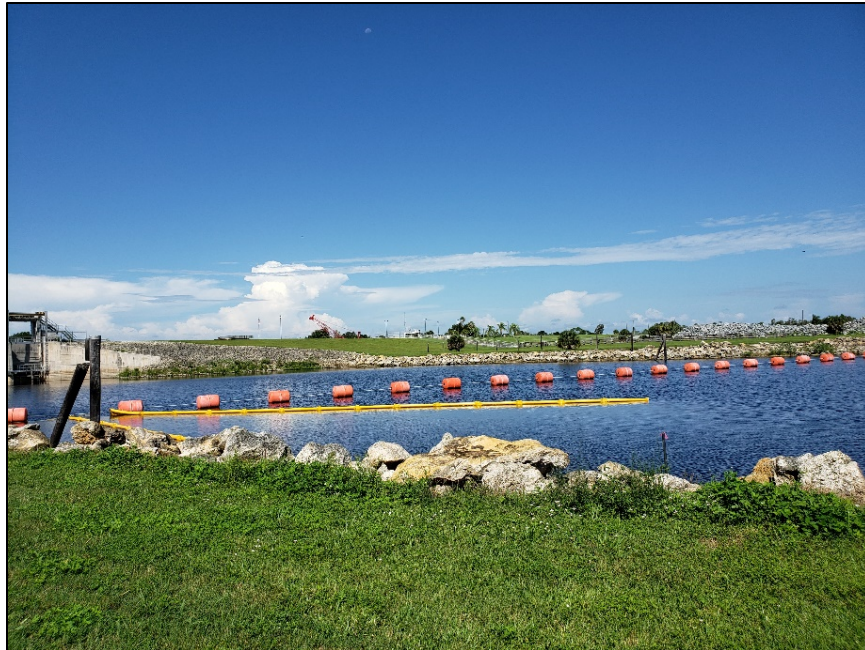
Figure A-1. Boom weir near canal lock and dam.
