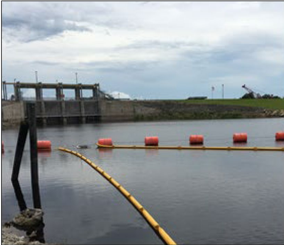
Figure 2-8. Booms and floating weir skimmer set upstream of the Moore Haven spillway.
