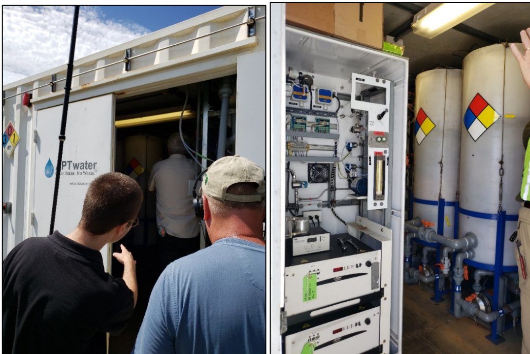
Figure A-15. Water treatment module where clarified water is oxidized to remove toxins from the solution.
