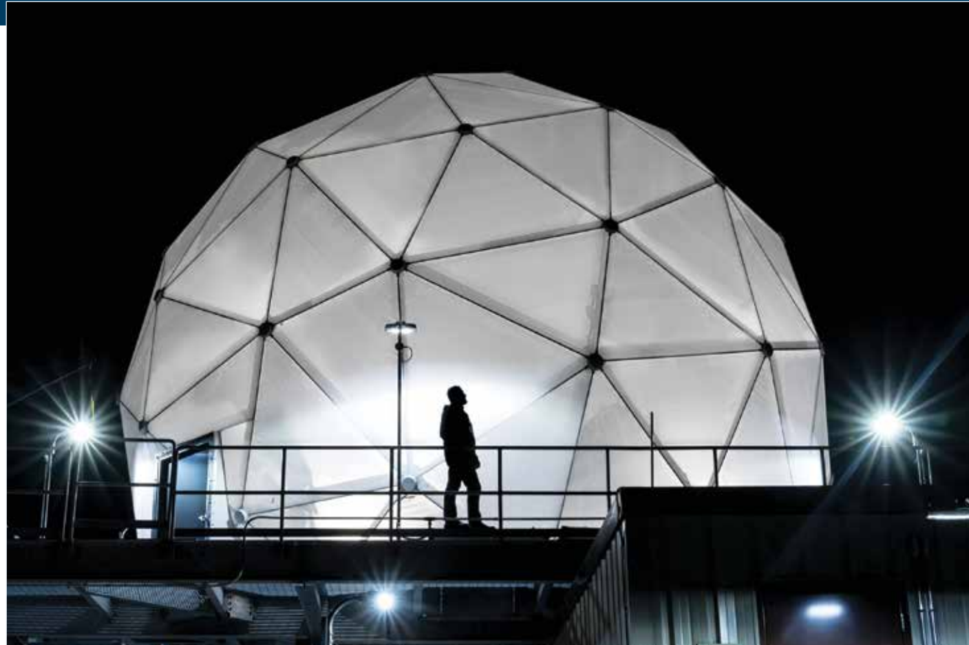
The 6.3-meter Multi-band Test Terminal installed on a roof at Lincoln Laboratory operates in the Ku, Ka, X, and EHF frequency bands. This Air Force-funded antenna enables the testing and evaluation of waveforms and techniques that may increase antijam protection for satellite communications.
