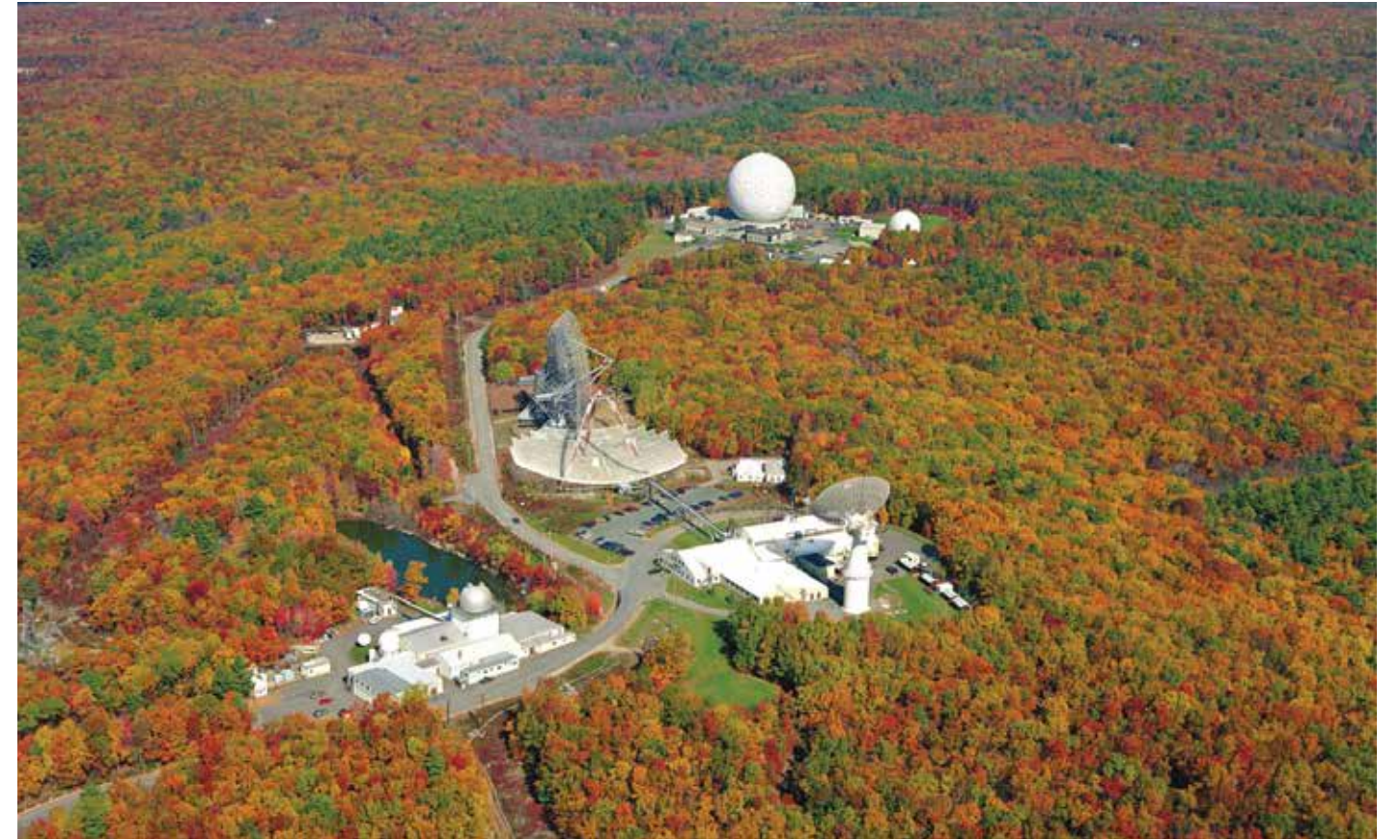
Lincoln Space Surveillance Complex, Westford, Massachusetts
