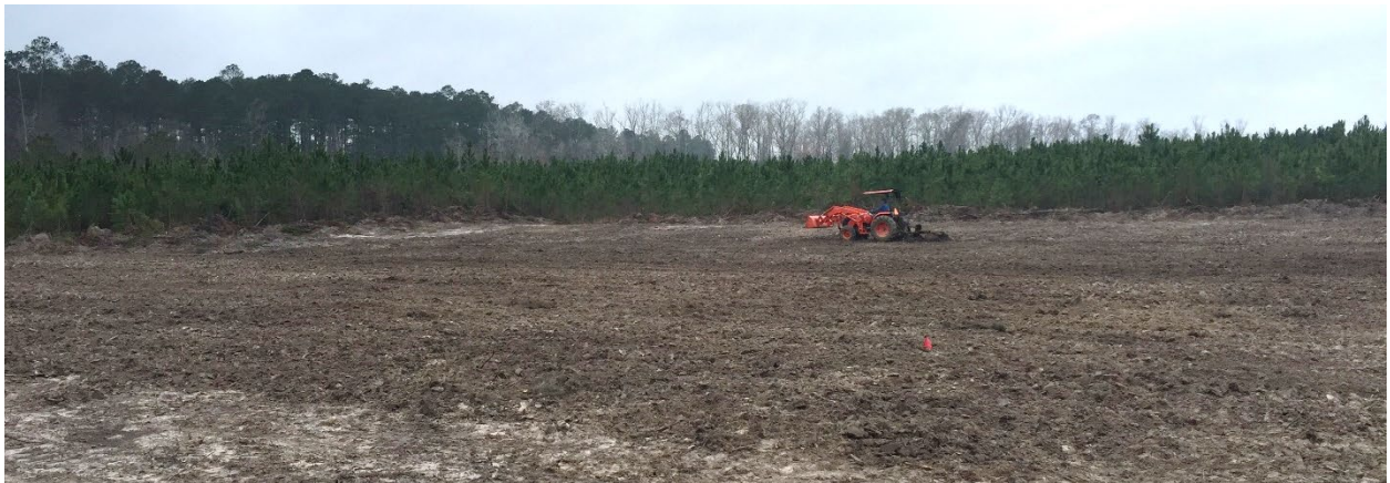
Figure 11. Initial site preparation.
