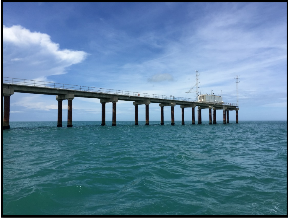
Figure 10. Photographs of the 1,840-foot-long FRF Pier
