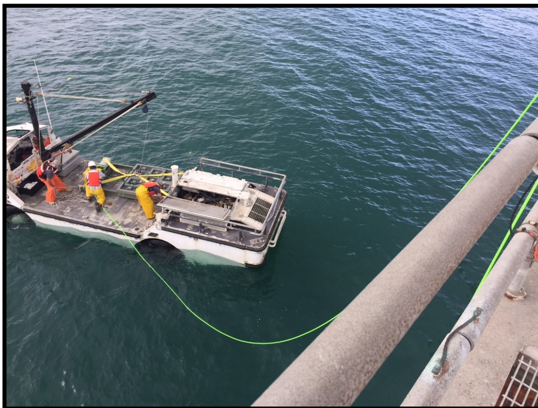
Figure 16. Connecting Pier-based Laptop to EM System by Lowering Cable from Pier
