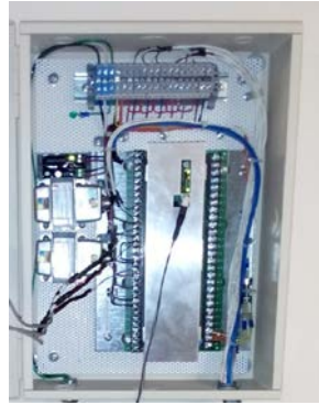
(b) Installed new BAS panel to accommodate additional signal communication
