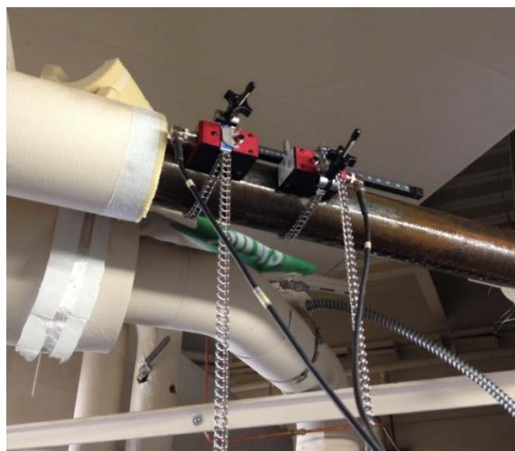
Figure 5.13. Temporary Ultrasonic Meter Installation on the Secondary Chilled Water Loop.
