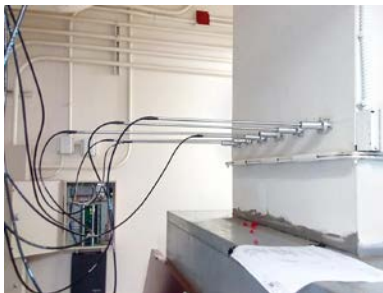
(c) Installed brackets with holding velocity probes
