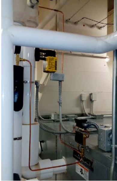
Figure 5.8. Permanent Water DP Installation for Virtual Valve Flow Meters.
