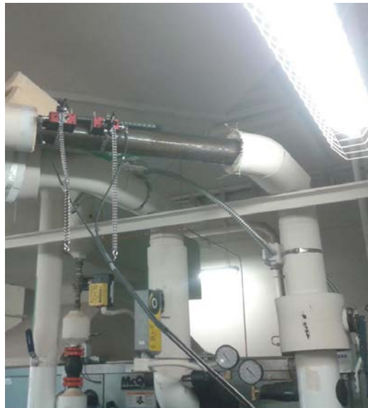
Installed ultrasonic meter
