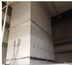
(a) Available holes for traverse measurements
