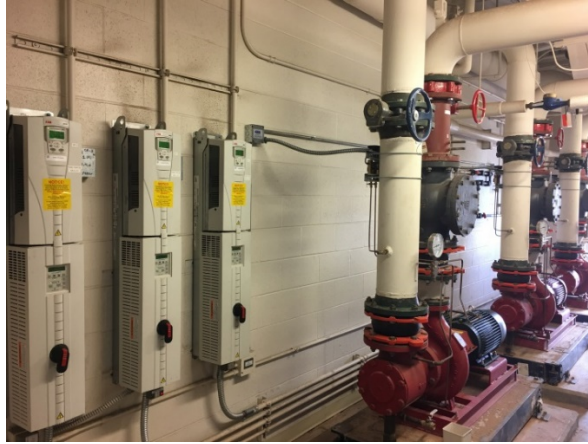
Figure 5.11. Permanent VFD Installation on Condensing Pumps.
