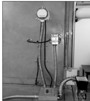
(a) Installed air differential pressure transducer
