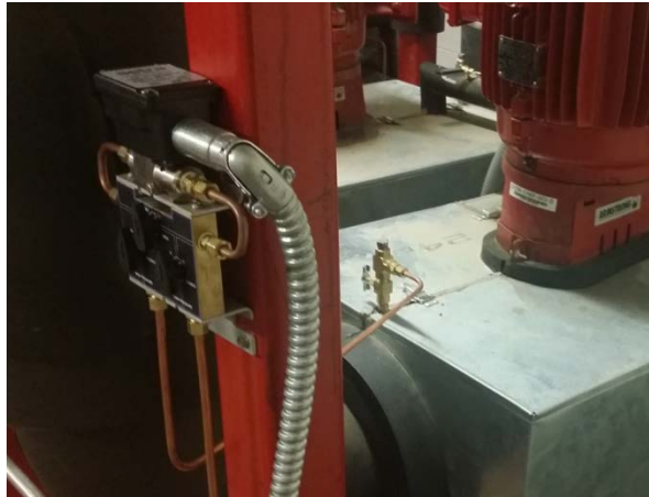
Figure 5.12. Permanent Differential Pressure Transducer Installation for Virtual Pump Flow Meters.
