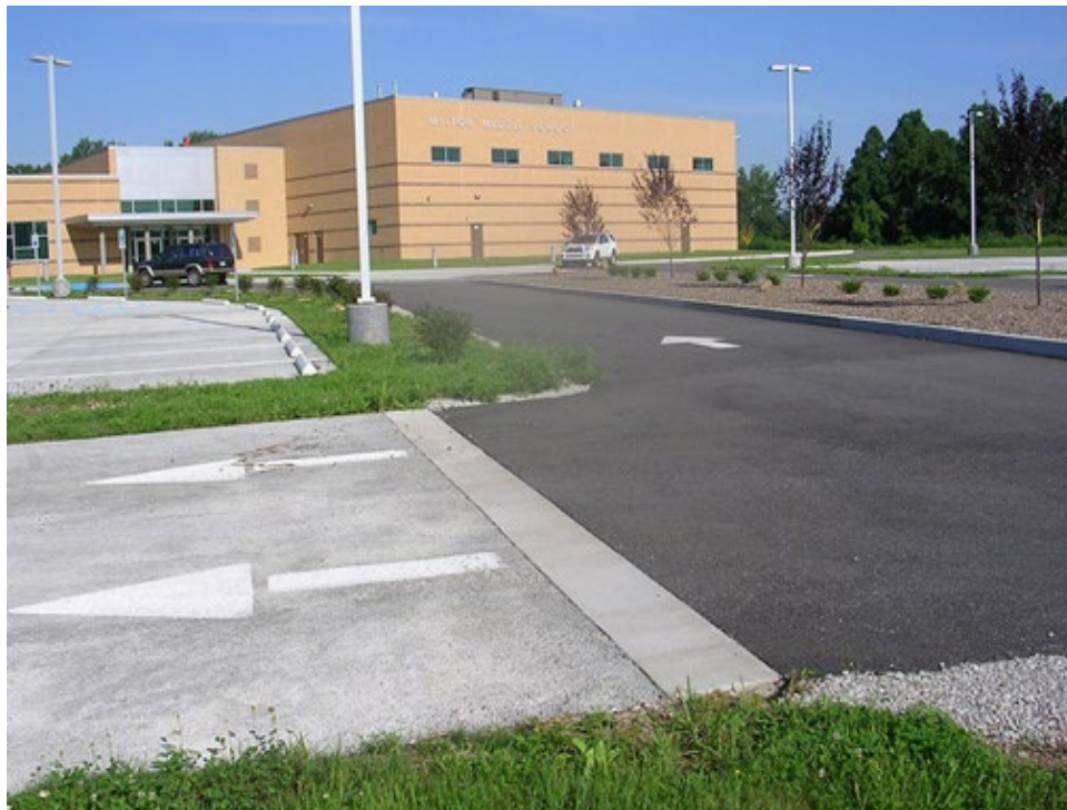
Figure 10. Permeable concrete (light gray) used throughout a parking lot. ( www.dep.wv.gov ).
