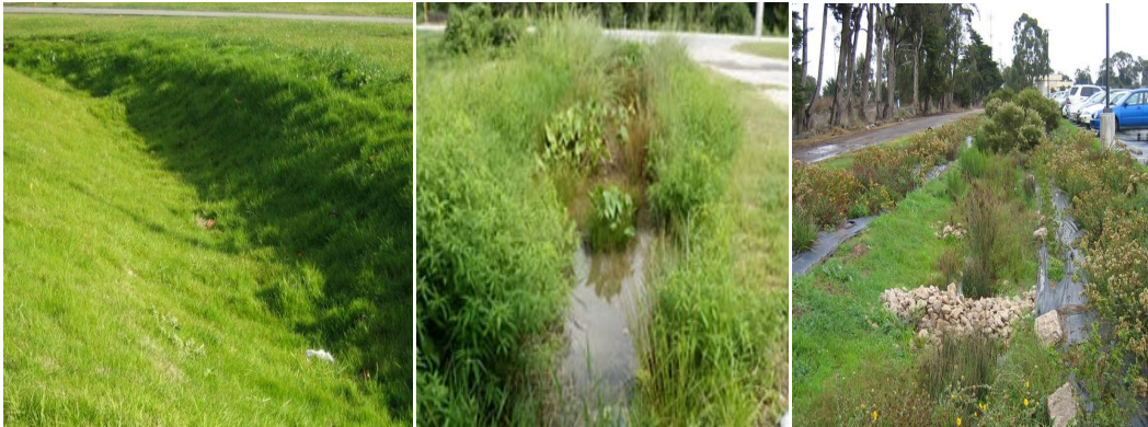
Figure 3. Three types of vegetated swales (from left): grass swale, wet swale, and bioswale.
