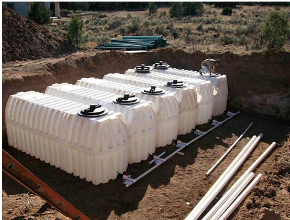
Figure 11.. Installation of a large underground cistern system ( www.theraincatcherinc.com ).
