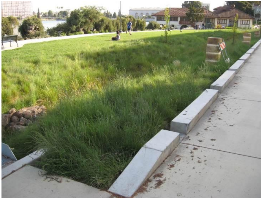
Figure 5. A vegetated swale featuring curb cuts and gravel filtration (waterunderground.files.wordpress.com).
