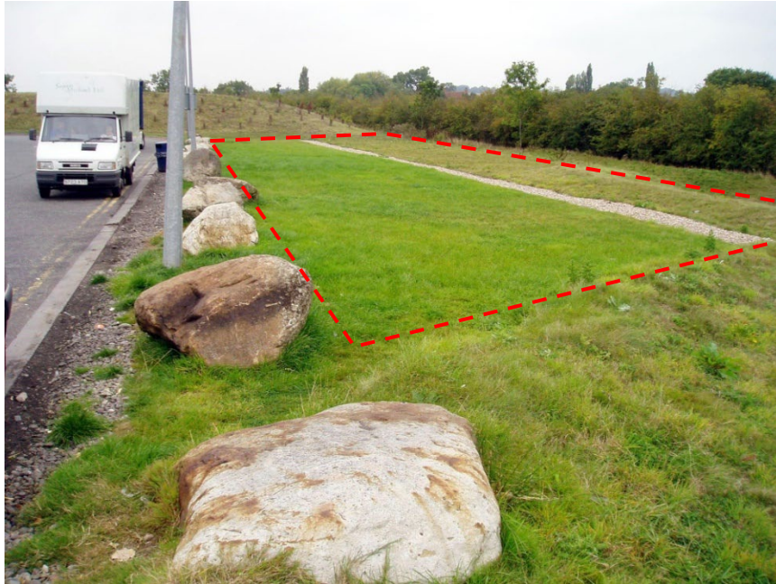
Figure 7. A vegetated filter strip with a gravel diverter ( www.susdrain.org ).
