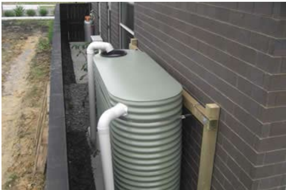
Figure 12. Small-scale, low-profile, above-ground rain collection system ( www.tanksalottx.com ).
