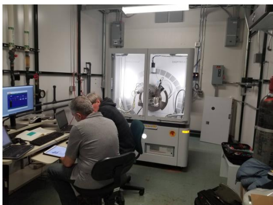
Figure 5(a). December 20 th 2018: PANalytical field engineers working on the installation of the XRD instrument
