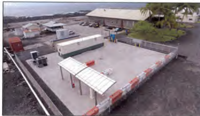
Figure 2.3.4: NELHA Hydrogen Production and Dispensing Station.
