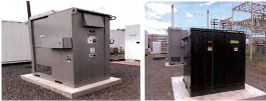
Figure 5.4. Installed load bank and step-up transformer.
