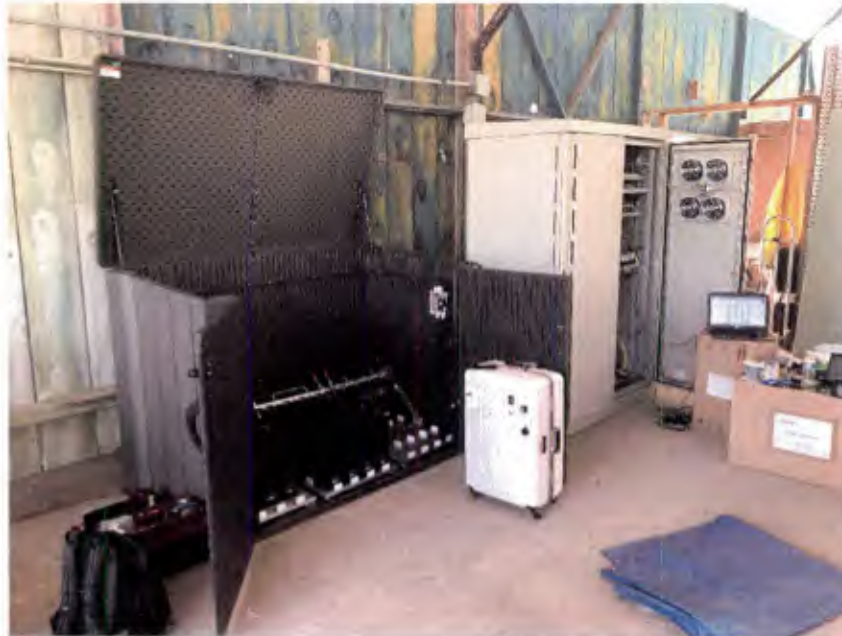
Figure 5.10. Swap battery charging station and portable BESS units.
