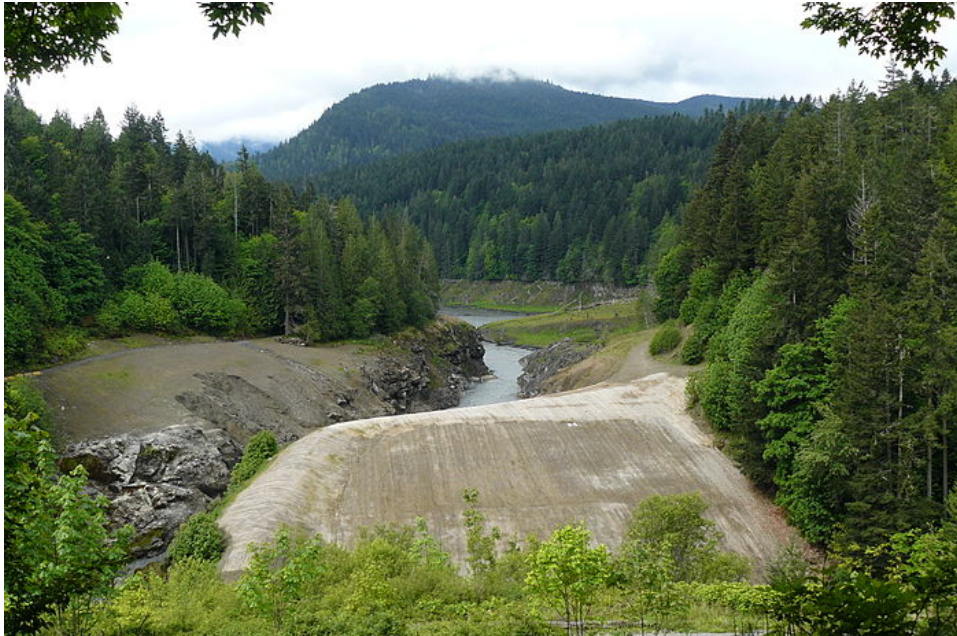
Figure 2. Elwha Dam after dam removal.
