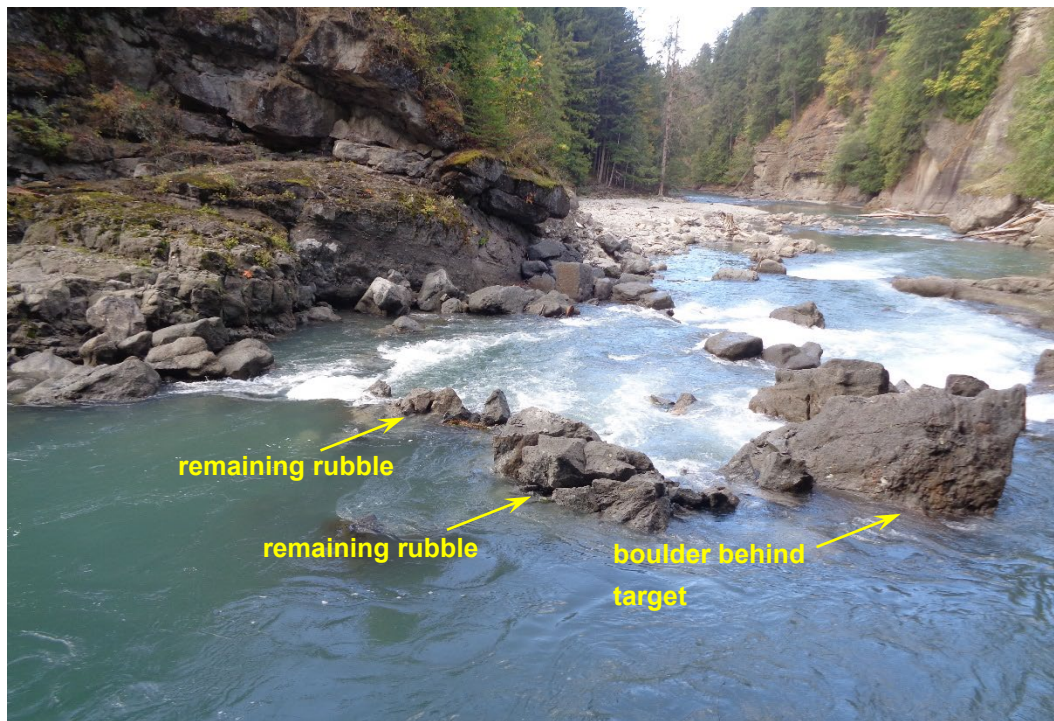
Figure 30. Post-demolition conditions at boulders downstream of ELD caisson.
