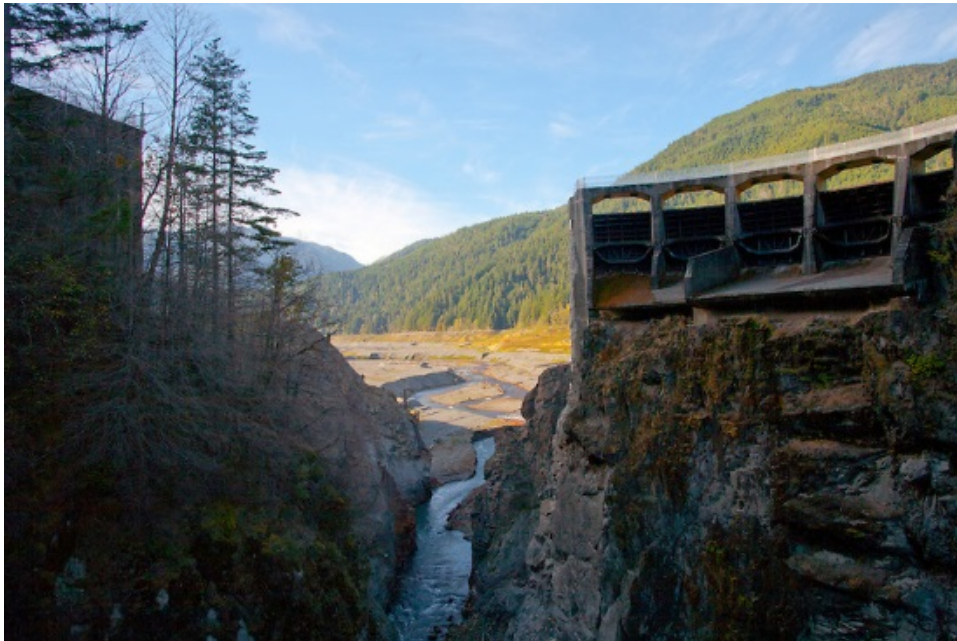
Figure 4. Glines Canyon dam after dam removal.
