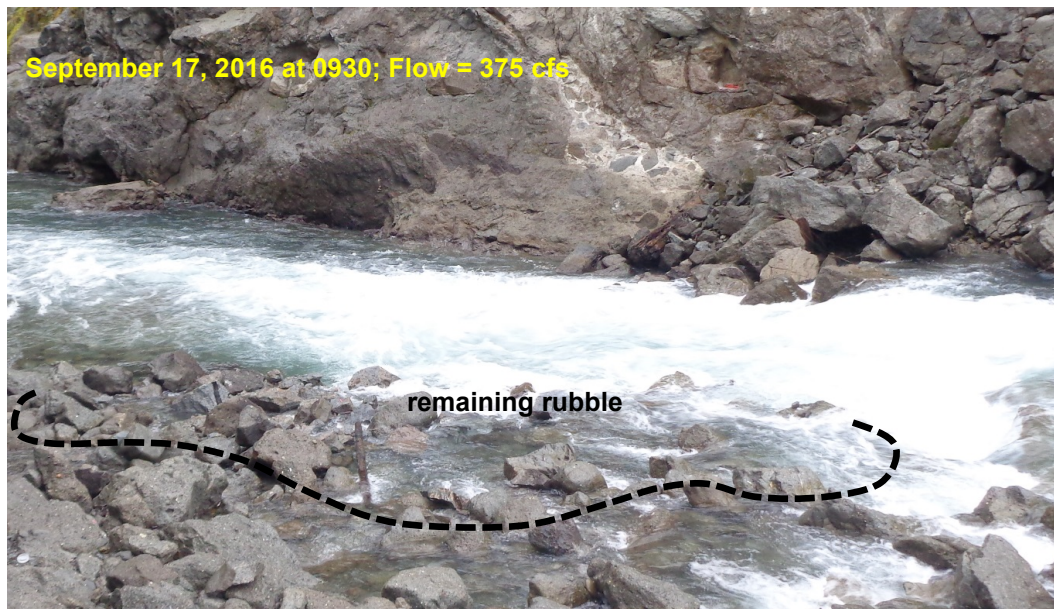
Figure 27. Rock shelf upstream of ELD site, post-demolition.
