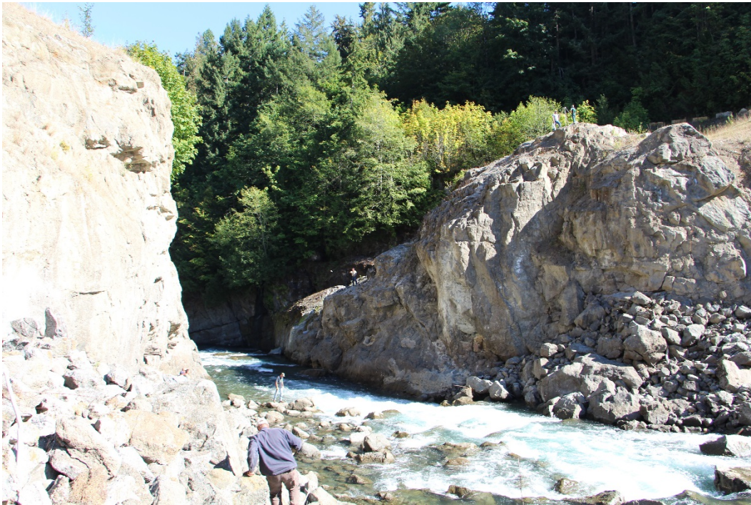
Figure 11. Downstream view at Elwha Dam site, September 2016.
