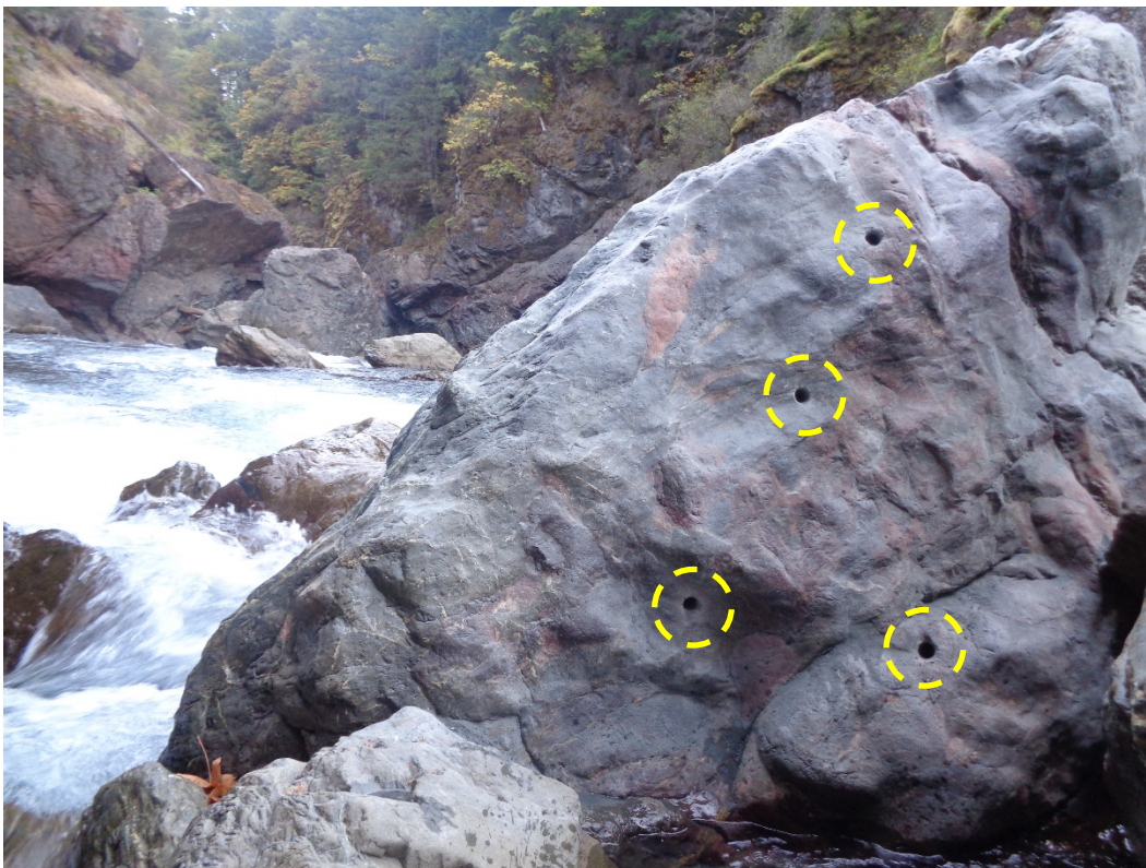
Figure 25. Typical drilled hole pattern (prior to charge placement).
