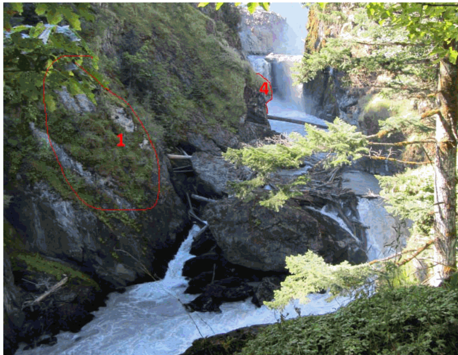
Figure 33. Obstruction downstream of GLI prior to dam demolition (courtesy of A. Ritchie).
