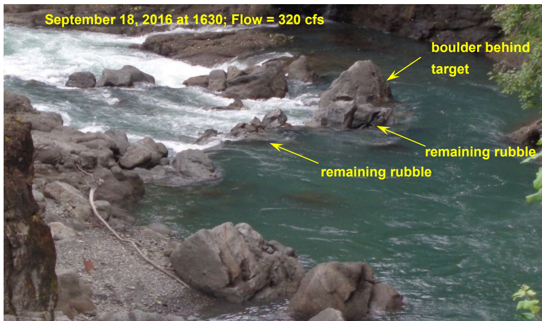
Figure 29. Boulders downstream of ELD caisson, post-demolition.
