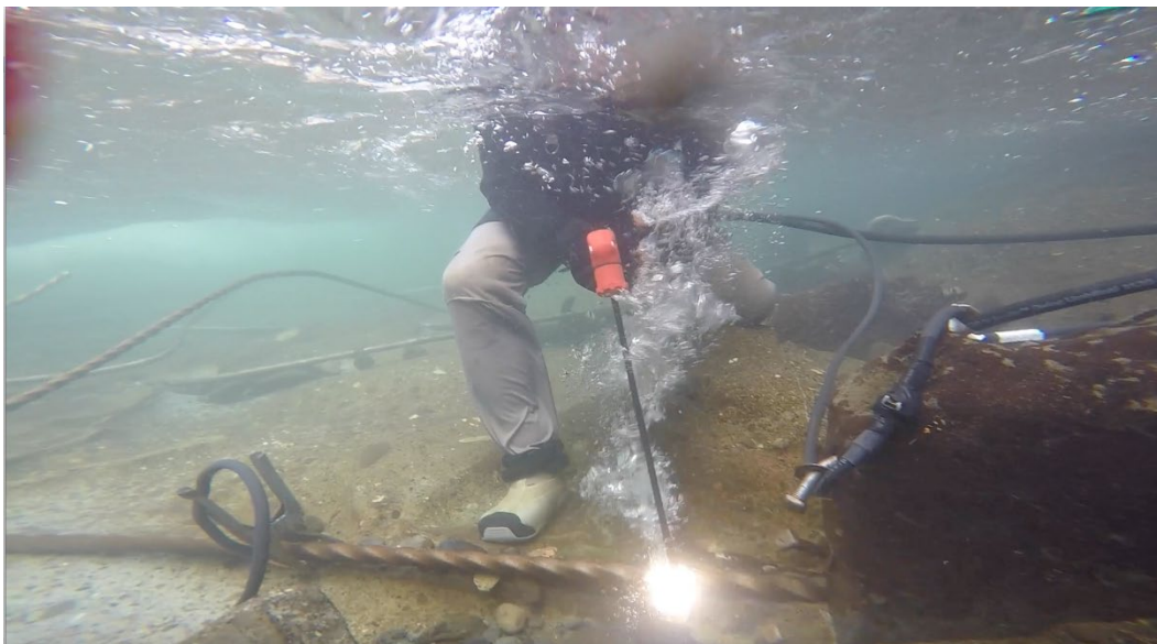
Figure 16. Underwater metal cutting.
