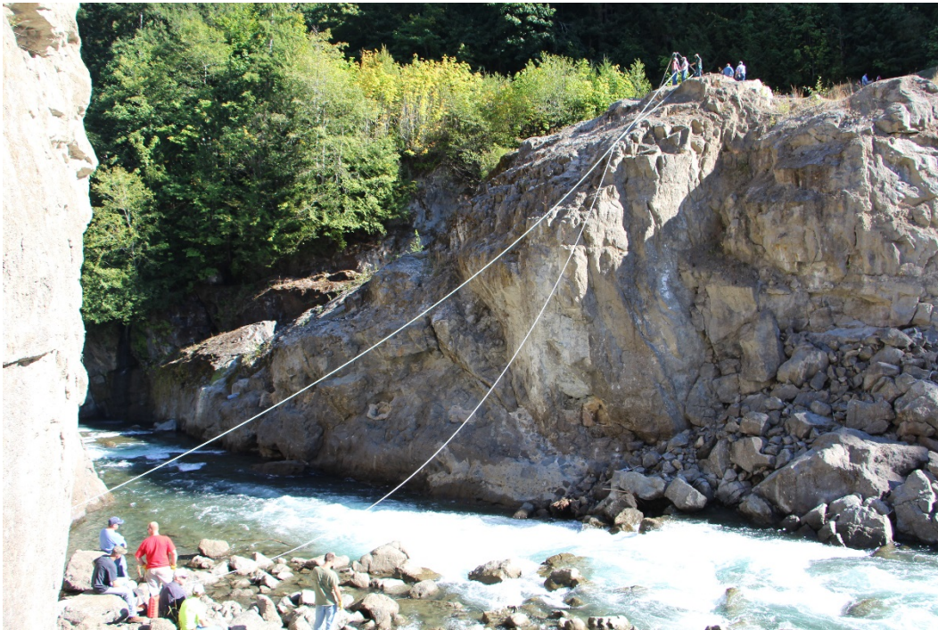
Figure 13. ELD cable system for equipment access.
