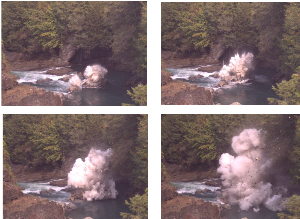
Figure 31. ELD boulder demolition from high-speed video.
