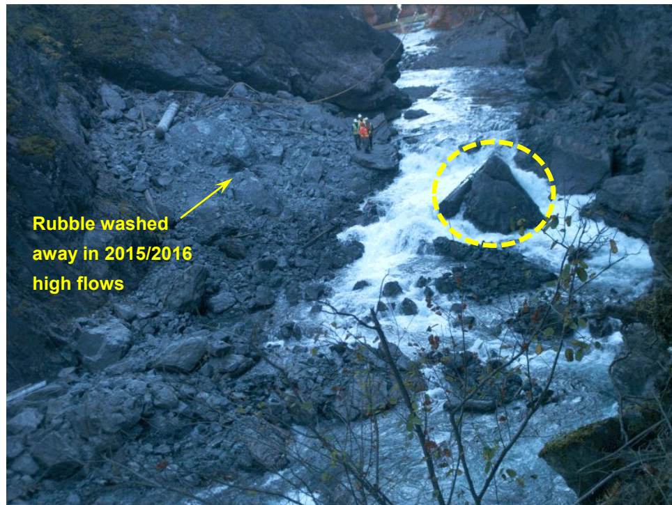
Figure 35. Channel downstream of GLI after 2015 blasting (courtesy of A. Ritchie).
