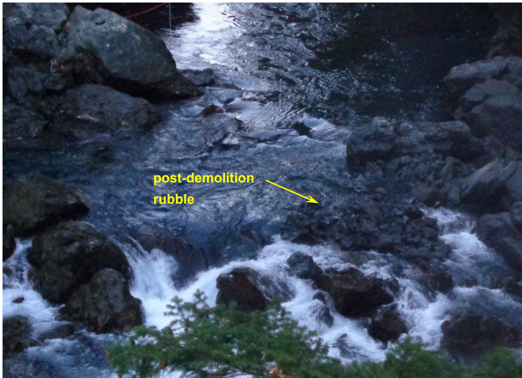
Figure 39. GLI left bank boulders after first two detonations.
