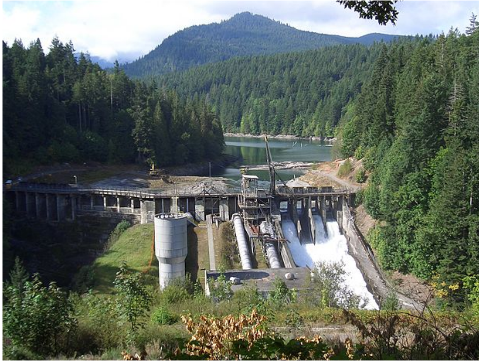
Figure 1. Elwha Dam before dam removal.
