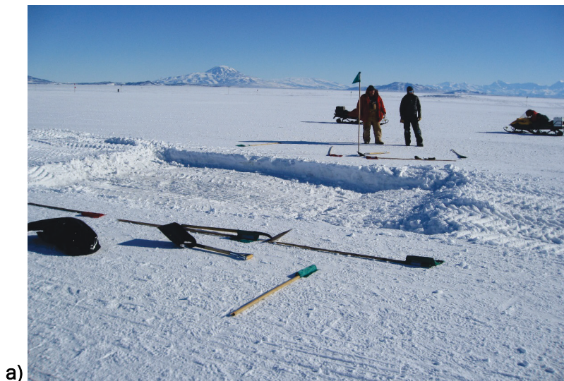
Figure 2. Patching of damaged area of compacted snow runway near McMurdo Station, Antarctica: a) excavated damaged area, b) fresh, tumbled snow being introduced to cavity, c) initial compaction of lower 8-inch layer, d) continued compaction of lower layer, and e) final compaction of upper 8-in. layer (which was placed and compacted in the same fashion as the lower layer).
