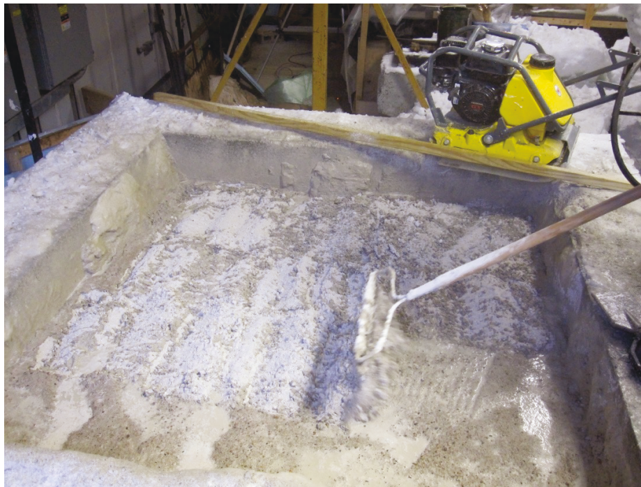
Figure 40. Layer of wetted dry flowable fill being stirred with rake when filling the base of the full scale crater.
