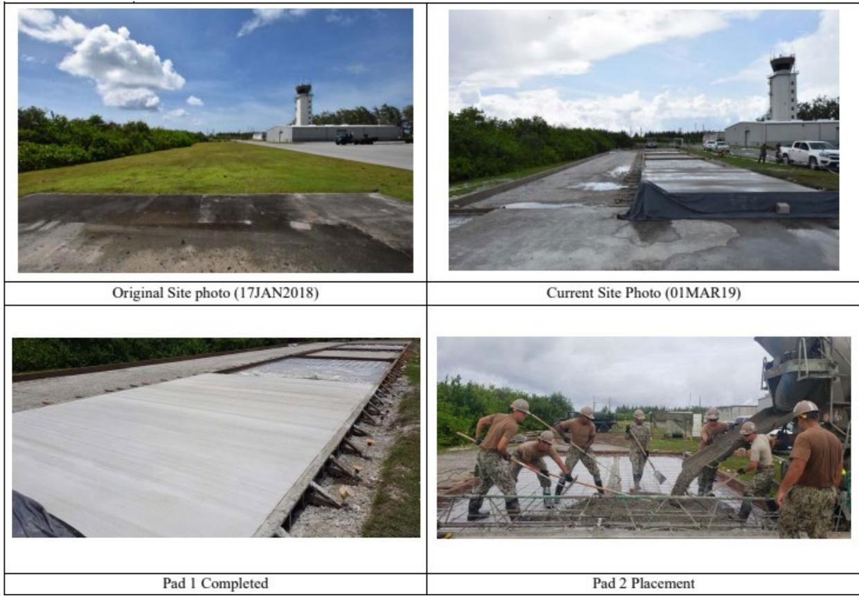
Figure 5 36ft x 205ft x 7in concrete pad construction (Source: Project Report from the 30<sup>th</sup> NCR)
