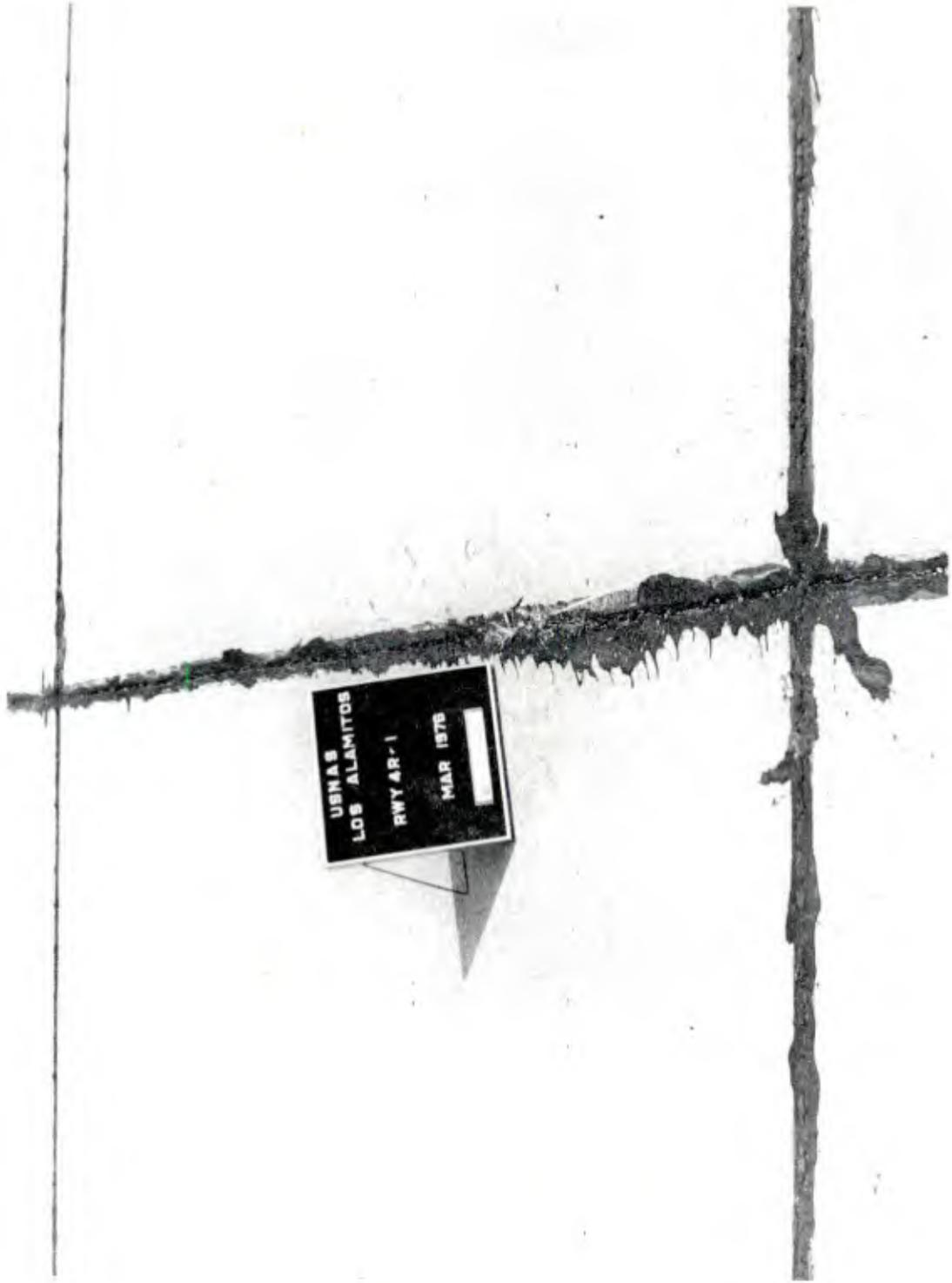
Figure 6. Vegetation in joints, Discrete Area R4R-1.
