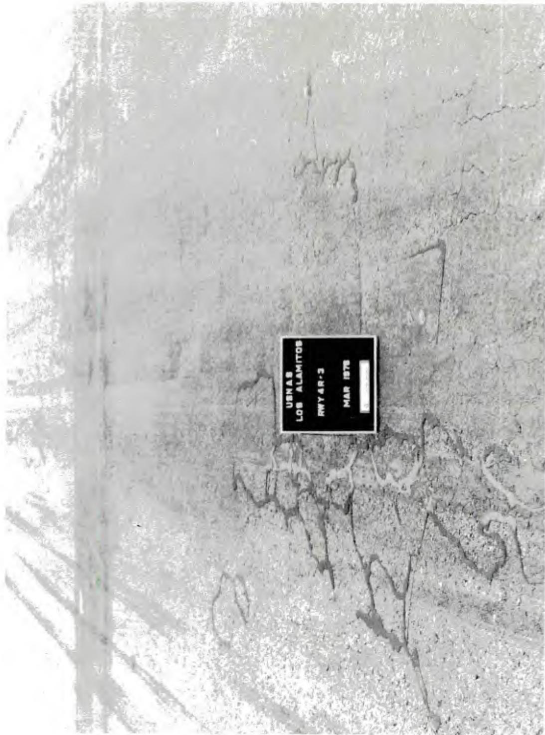
Figure 4. Pattern cracking, Discrete Area R4R-3.
