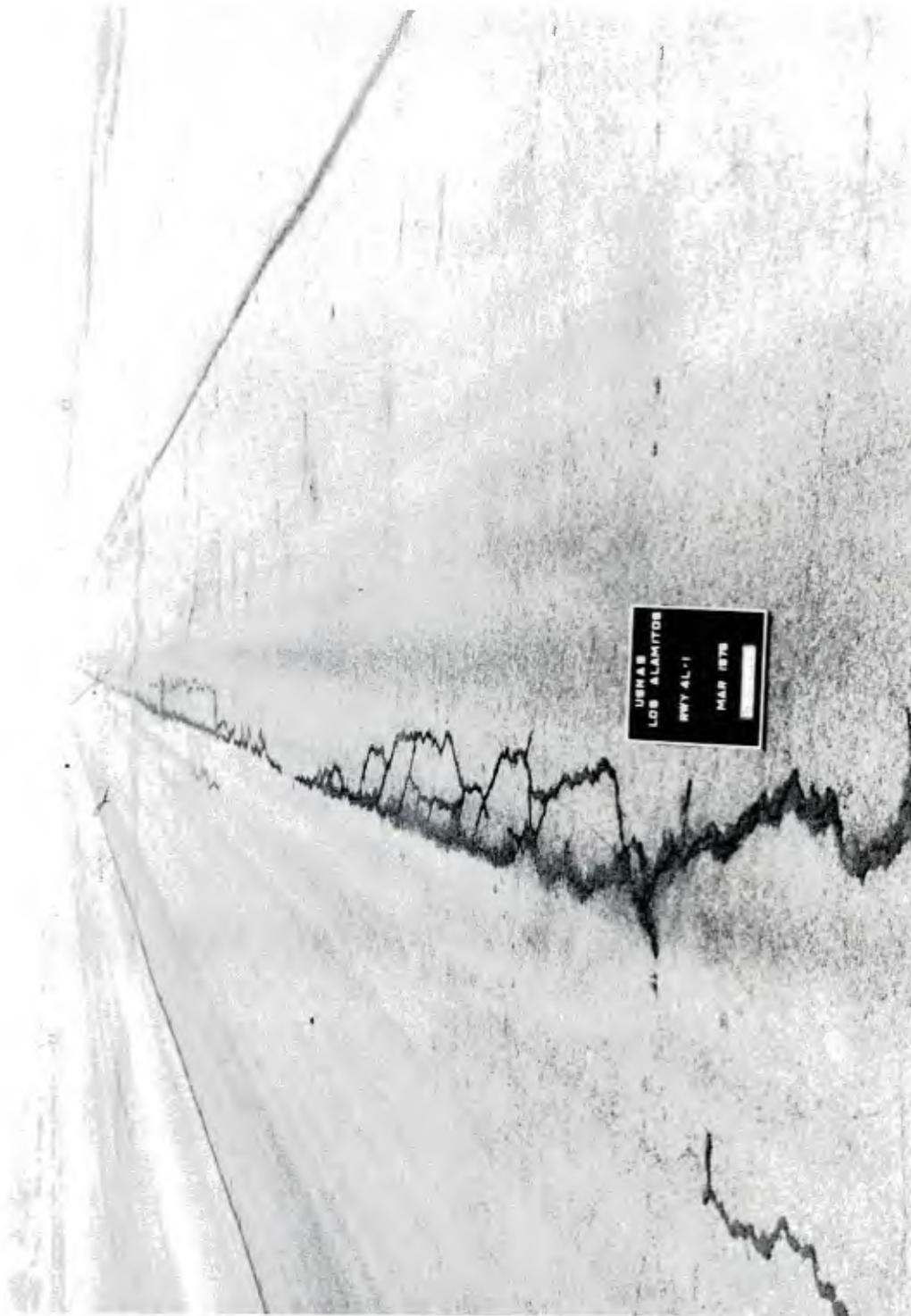
Figure 5. Longitudinal construction joint cracks, Discrete Area R4L-1.
