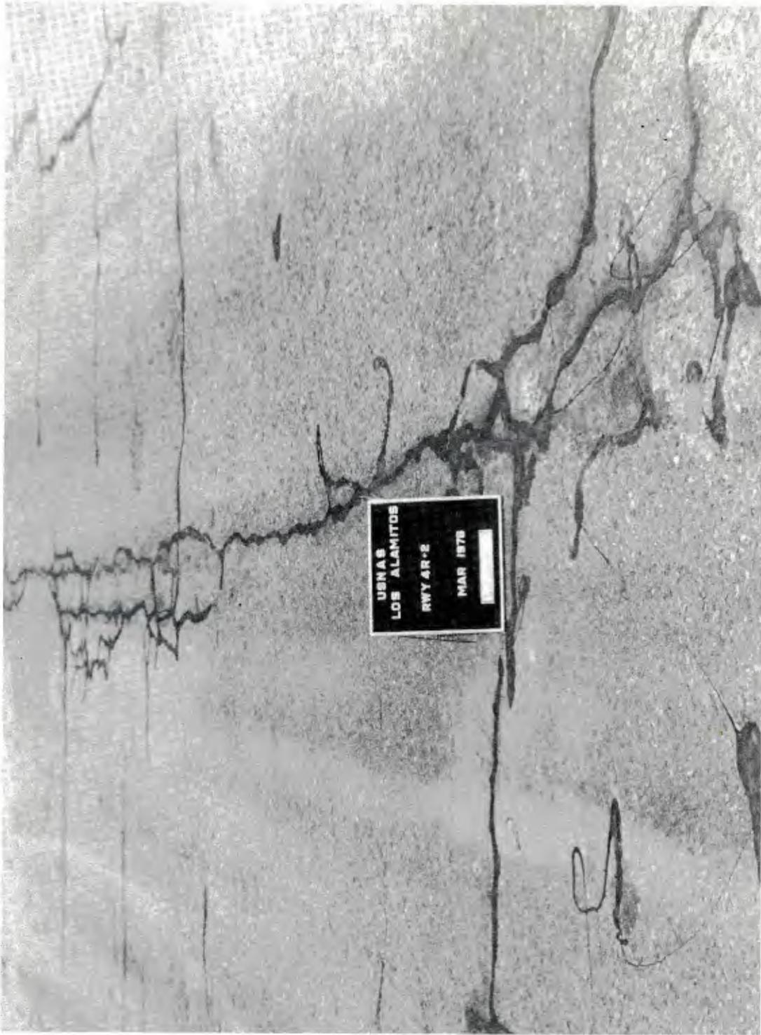
Figure 3. Typical partially sealed pattern cracking, Discrete Area R4R-2.
