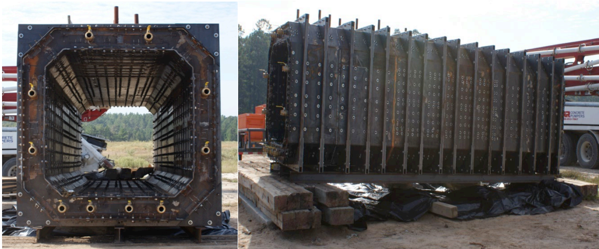
Figure 2. The 7 ksi column cross-section (left) and inclined steel formwork (right).
