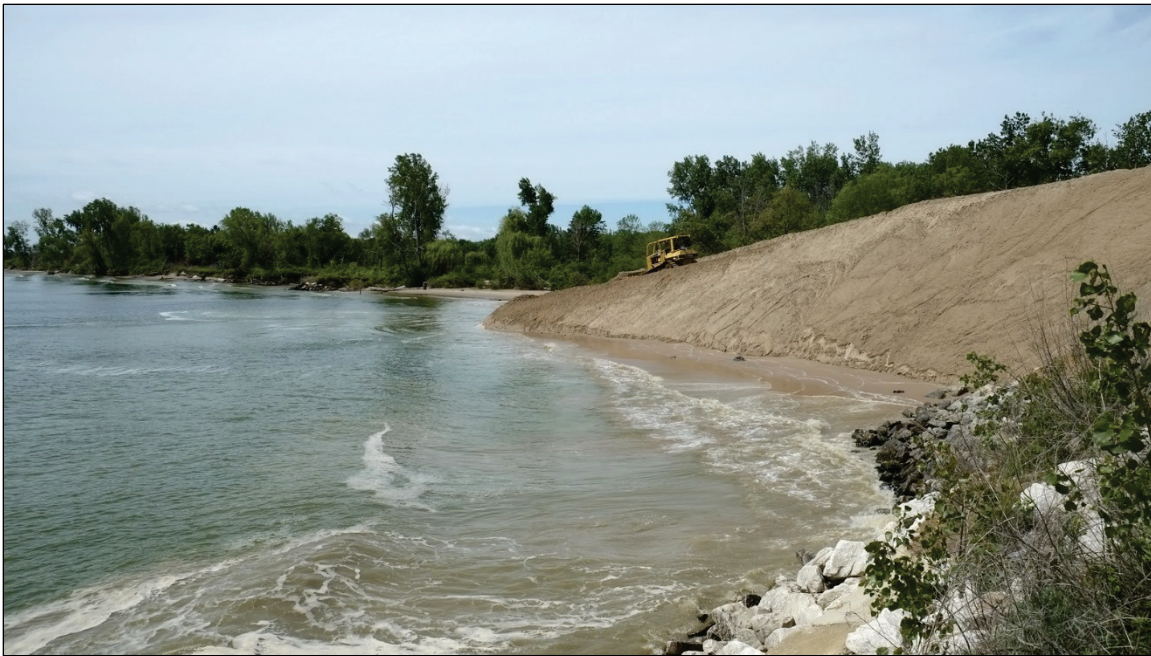
Figure 9. Sand dredged from the entrance channel at North Point Marina is piled south of the entrance and pushed into the lake. Photograph 17 June 2014.
