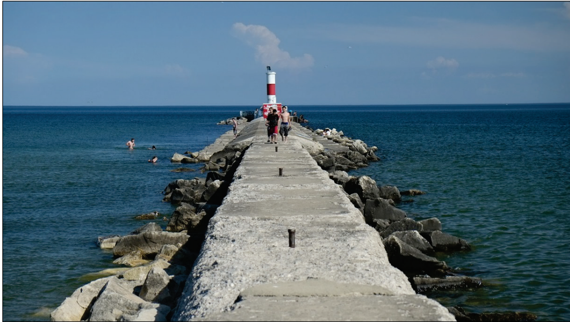
Figure 15. Waukegan Harbor north breakwater, view looking east. Shallow lakebed on the north side of the pier is demonstrated by the bathers standing in shallow water left of the structure. Photograph 17 June 2014.
