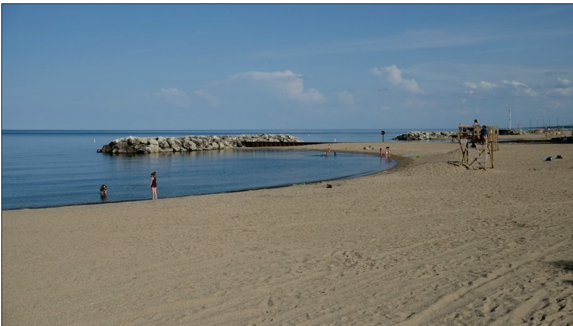
Figure 20. Forest Park Beach, City of Lake Forest. The shore-parallel breakwaters protect crescent-shaped beaches. Photograph 17 June 2014.
