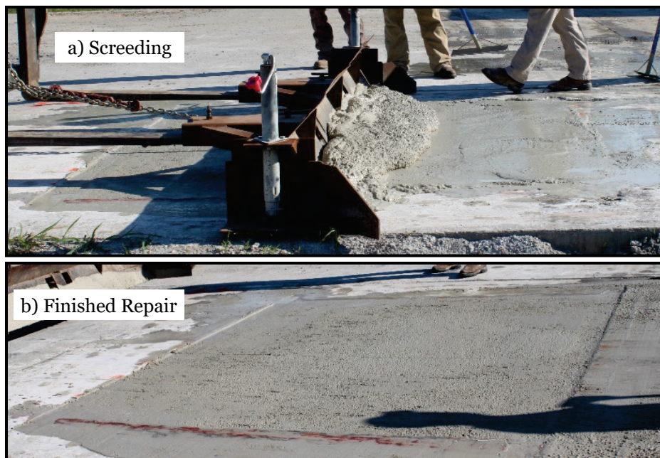
Figure 3.2. Small crater RSC repair with the SSO.
