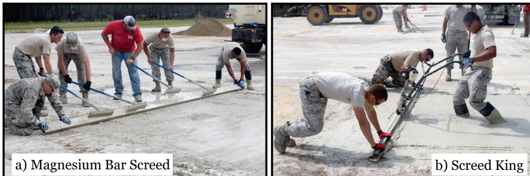
Figure 5.3. Bar screed and Screed King in use at the RADR demonstration.
