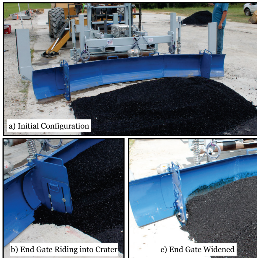
Figure 3.25. Small crater C1 AC repair with the ASTH.
