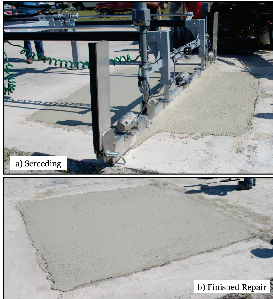
Figure 3.7. Small crater RSC repair with the ASHyd.
