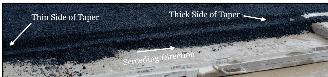
Figure 4.10. Tapered AC edge due to upward angle of end gate nose.
