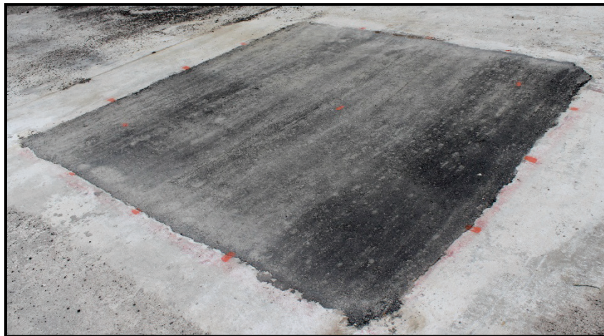
Figure 3.14. Completed small crater AC repair with the SSO.
