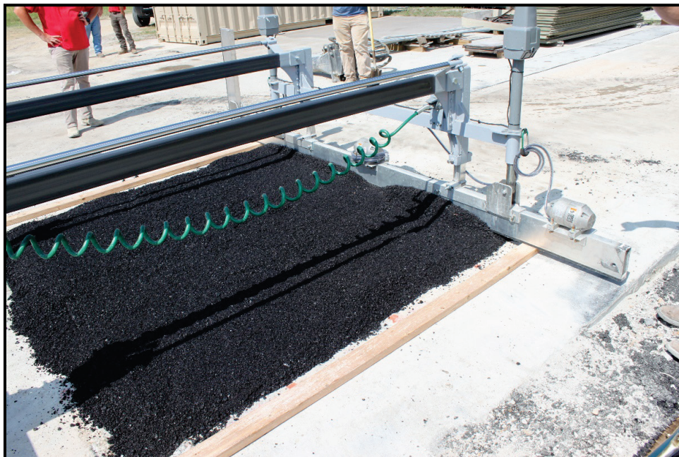
Figure 3.22. Small crater AC repair with the ASHyd.
