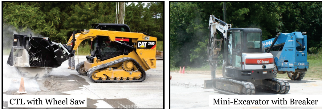
Figure 2.3. Producing test craters.
