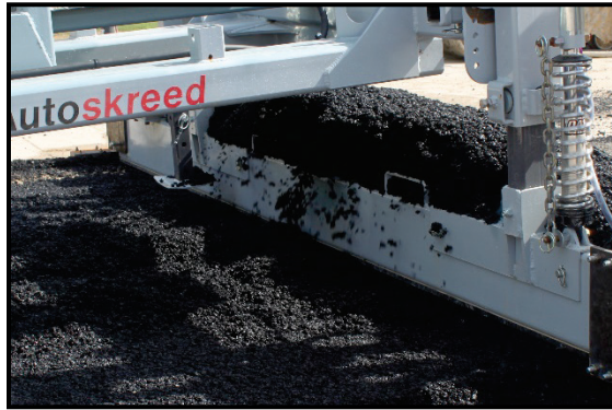
Figure 4.8. AC overtopping ASTH-Mod screed board.
