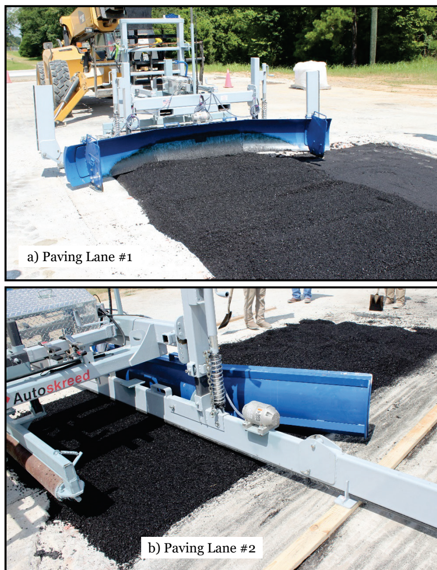
Figure 3.27. Large crater AC repair with the ASTH.
