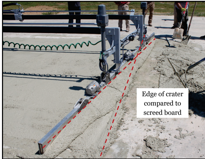
Figure 3.8. Angled ASHyd screed board.
