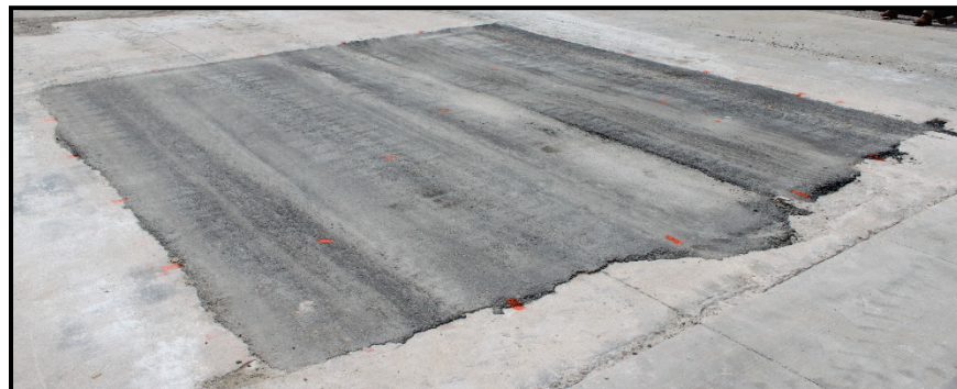
Figure 3.18. Completed large crater AC repair with the SSO.
