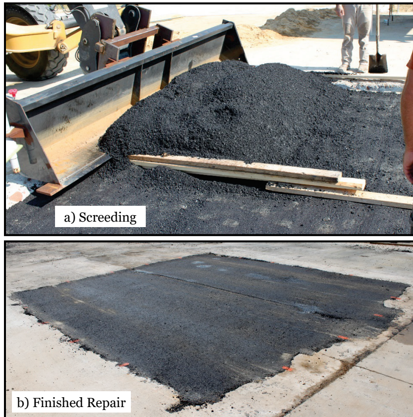
Figure 3.21. Large crater AC repair with the BSO.
