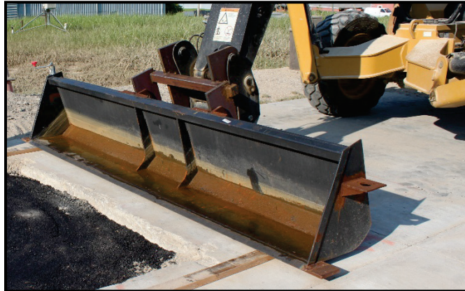
Figure 2.12. Bucket Strike Off.
