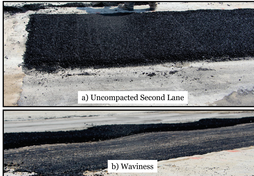
Figure 3.17. Second paving lane of large SSO repair.
