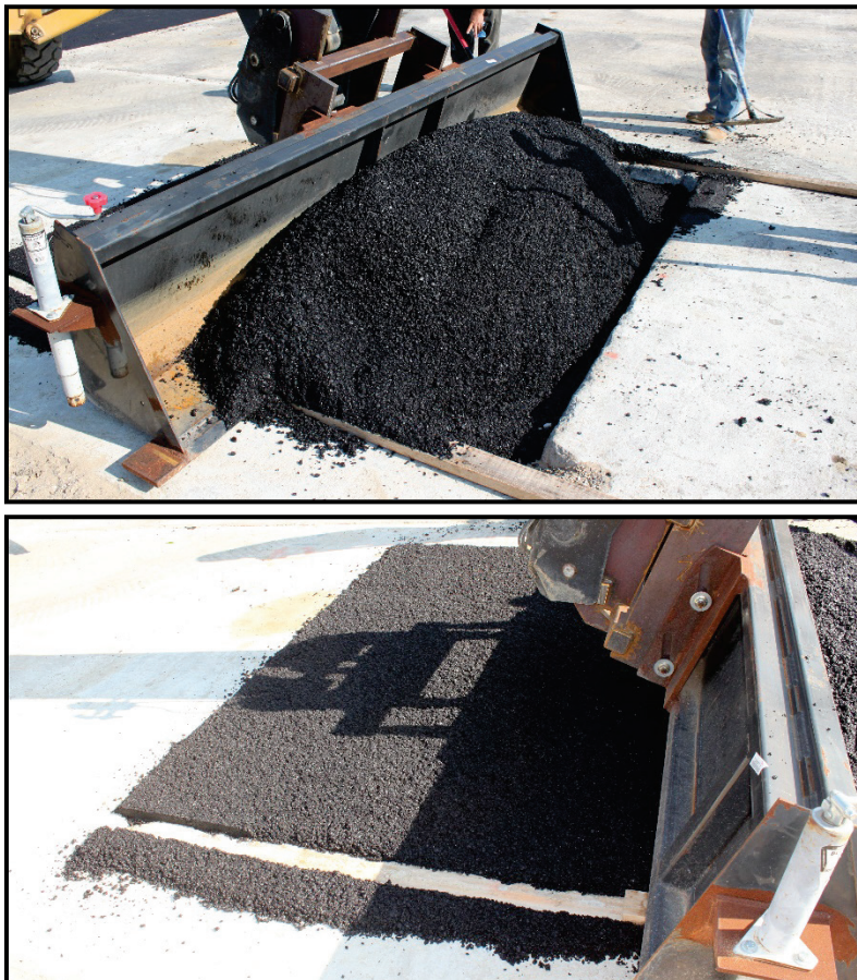
Figure 3.19. Screeding small crater AC repair with the BSO.
