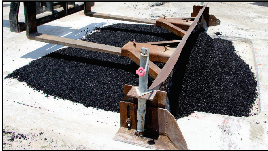
Figure 3.12. Screeding small crater AC repair with the SSO.
