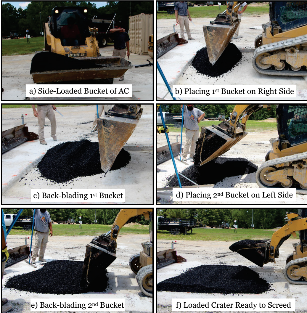
Figure 2.19. Photos of loading AC and performing pre-strike-off.
