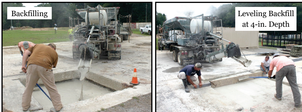
Figure 2.4. Placing FF-CTS-2 backfill in test craters.
