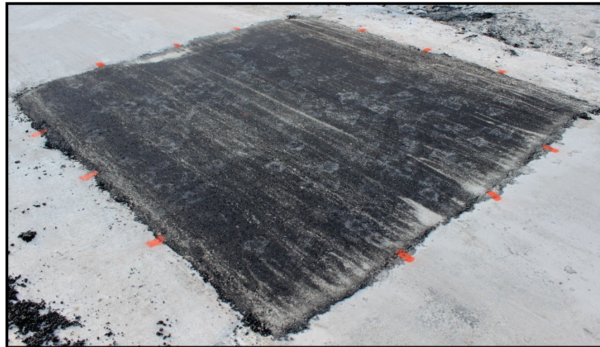
Figure 3.24. Completed small crater AC repair with the ASHyd.
