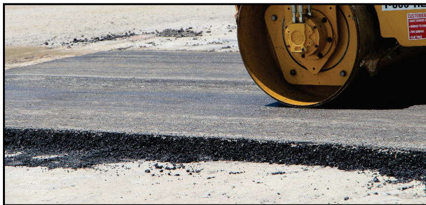
Figure 3.16. Inside face of first paving lane of large SSO repair.
