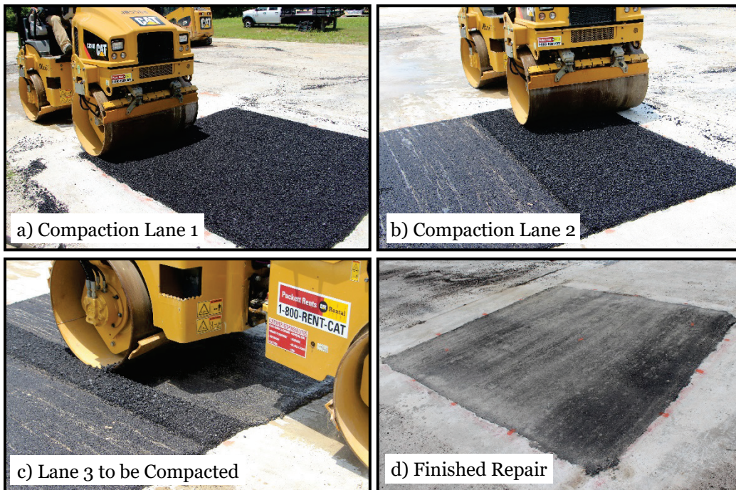
Figure 2.21. Photos of AC compaction with CAT CB24B.
