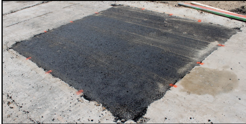
Figure 3.20. Completed small crater AC repair with the BSO.
