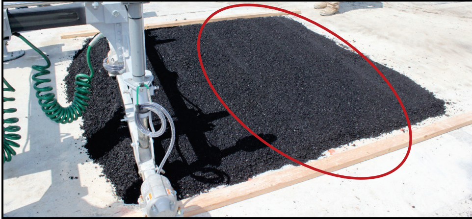
Figure 3.23. Waviness in screeded surface of ASHyd small crater AC repair.
