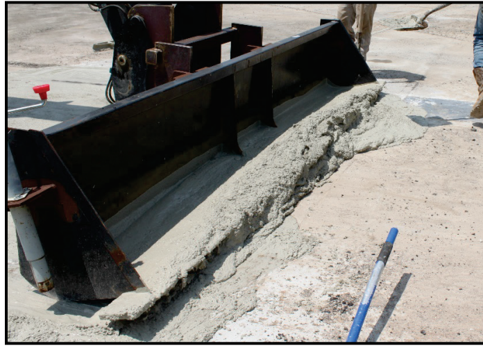
Figure 3.5. Excess RSC retained in BSO bucket requiring more cleaning.
