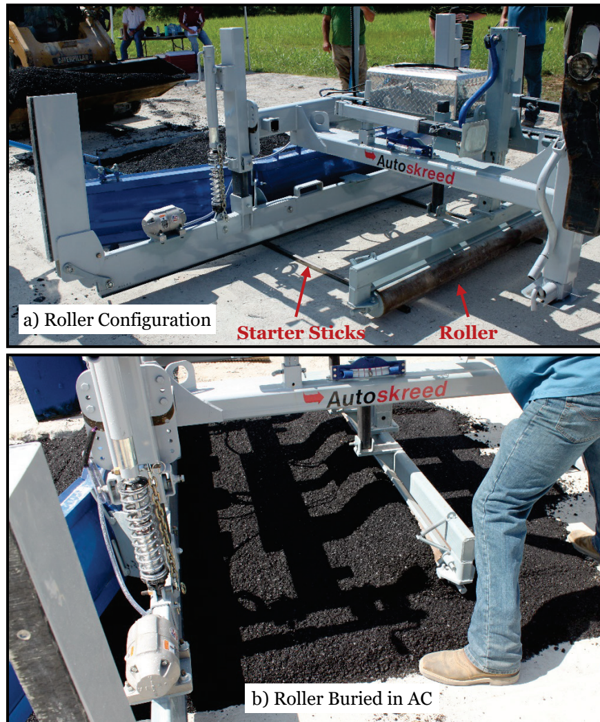
Figure 3.26. Small crater C2 AC repair with the ASTH.
