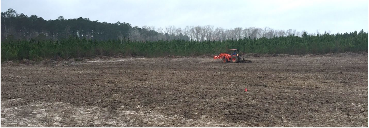
Figure 6. Initial site preparation.
