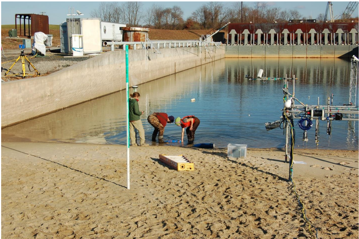
Figure 5. Picture showing the LWE facility looking offshore.
