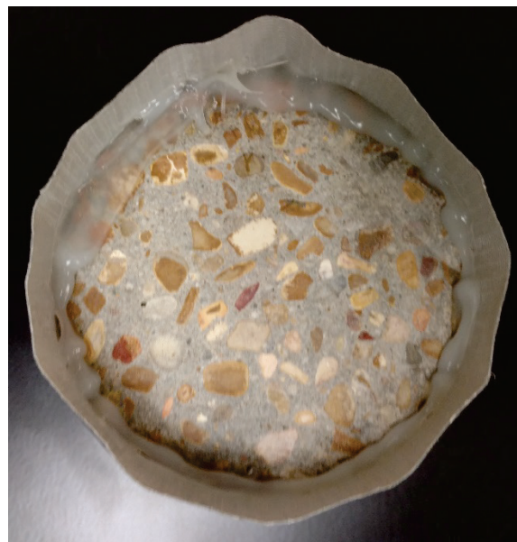
Figure 21. Exposed concrete surface.
